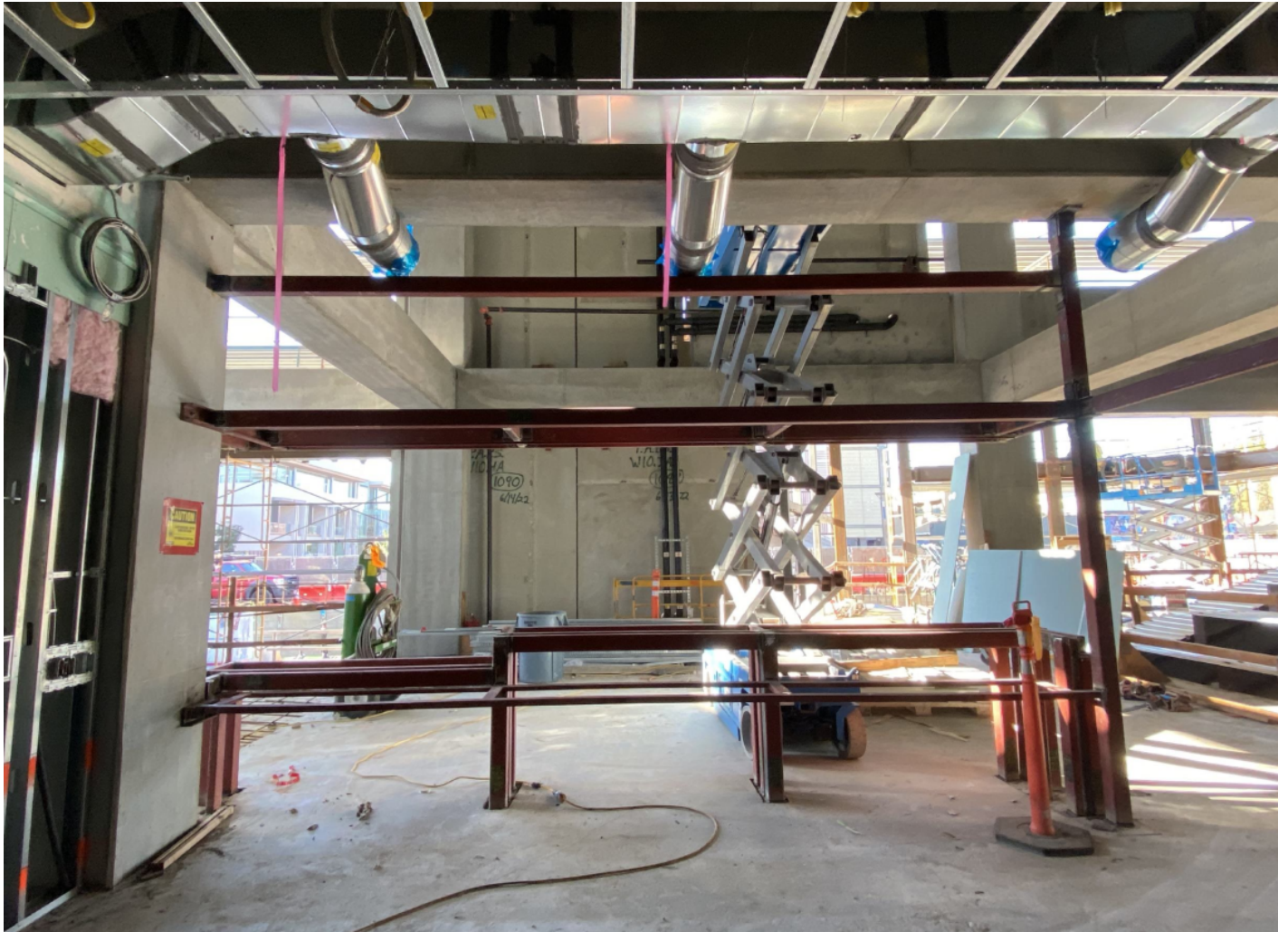
Public counter steel at lobby.
