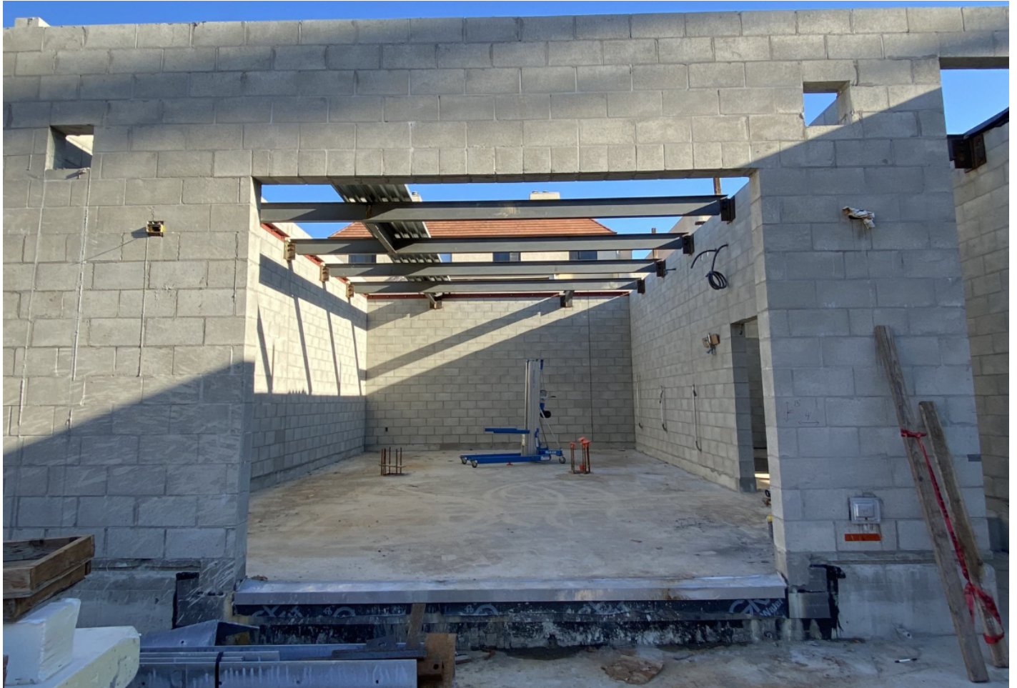
Utility Room installation progress photo.
