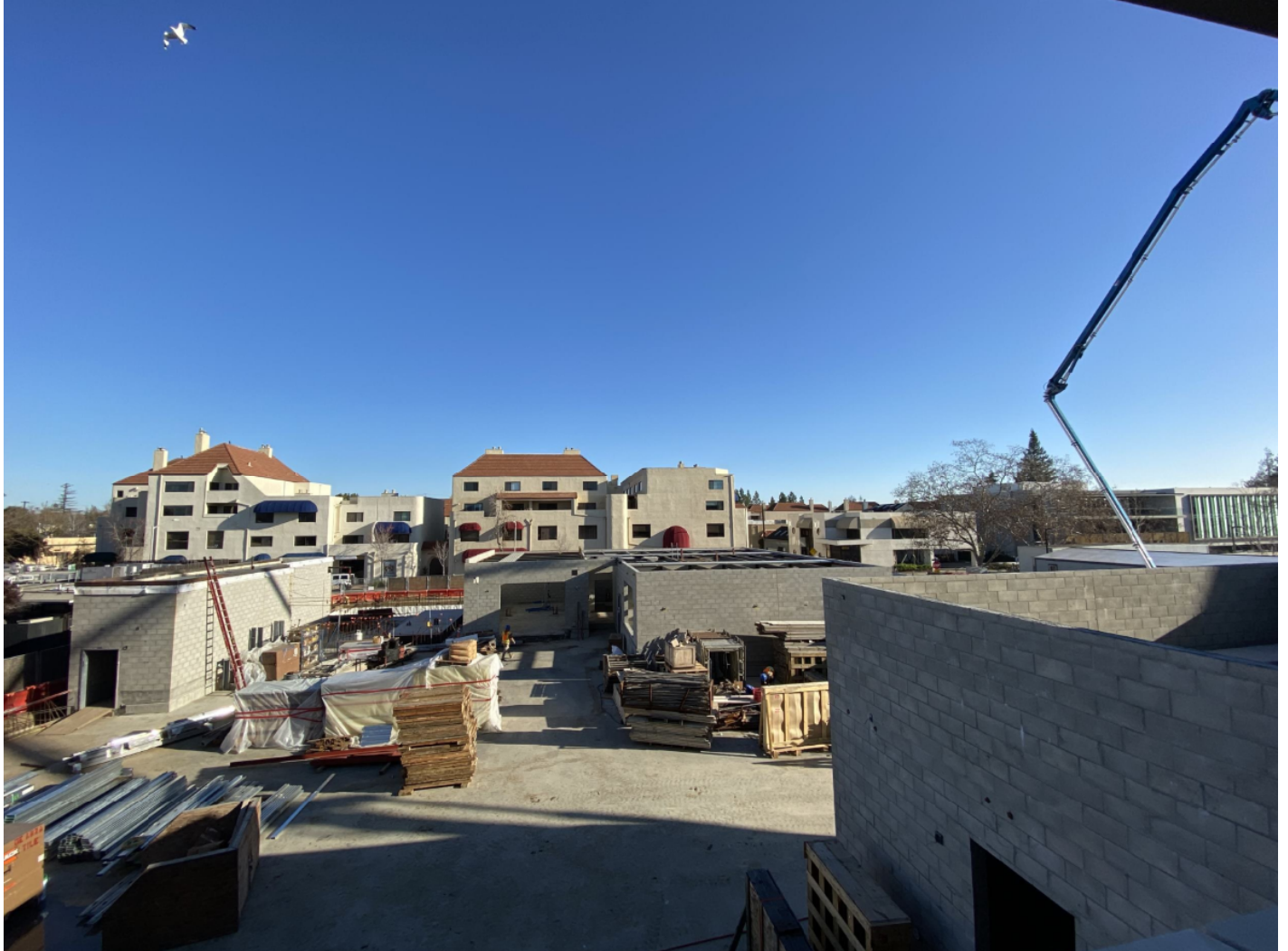
View of utility yard from Level 2.
