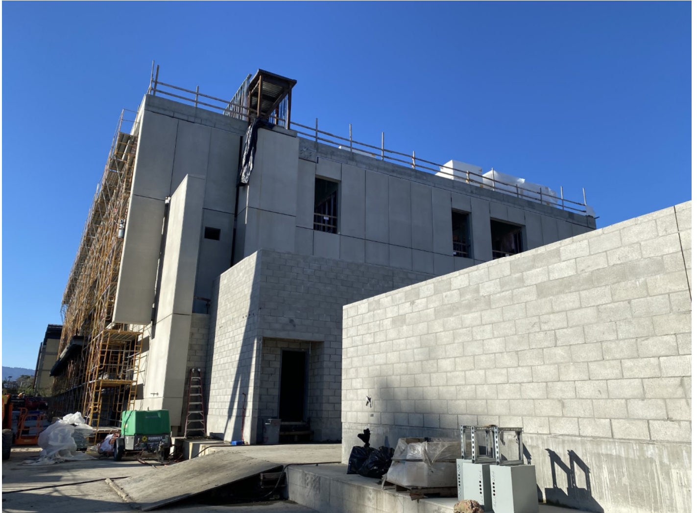
View of building from South East elevation.
