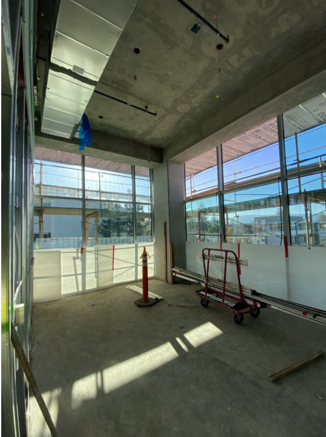
Level 3 Curtainwall completion.
