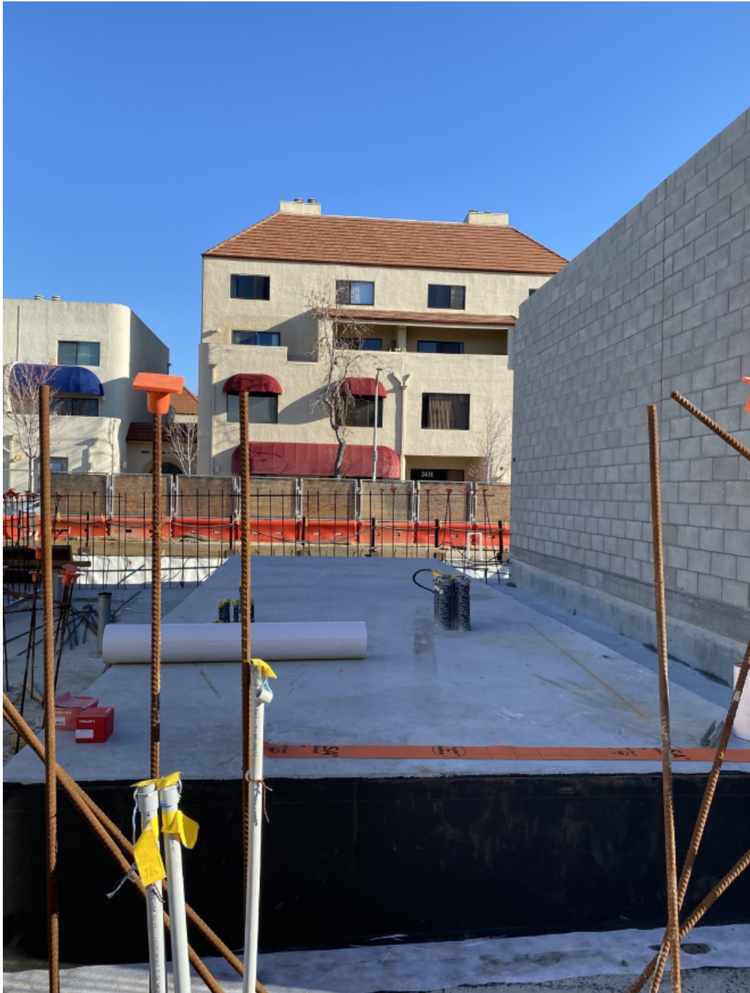
Generator pad waterproofing.
