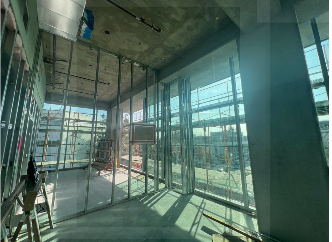
Level 3 Window Installation.
