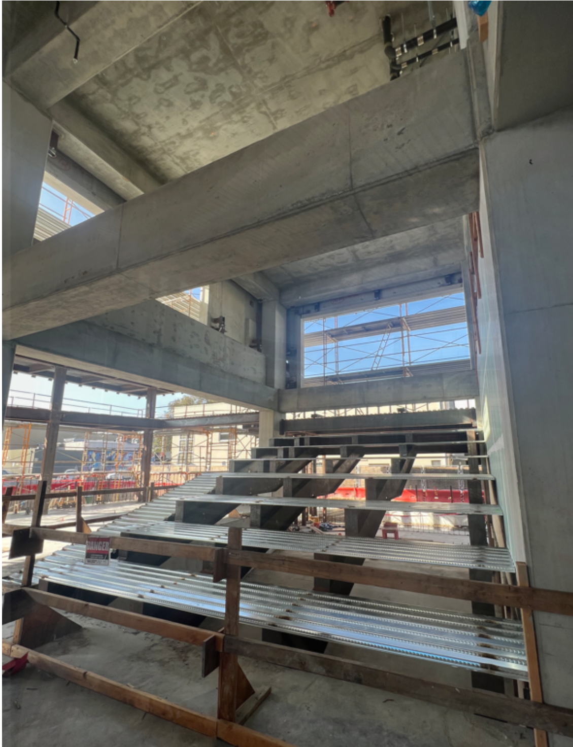
View of stair stringer near Multi-Purpose Room.
