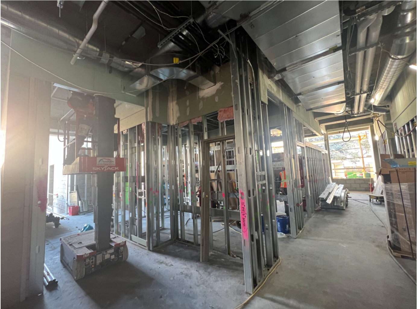
Interior Framing Level 1.
