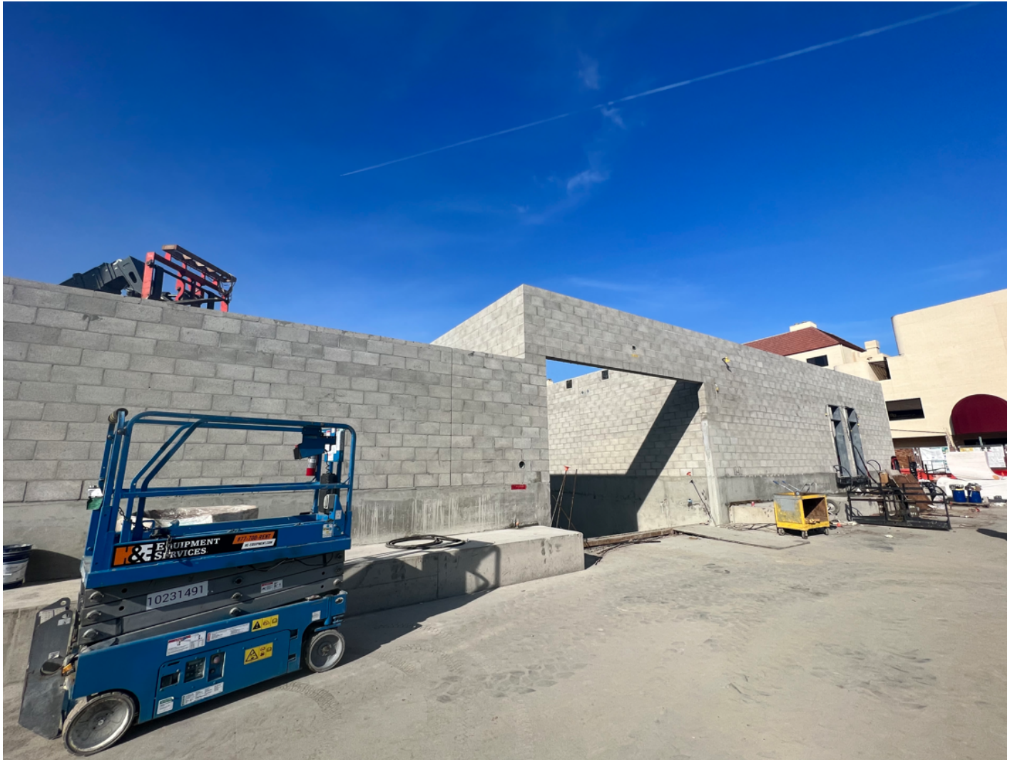
CMU Wall at Utility Yard.
