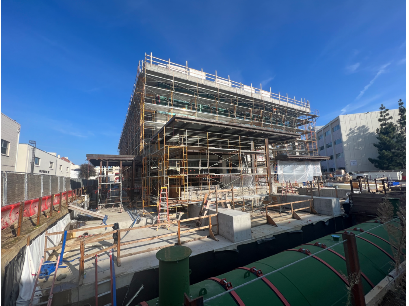
View from North West elevation.
