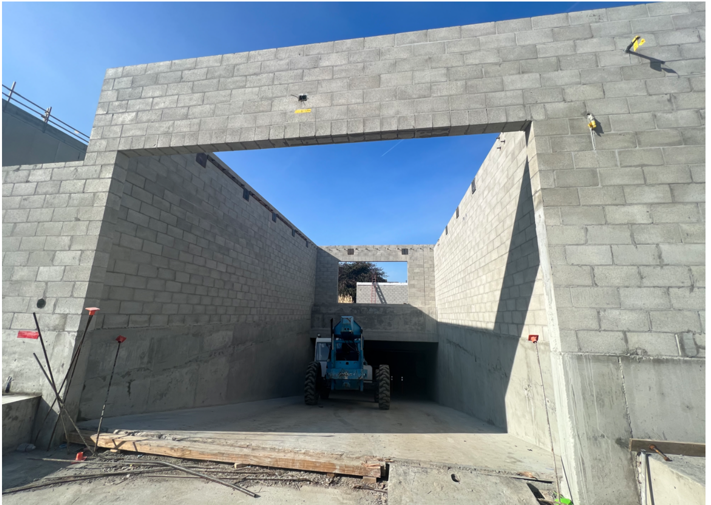
CMU Wall at Utility Yard.
