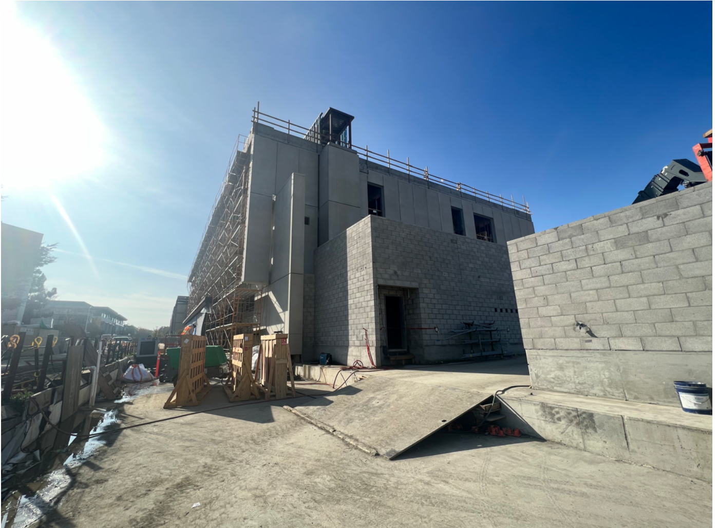
View from South elevation capturing the CMU Walls.
