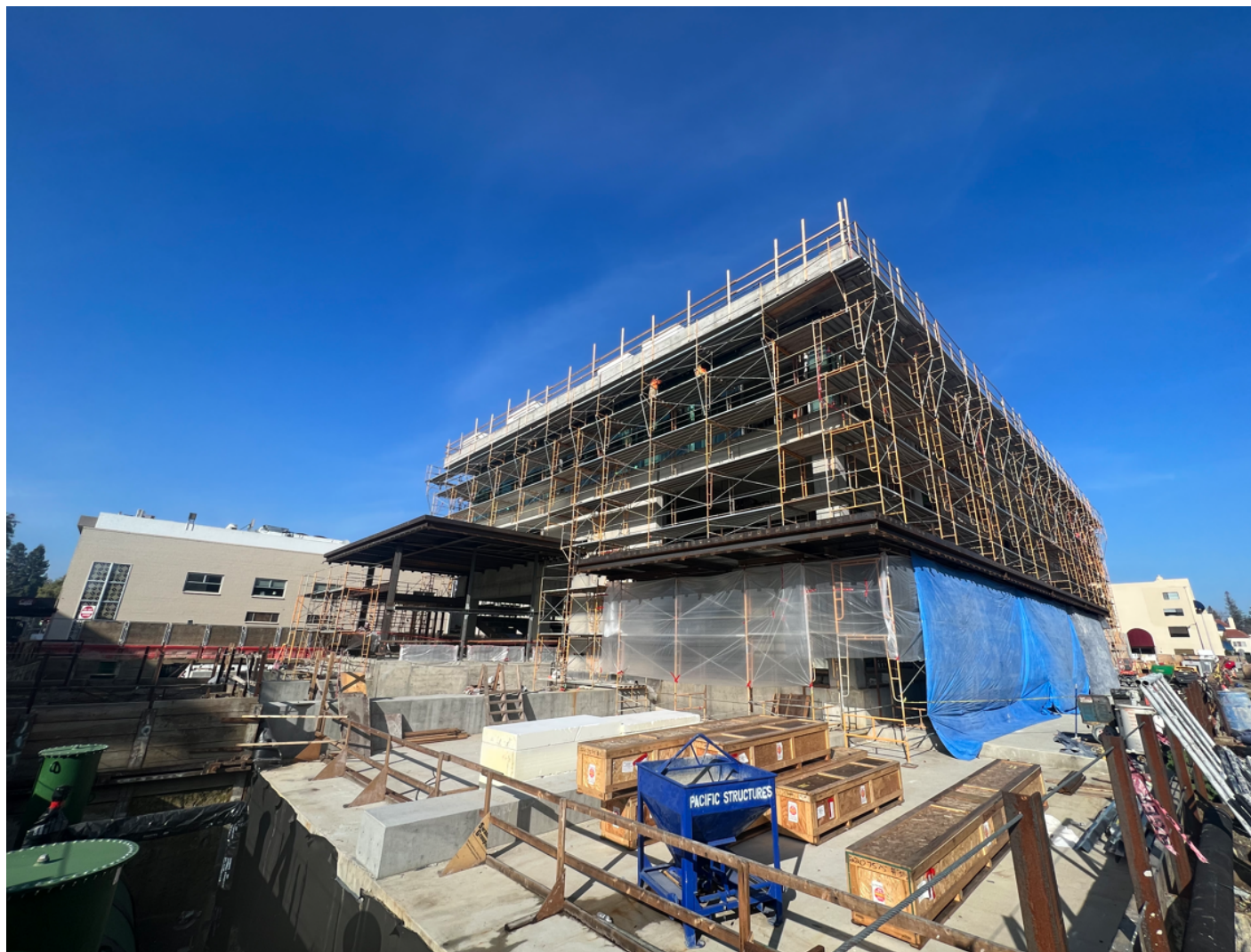
View from South West elevation.
