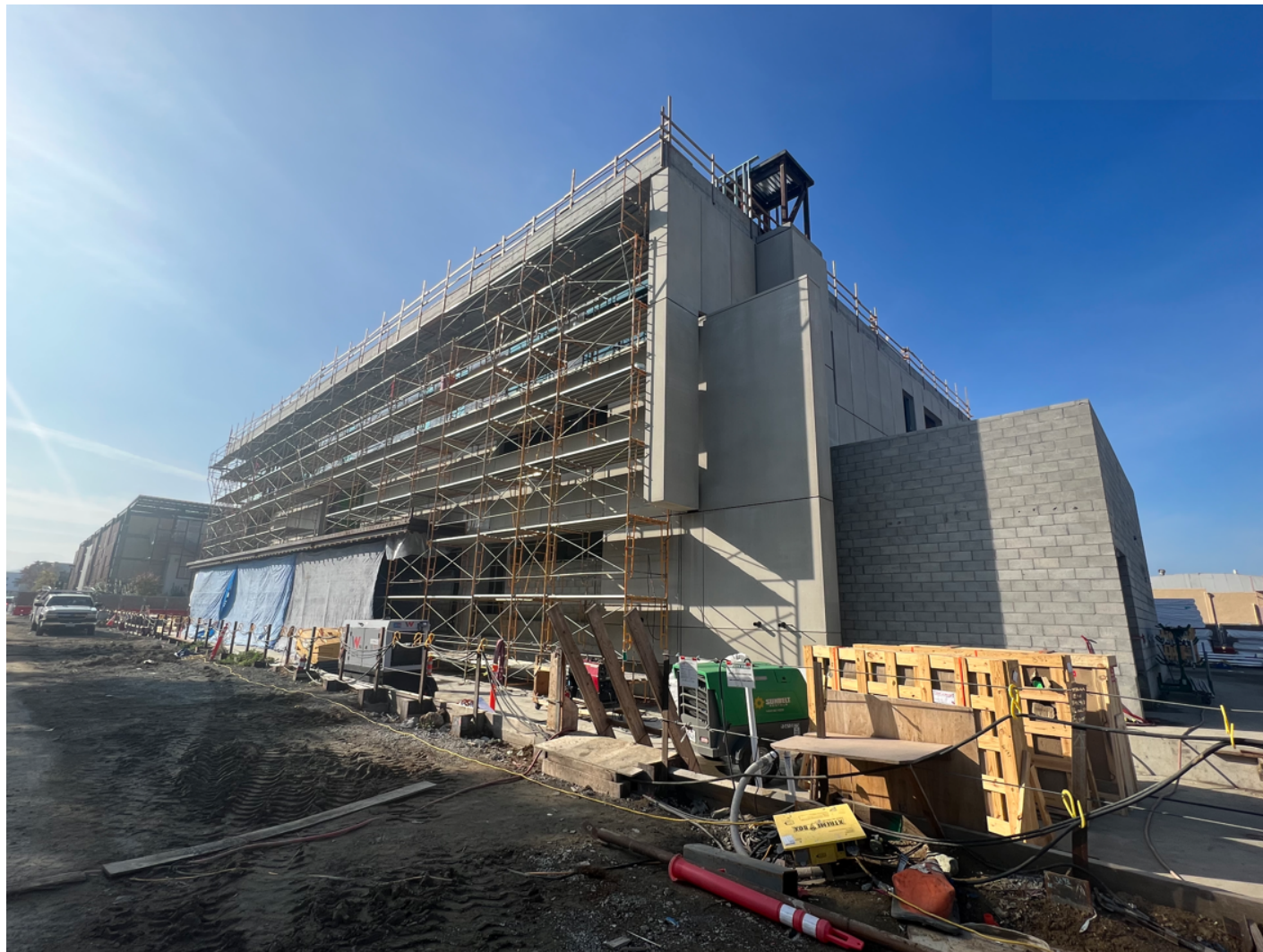
View from South East elevation.
