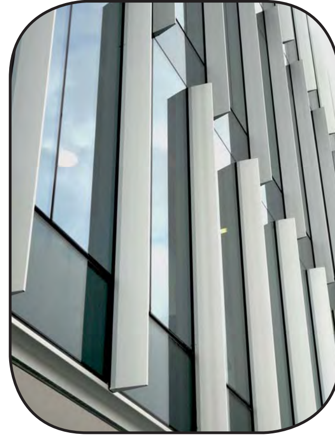
M9 Vertical Aluminum Fin White Mullion Caps where Shown (Basis of Design: Kawneer)
