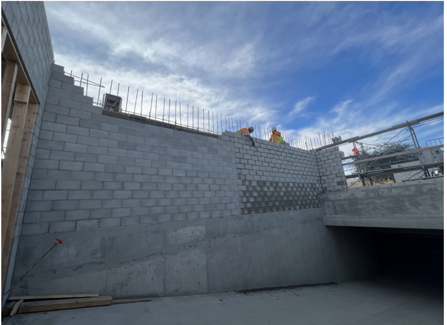
CMU wall at Garage Driveway.
