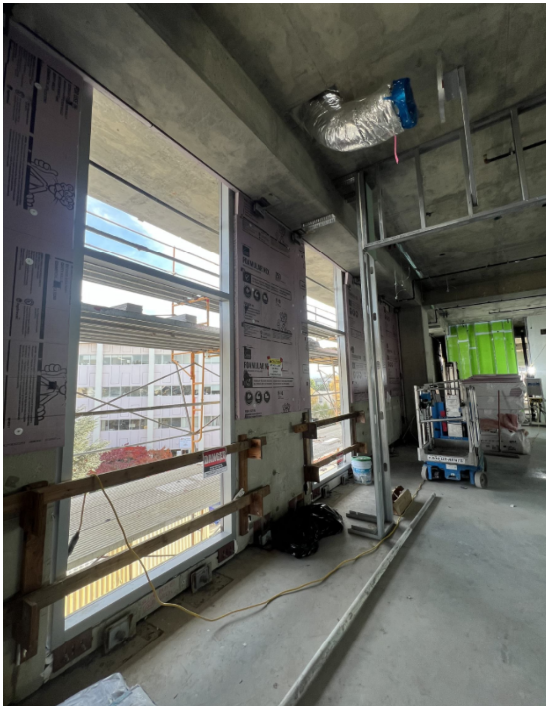
View of Window Frame install on Level 3.
