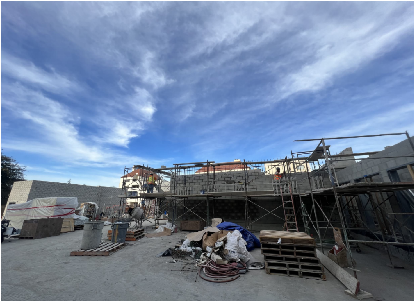
CMU Wall at Utility Yard.
