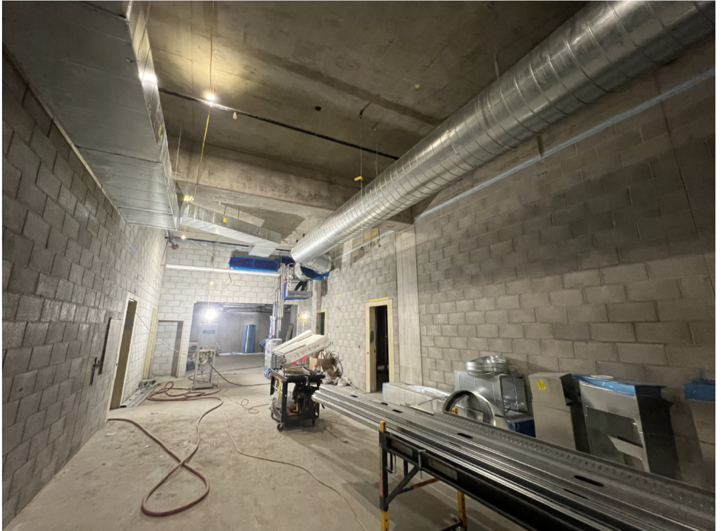
CMU wall at Salley Port.
