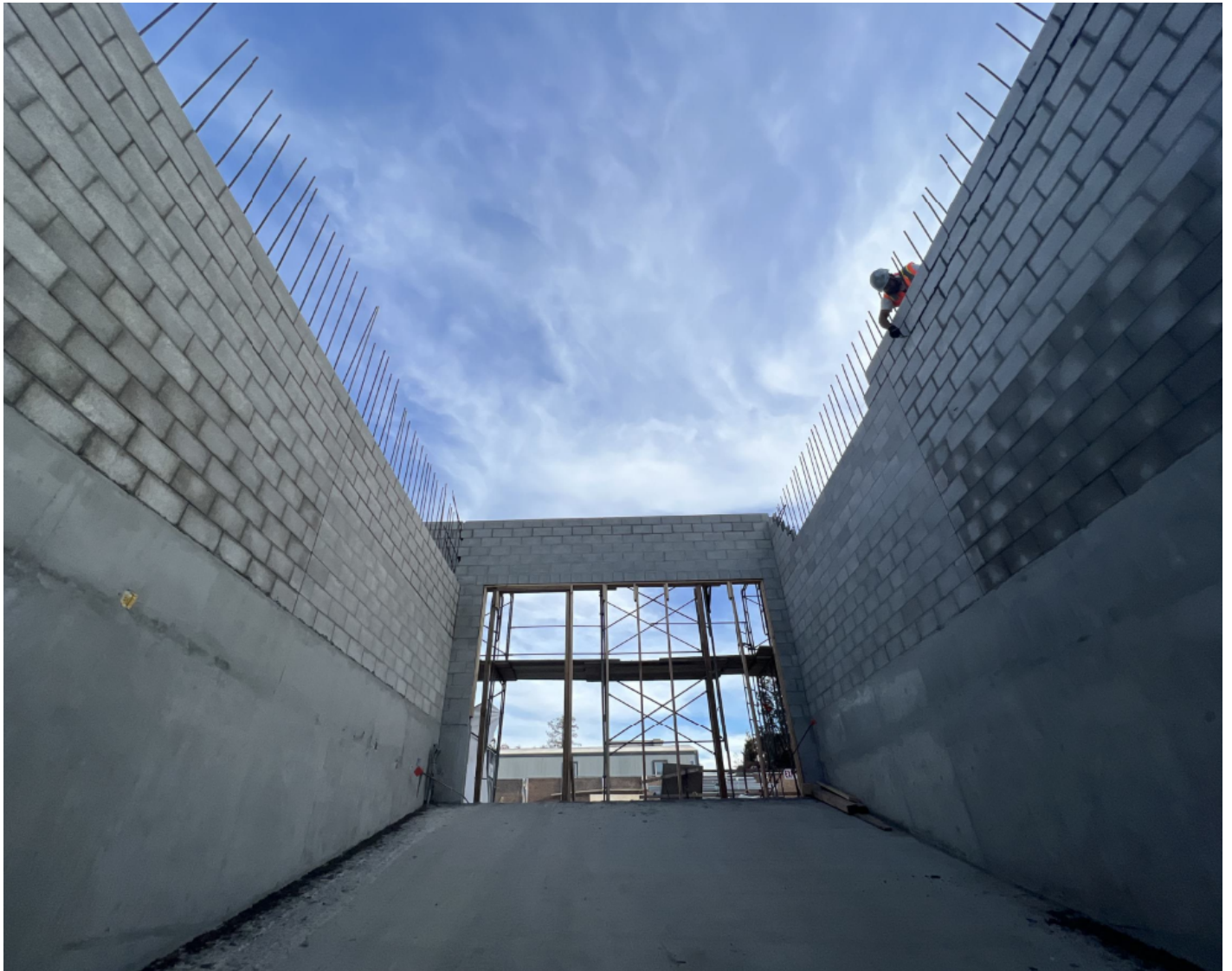
CMU wall at Garage Driveway.
