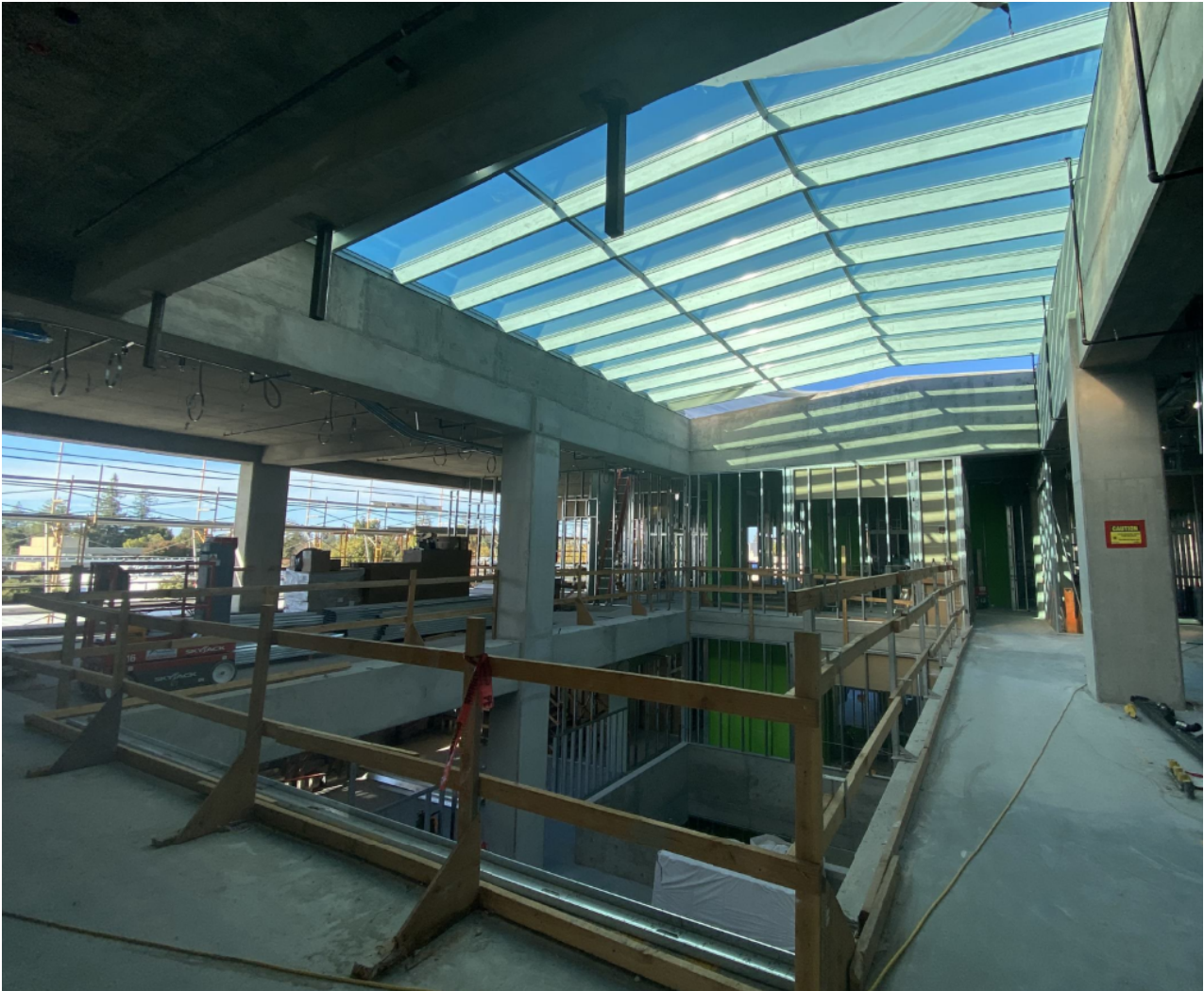
Skylight view and framing on Level 3.
