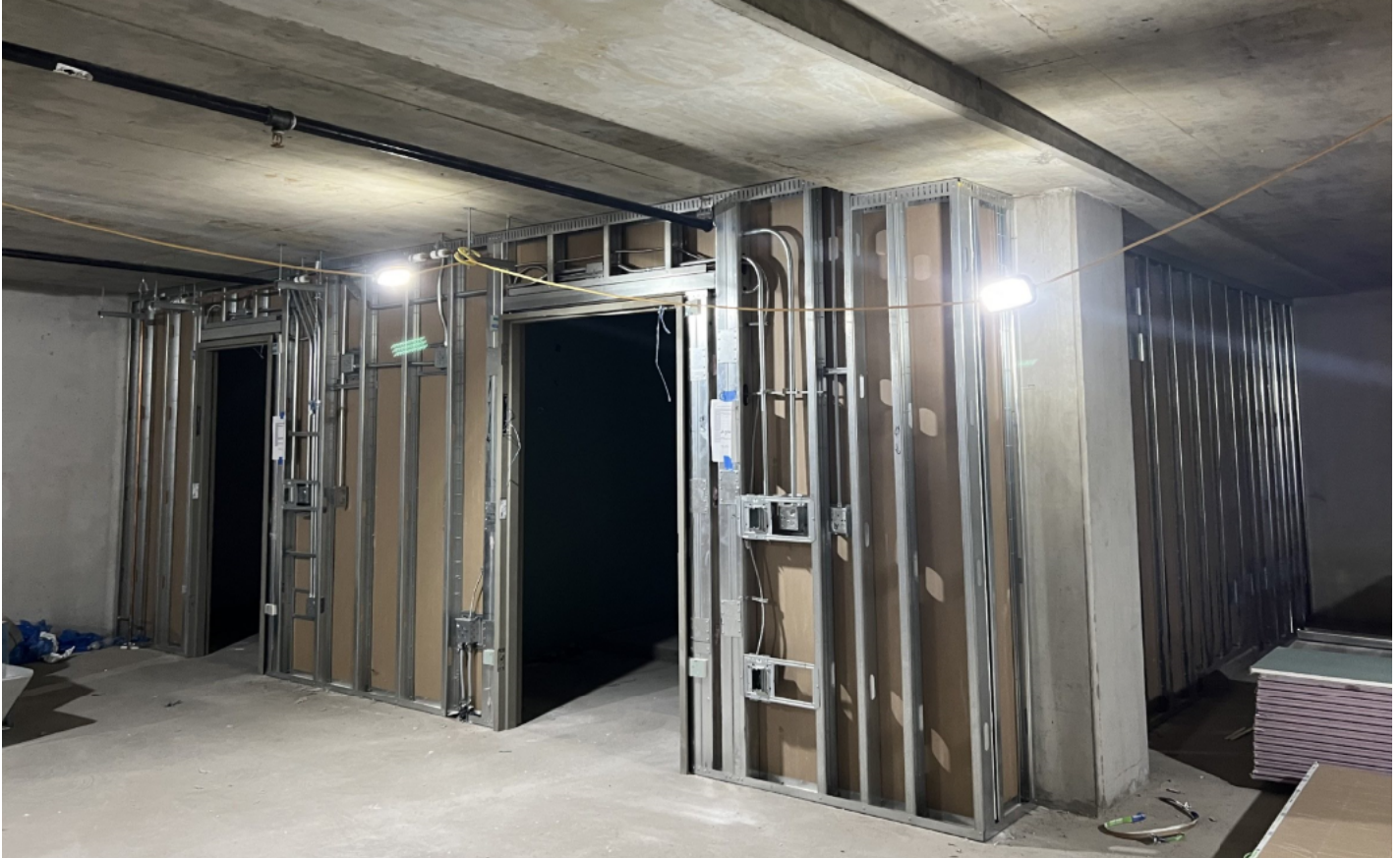
Basement level framing and one-sided drywall.
