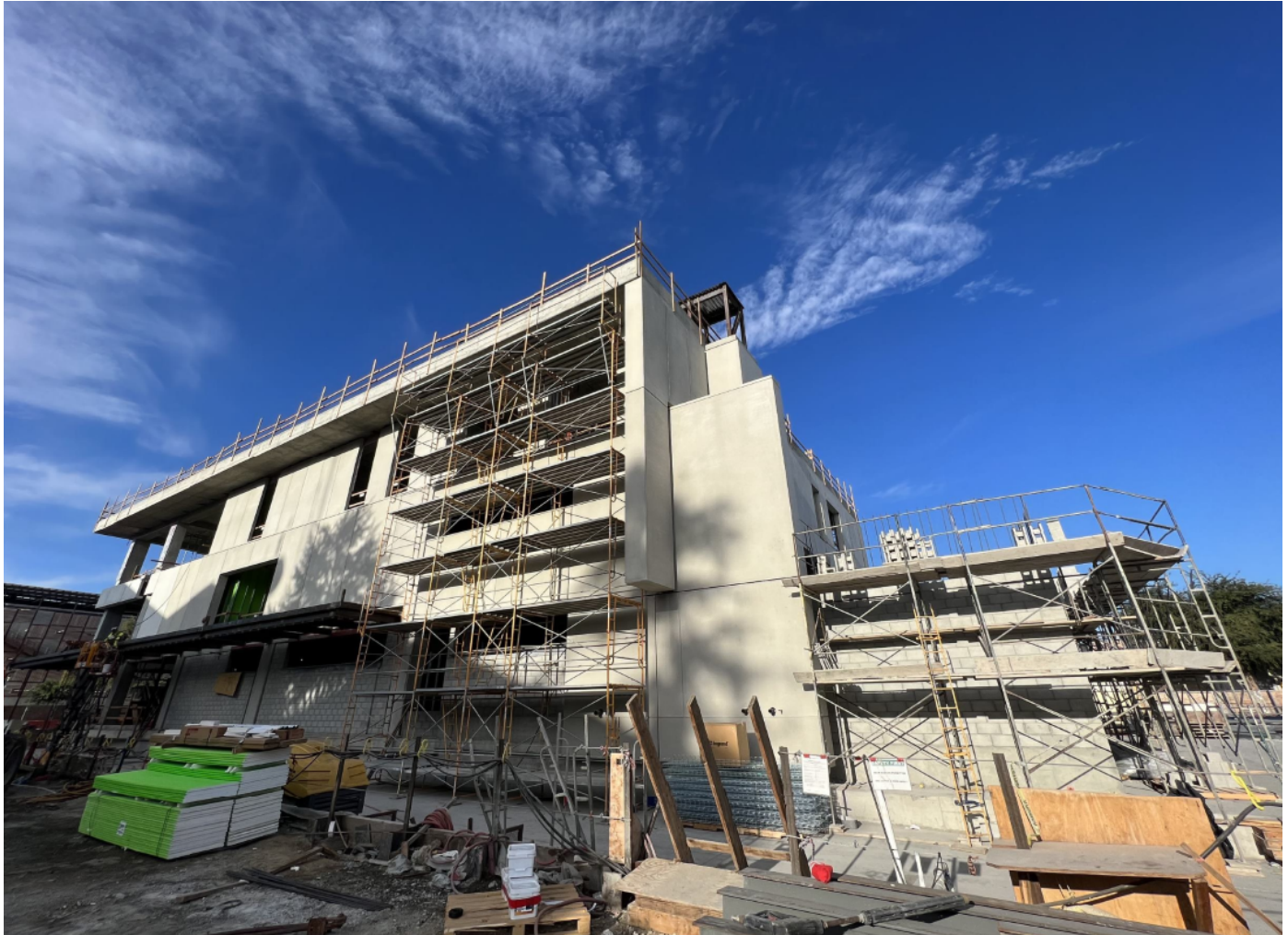
Precast and scaffold install at South-East Elevation.
