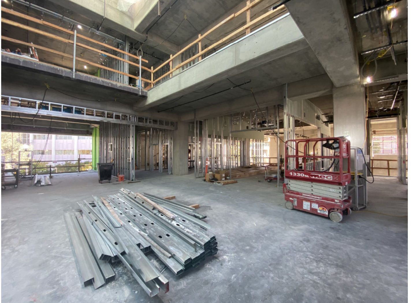
Framing and skylight view from Level 2.
