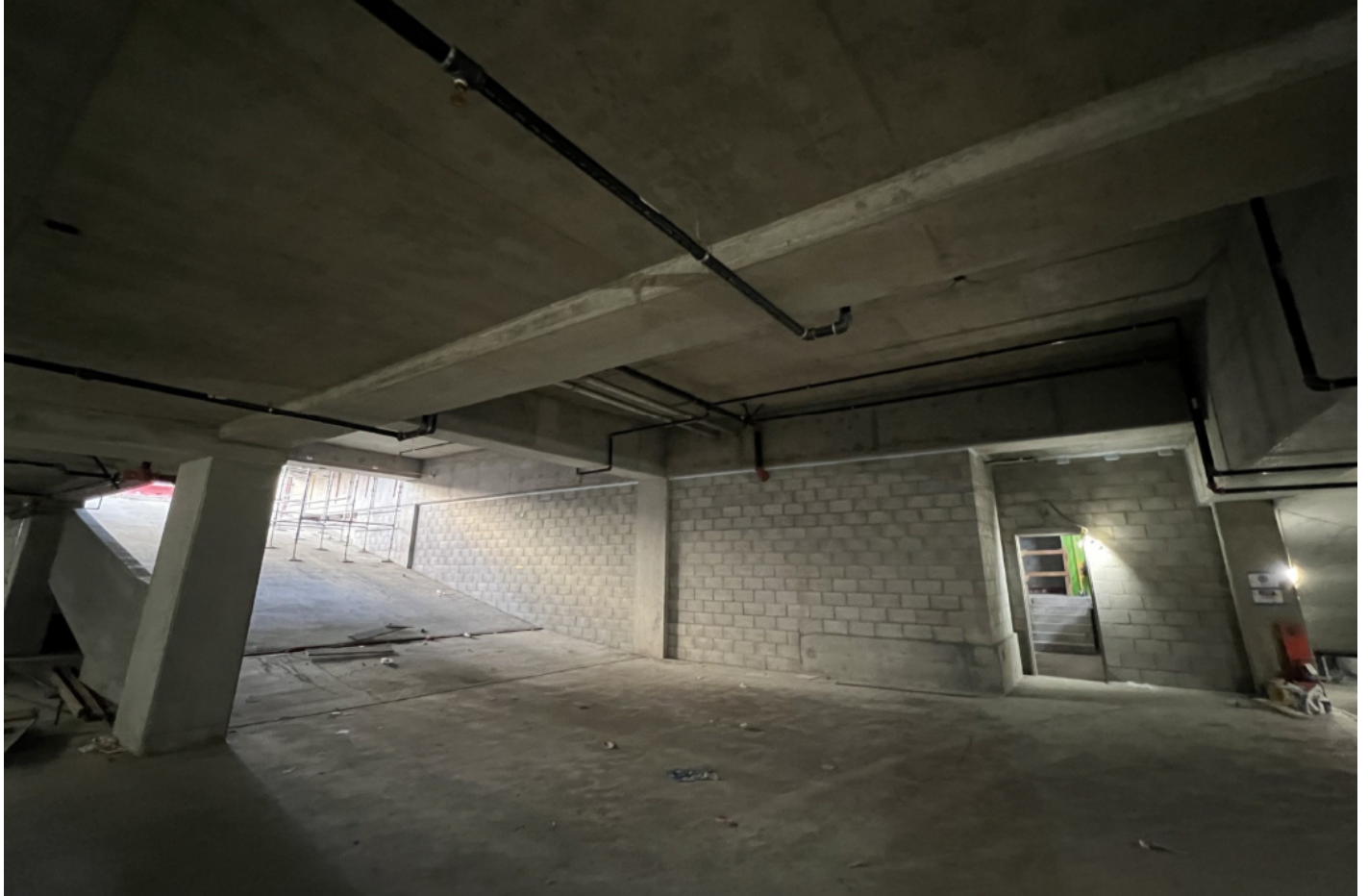
View of basement ramp into Basement Level 1.
