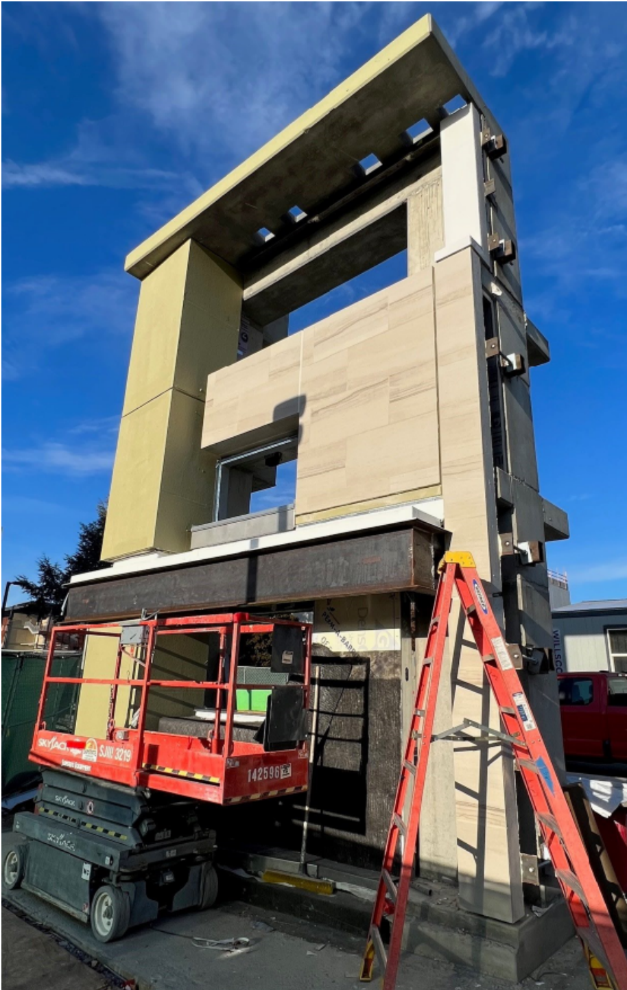
Continuation of Mock-Up install.
