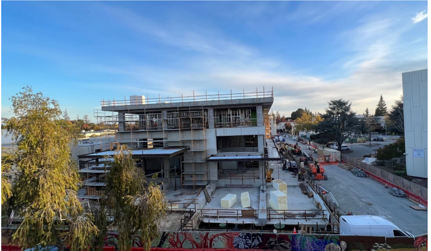
View from Sherman Avenue Parking Garage.
