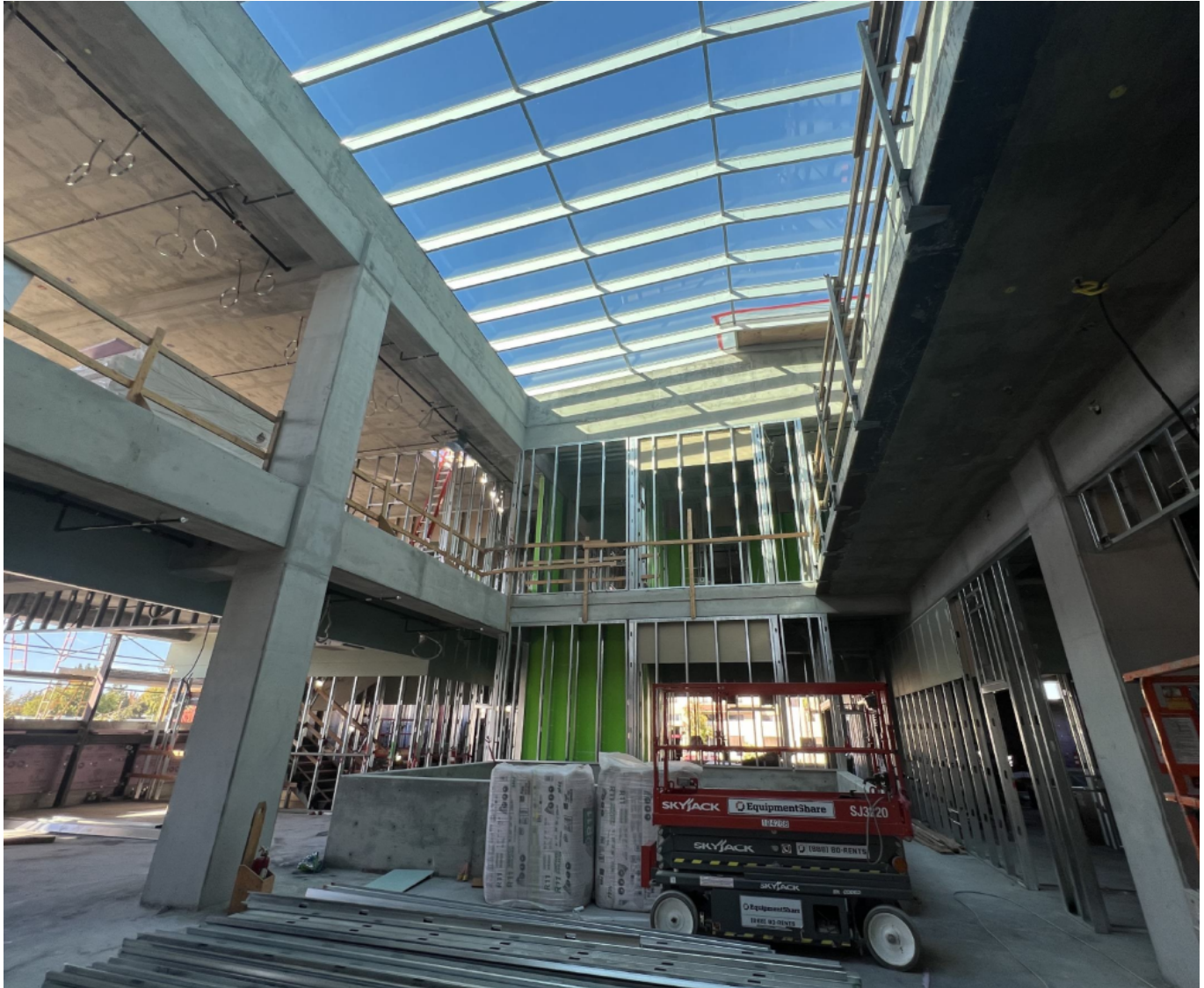
Framing and skylight view from Level 2.
