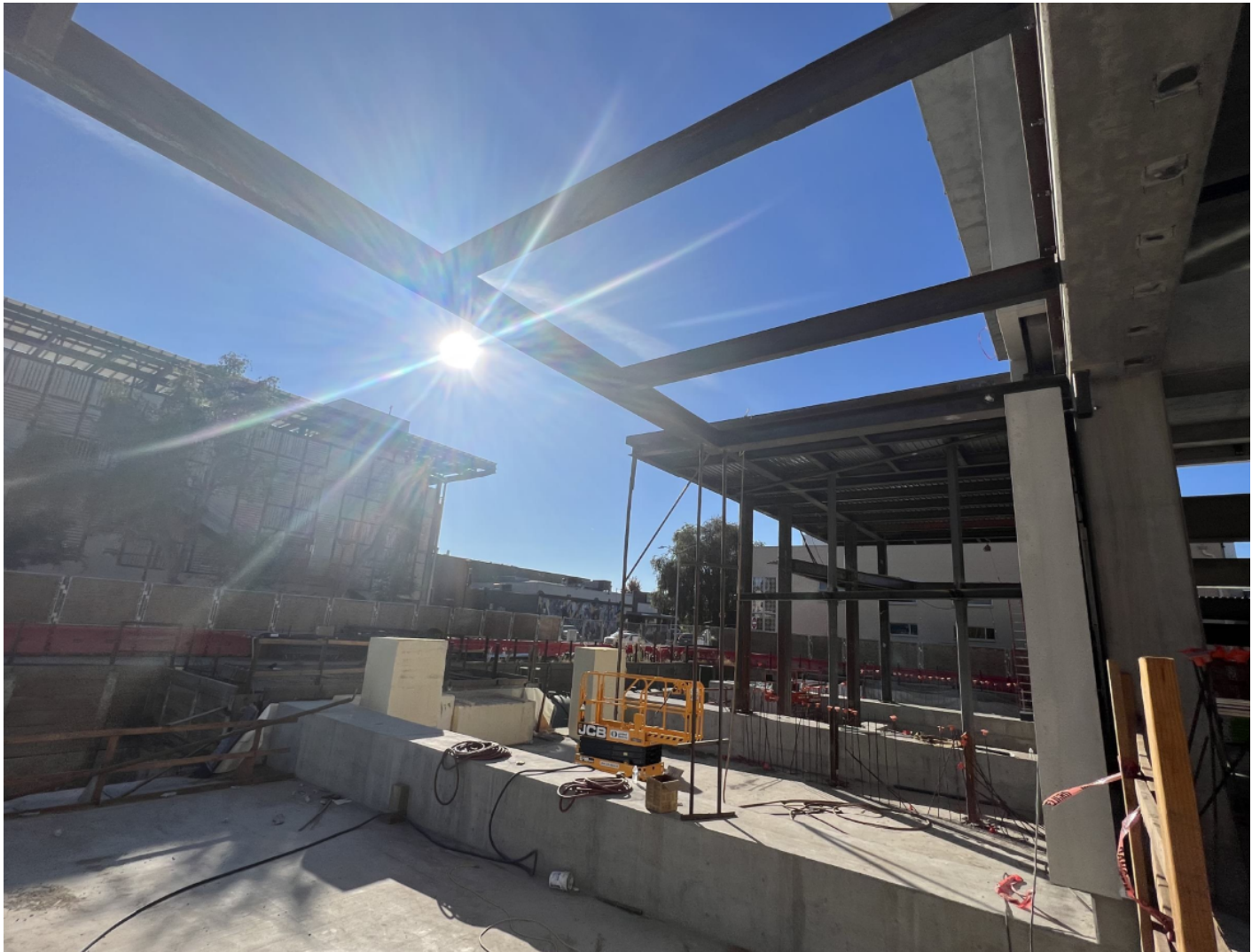
Multi-purpose room steel framing at West elevation.
