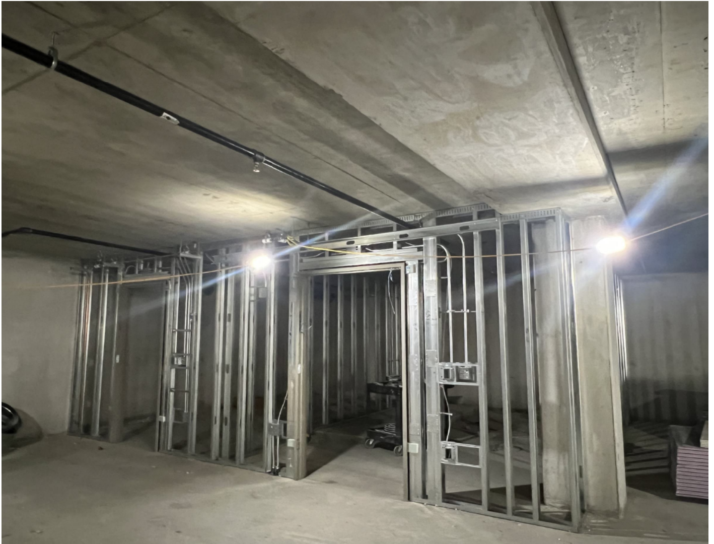
Basement level framing.
