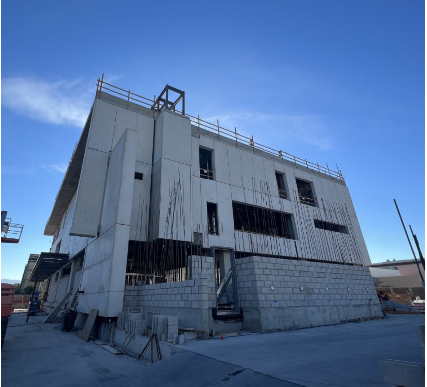
Precast install at East elevation.
