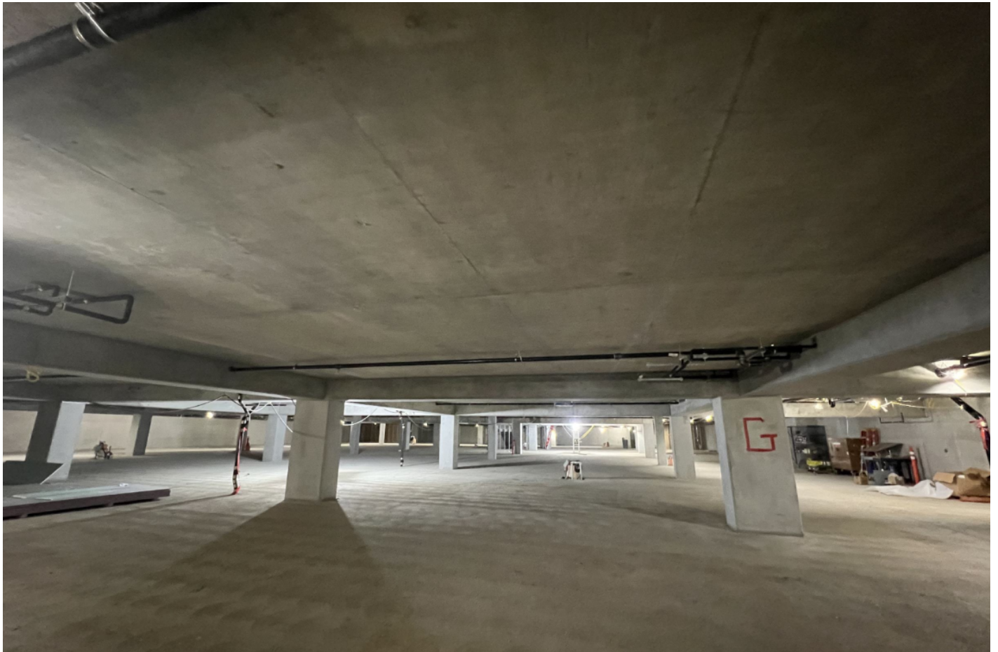
View of basement parking area.
