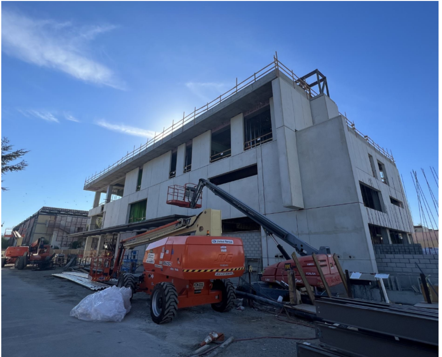
Precast install at South-East Elevation.
