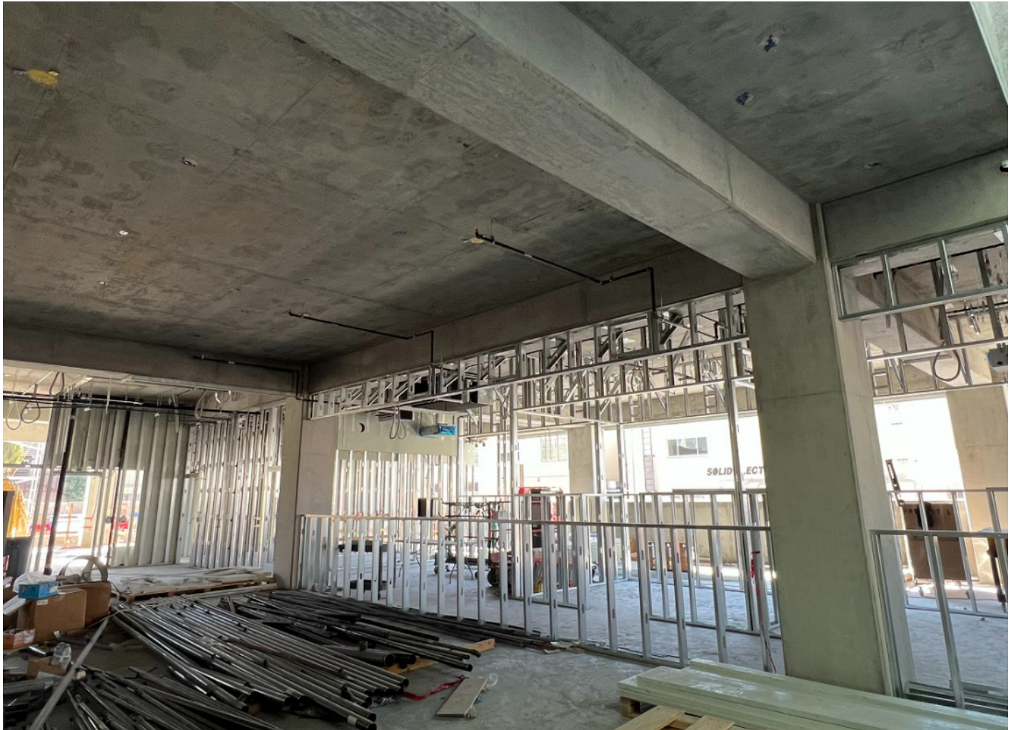
Framing on level 1.
