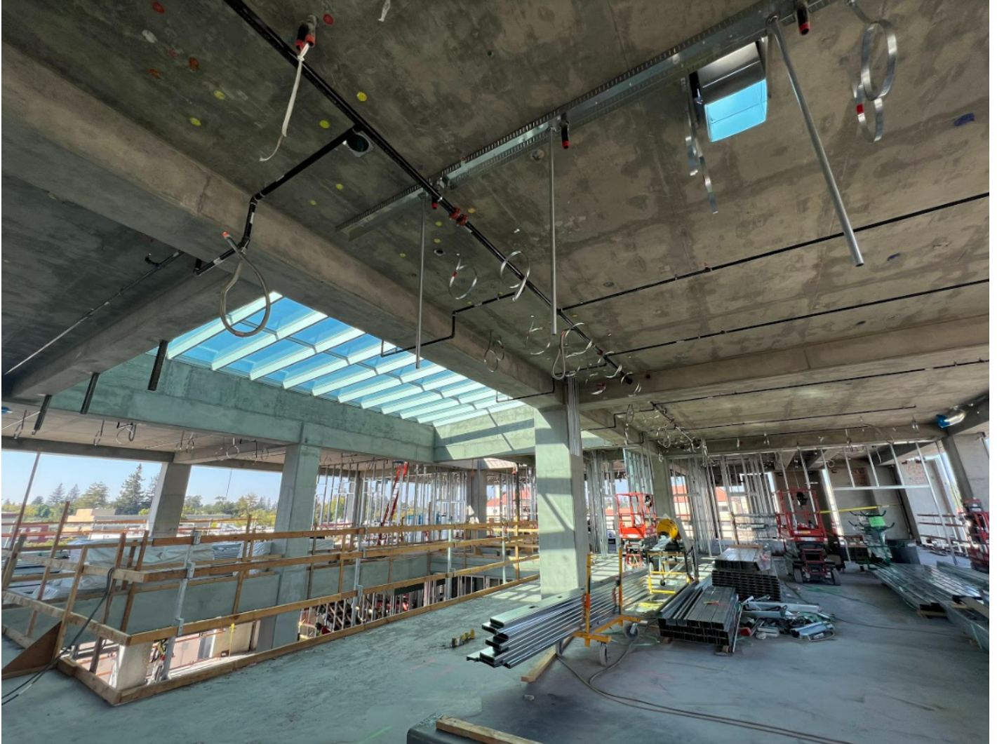
Skylight view and MEP inserts on Level 3.
