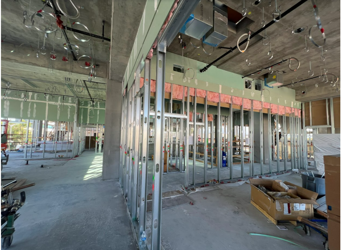
Framing and MEP inserts on Level 2.
