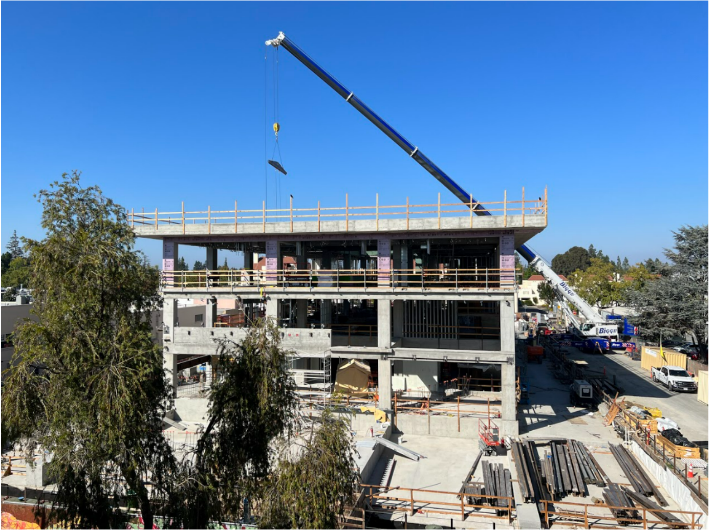
Placement of CMU walls, cement board, and framing.
