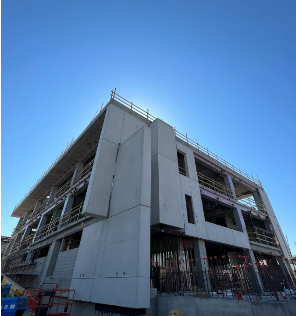
Precast install at South-East Elevation.
