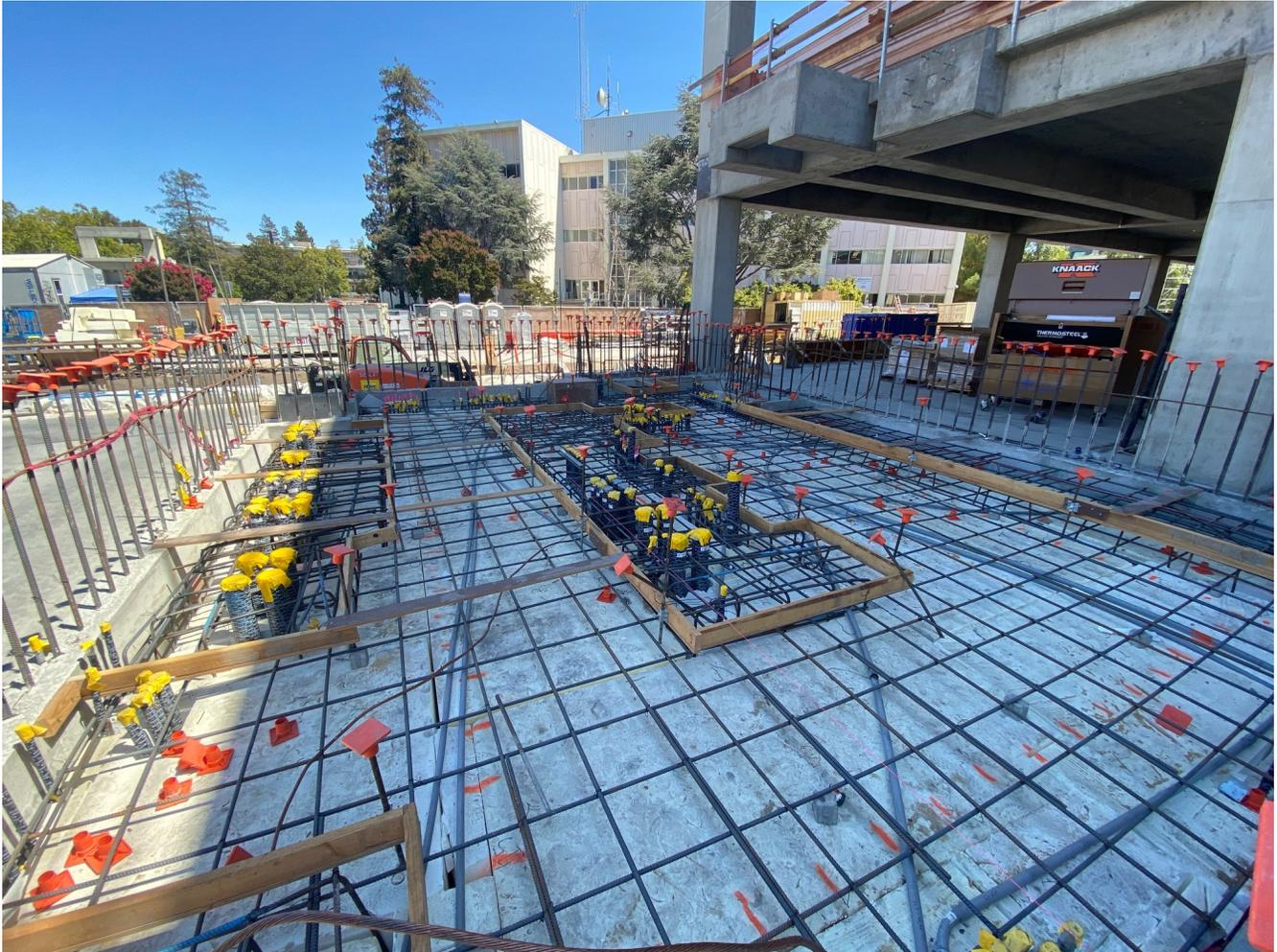
Structural foam, rebar, conduits, and formwork in place in the Utility Yard.
