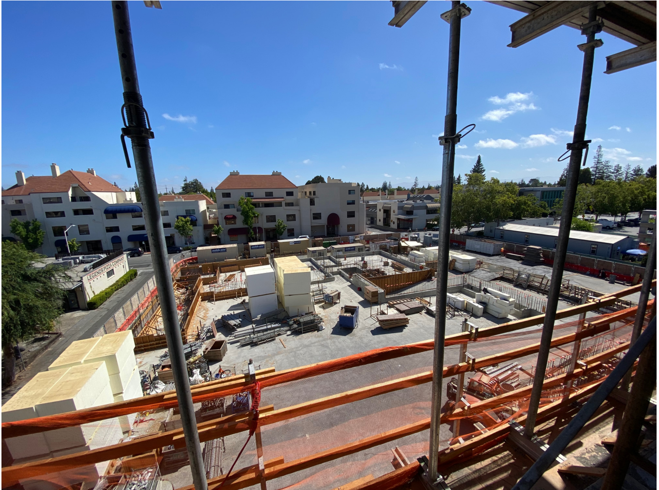
Looking down at future Utility Yard from Level 3.
