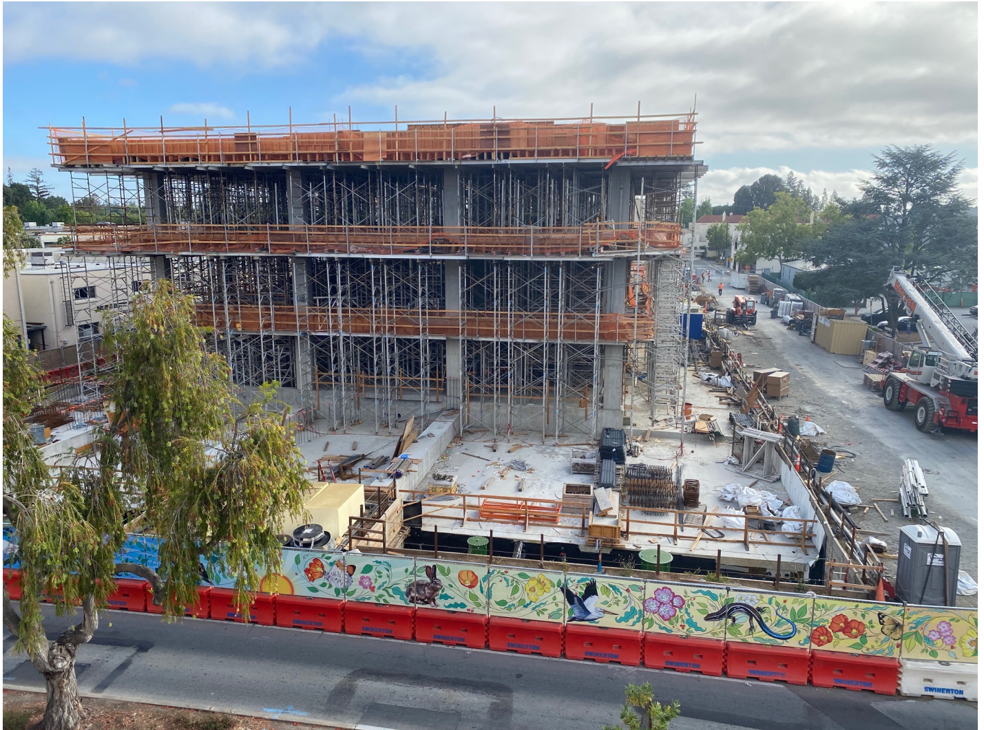
Formwork in place for Level 4 (roof) concrete slab.
