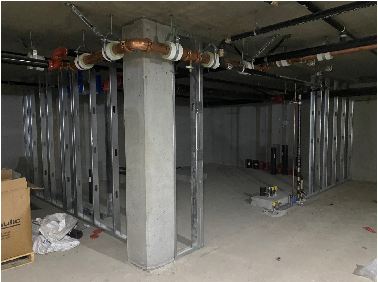
Metal framing and overhead MEP being installed in Level B2.
