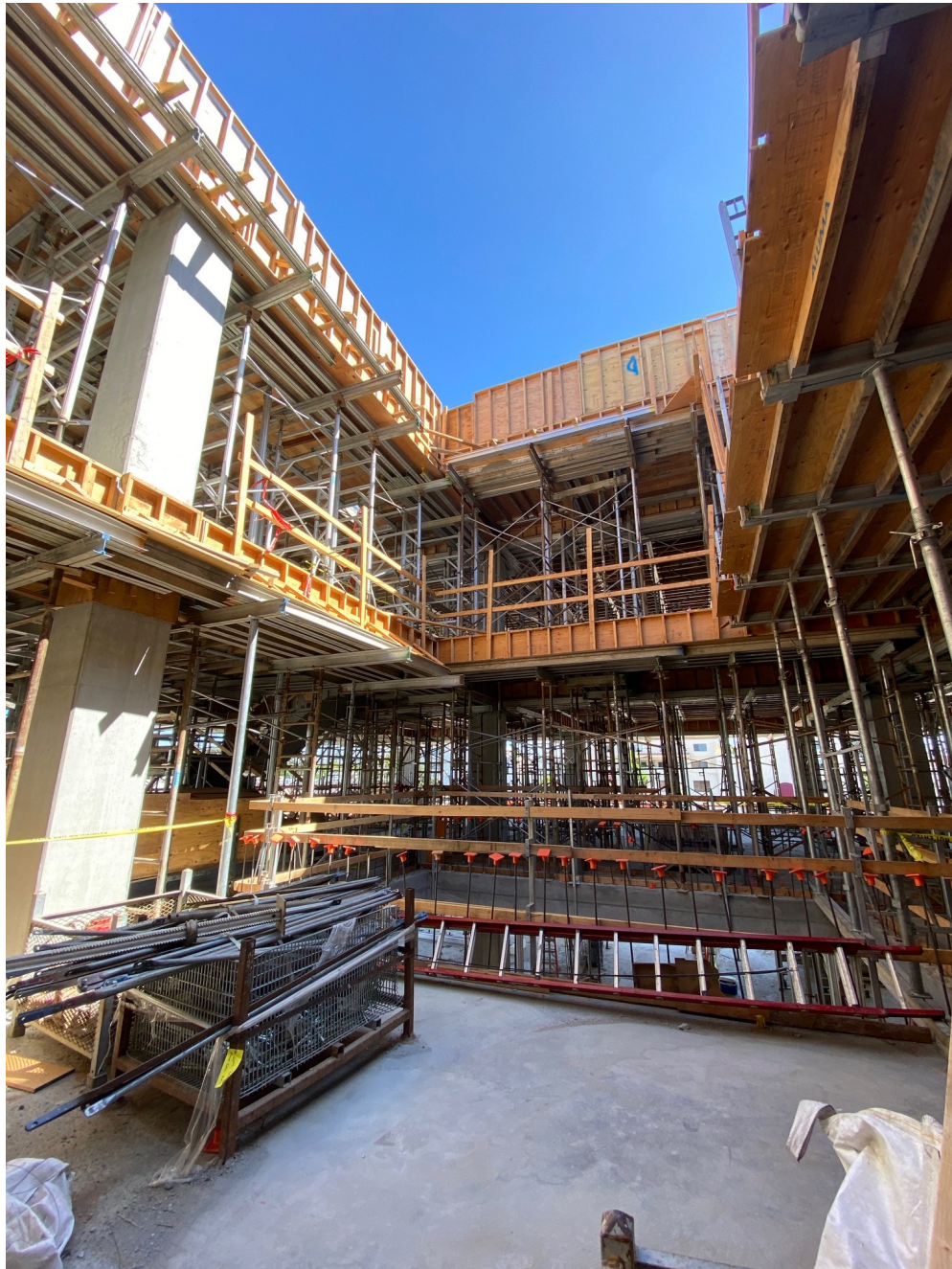
Looking up through future skylight from Level 2.
