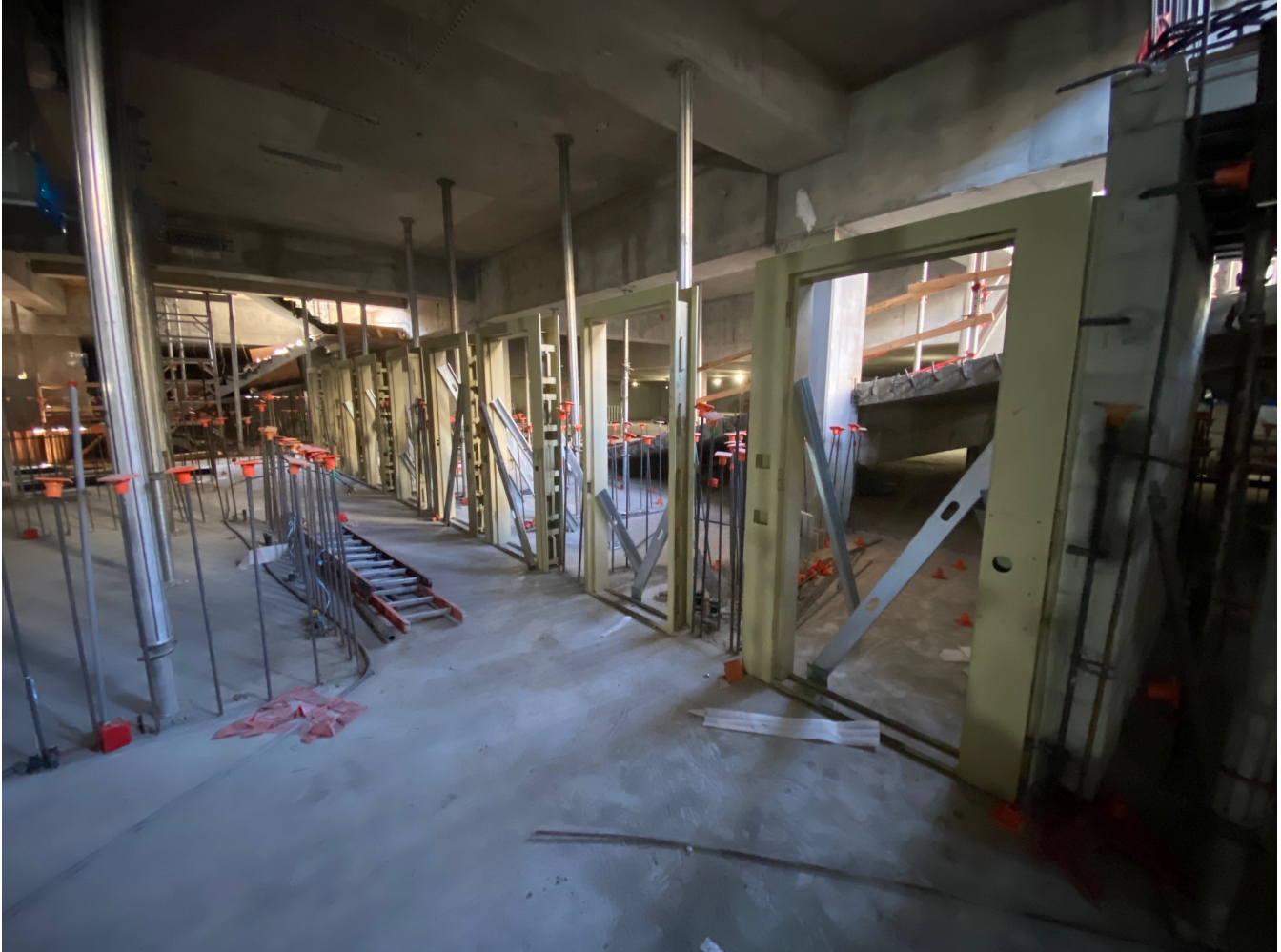
Door frames/thresholds being installed in Level B1.
