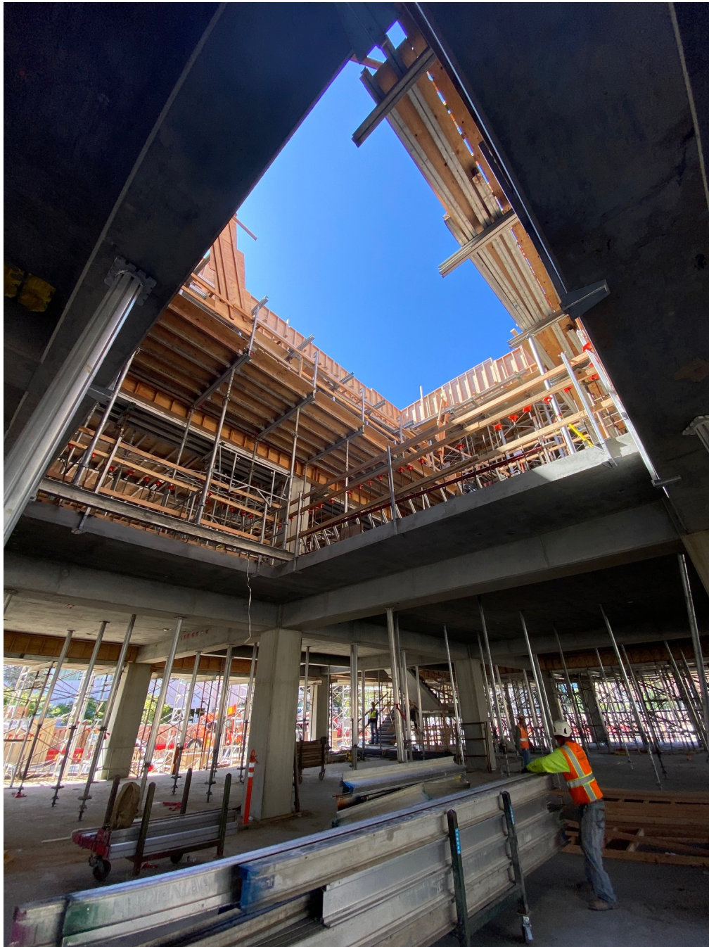
Looking up through the future skylight from Level 1.
