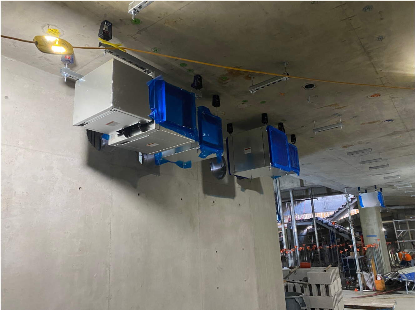
Mechanical ductwork being installed in Level B1.
