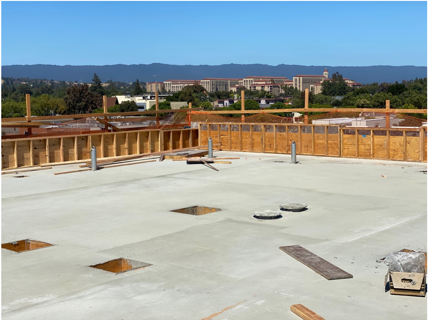
Concrete slab on Level 4 (roof) and concrete formwork in place.
