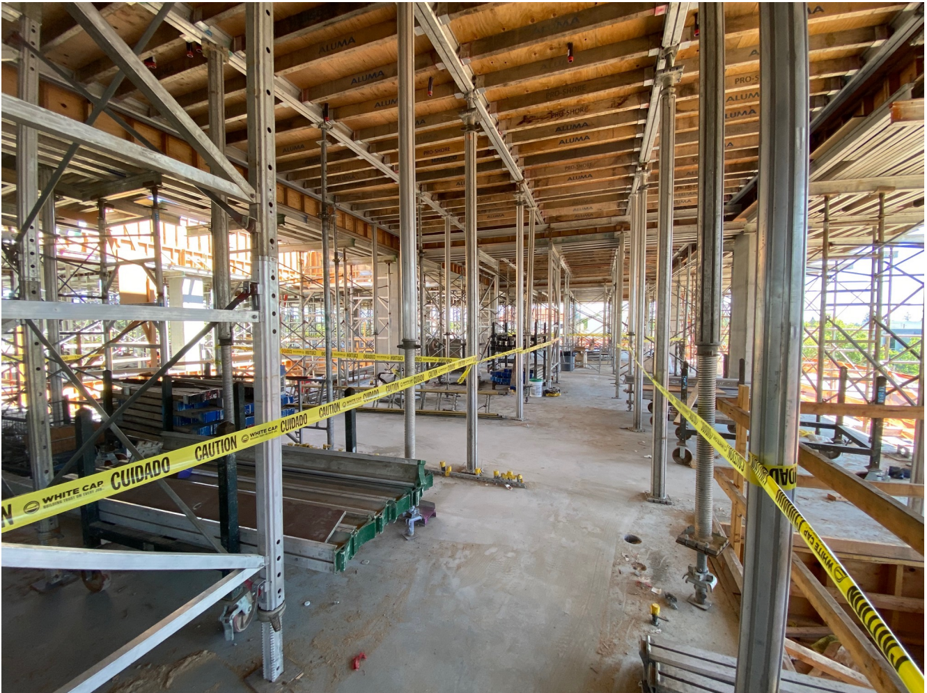
Concrete slab formwork in place on Level 3.
