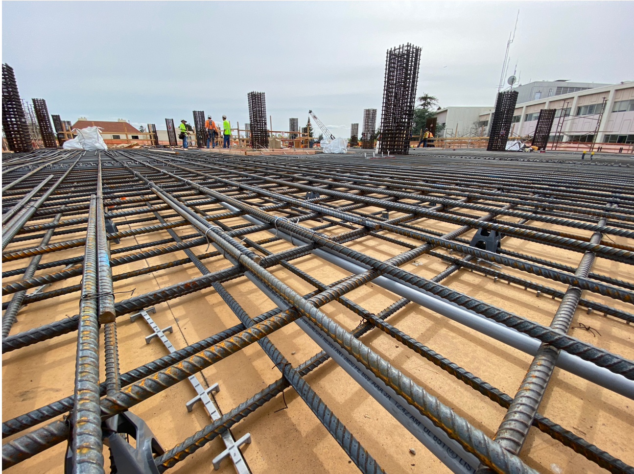
Formwork and rebar in place for Level 3 concrete slab.
