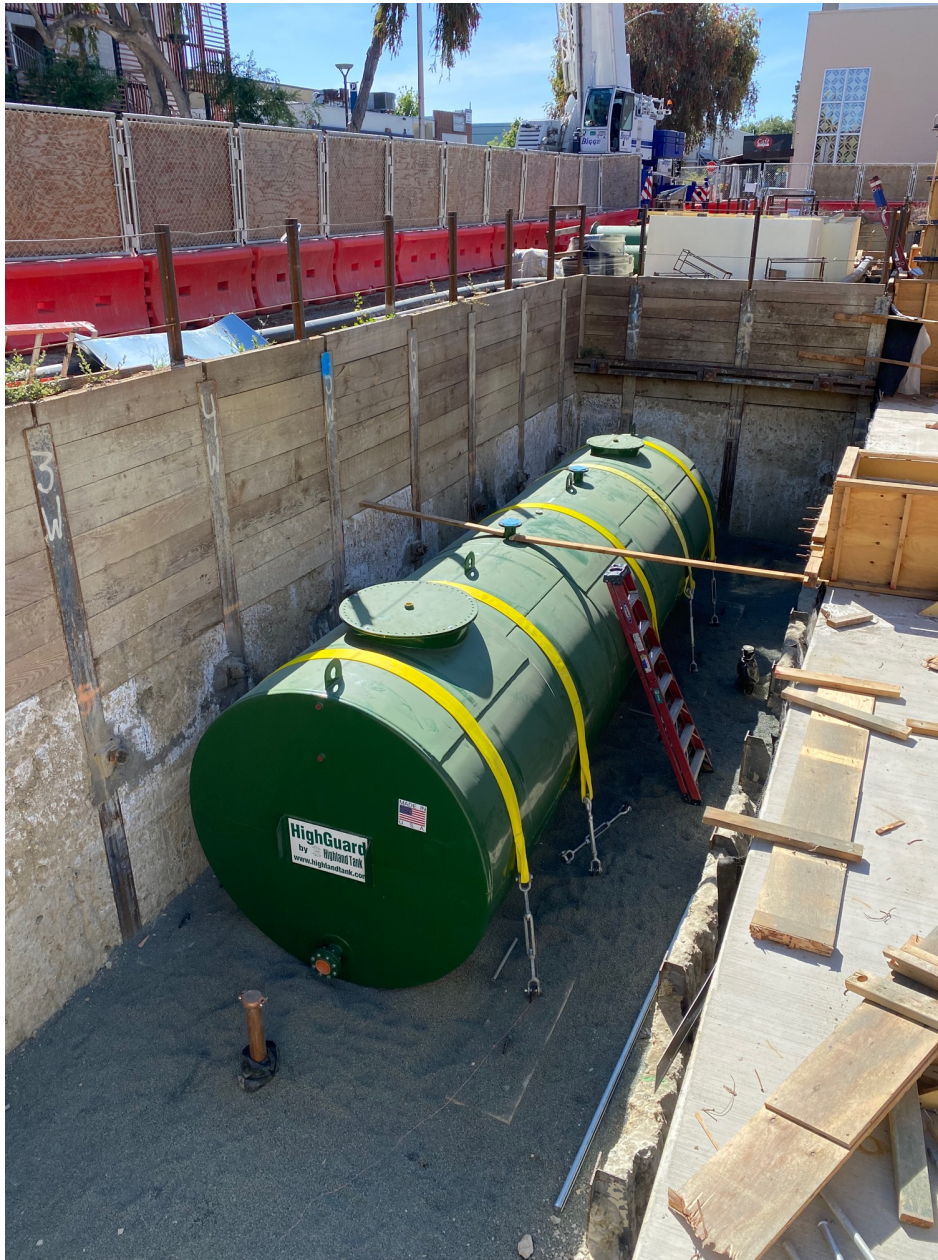
Potable water tank in place.
