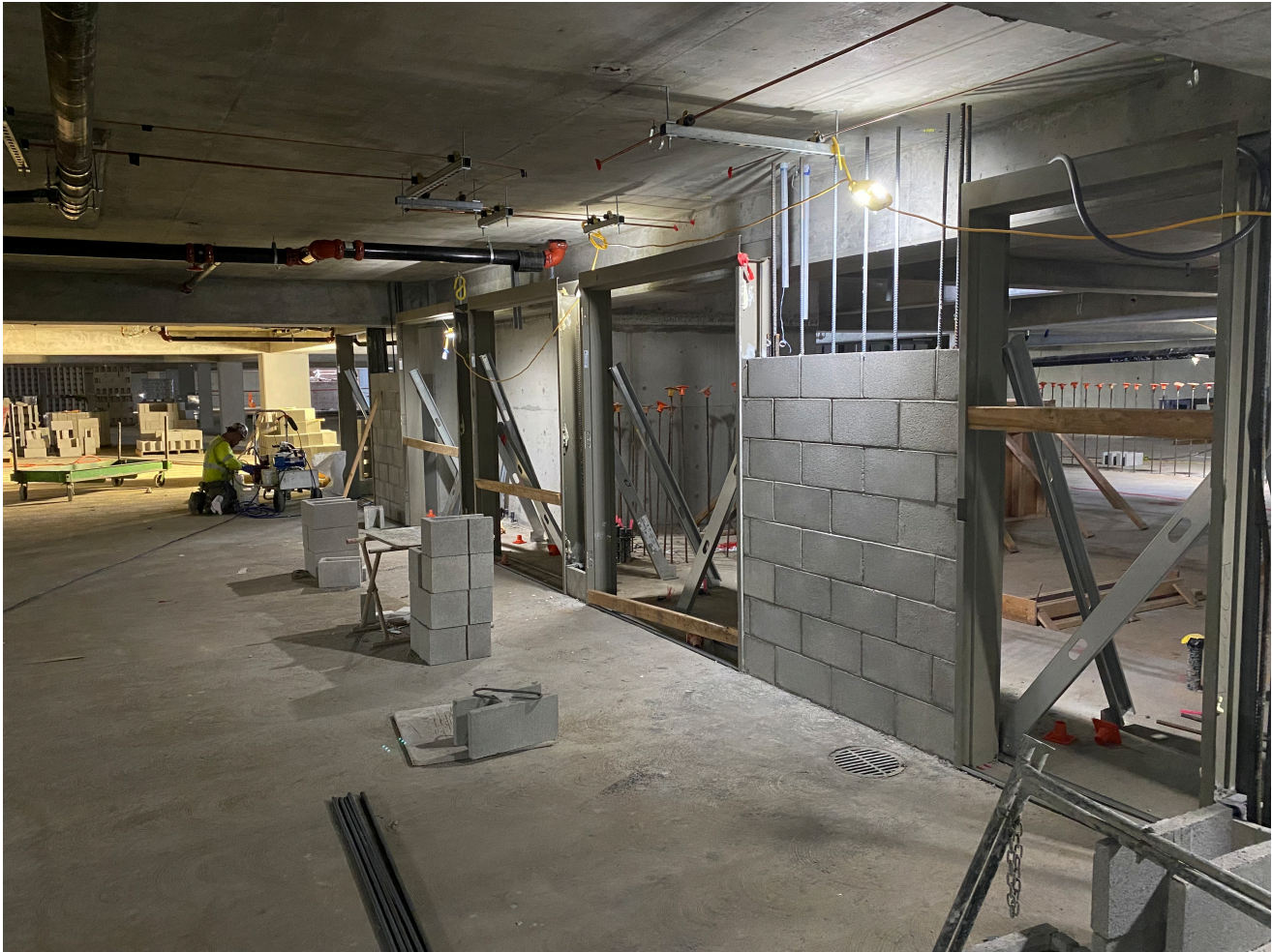
Concrete masonry unit (CMU) wall installation ongoing on Level B2.
