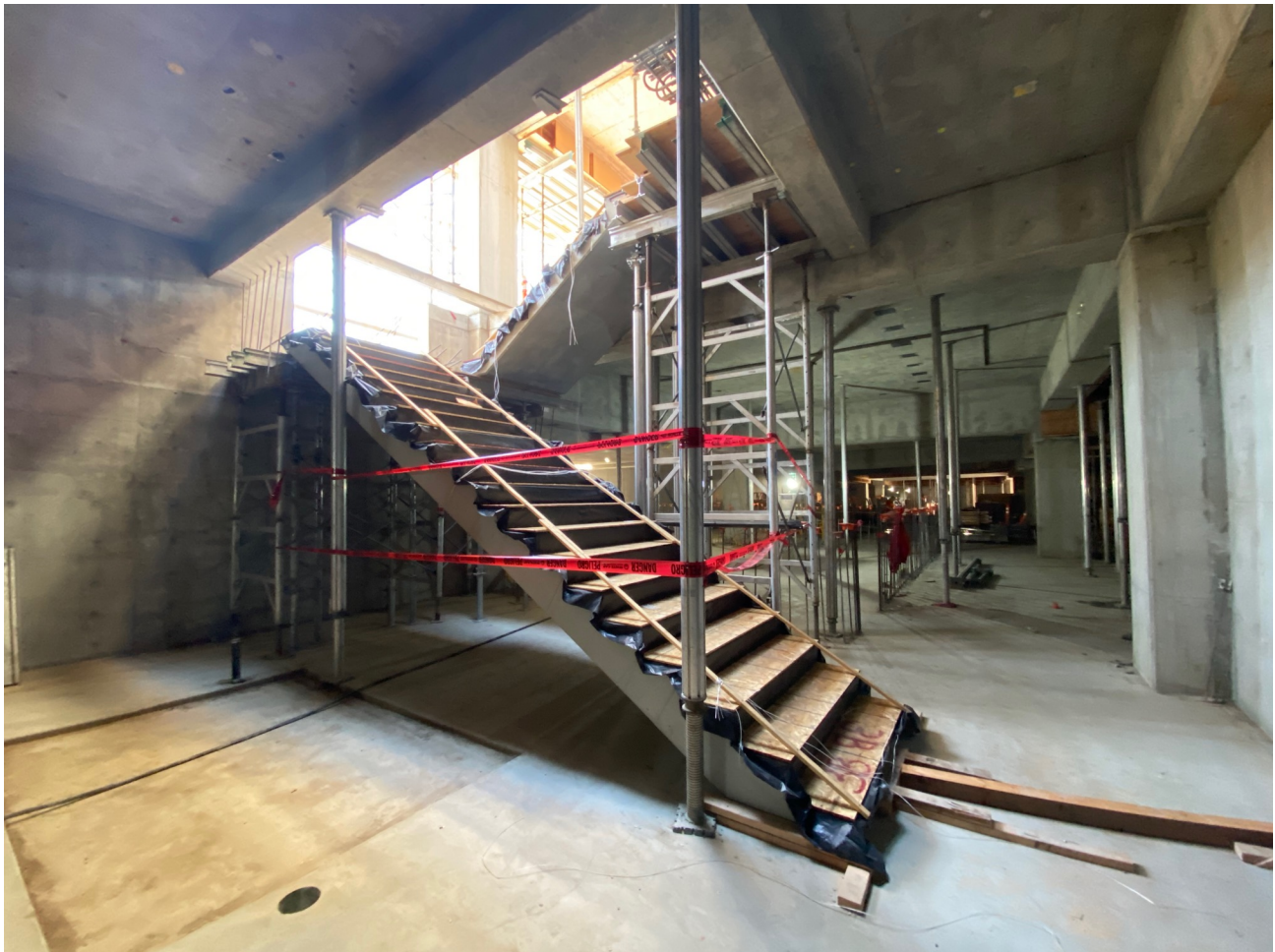
Precast concrete stairs in place between Level B1 and Level 1.
