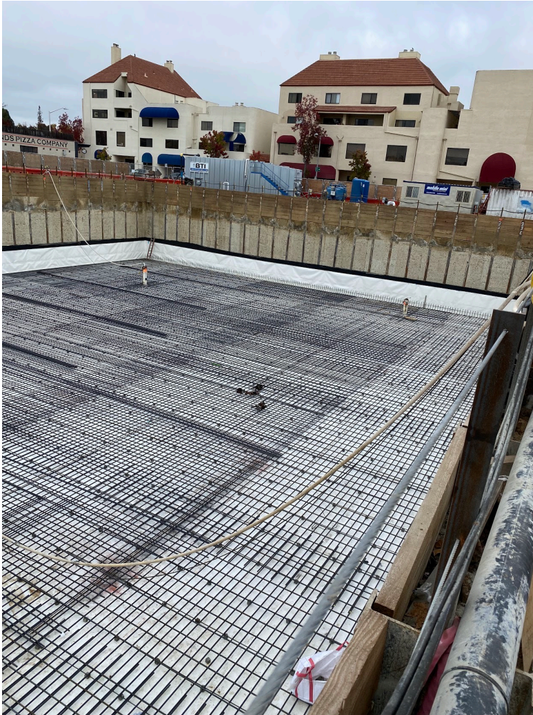
Rebar and Waterproofing in place in Area B.
