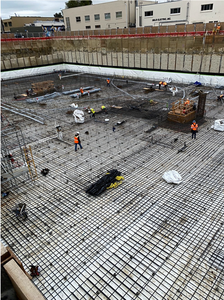
Rebar and Waterproofing in place in Area A.
