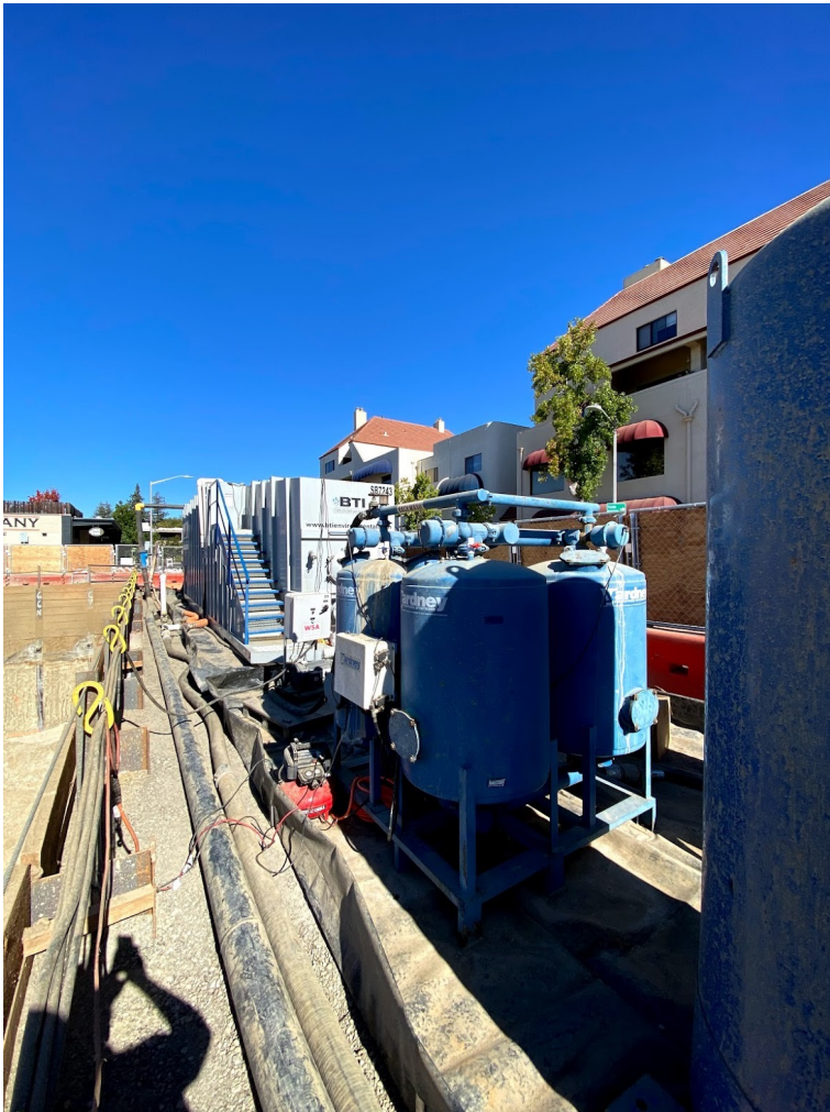
Dewatering pumping and treatment equipment installed.
