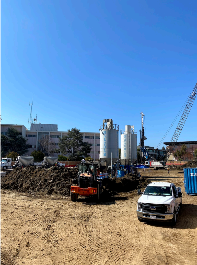
On-Site Batch Plant for Shoring Wall
