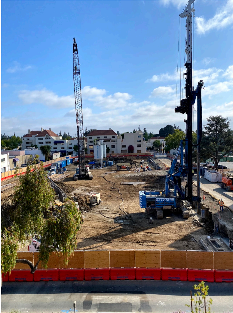
Shoring Wall Installation
