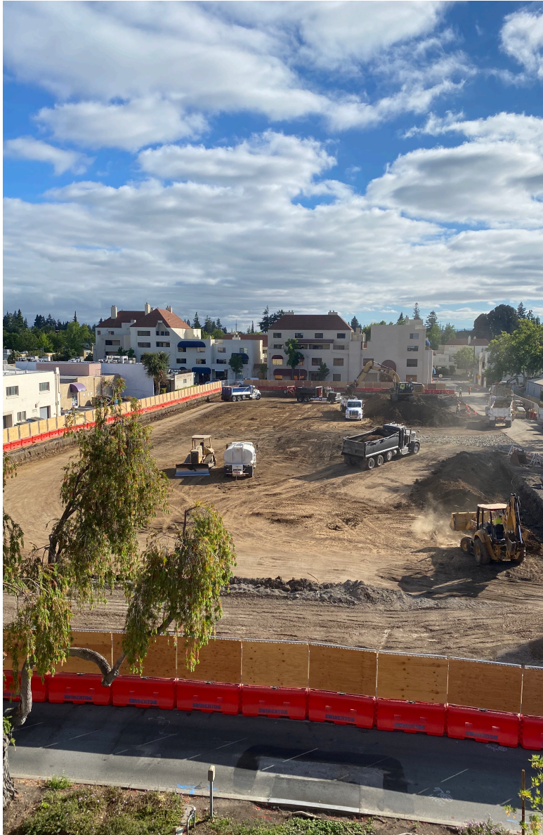
Preliminary site soil excavation.
