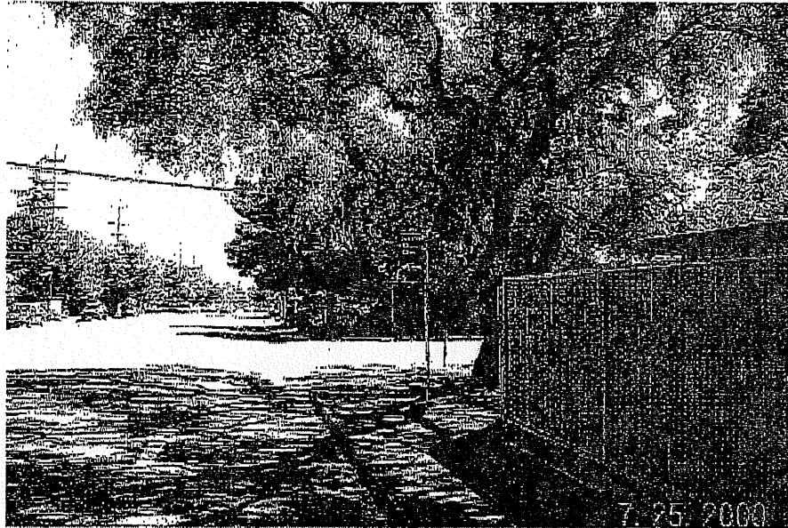
(13) #127910 EB W. Charleston Road NS Ruthelma Ave. *Install 10'x55' PCC Bus Pad
