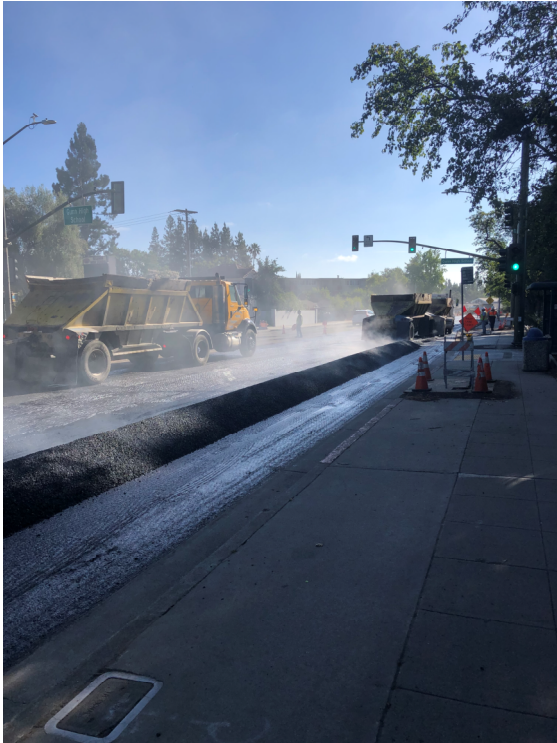
Asphalt Milling
