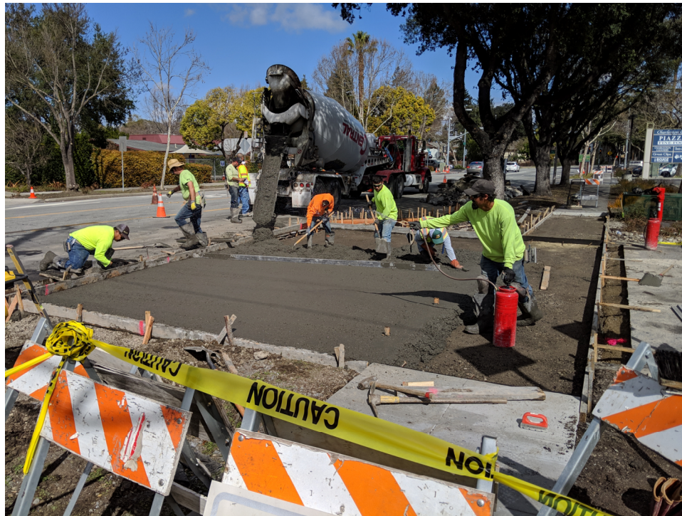
Concrete forming, pouring, and sidewalk work
