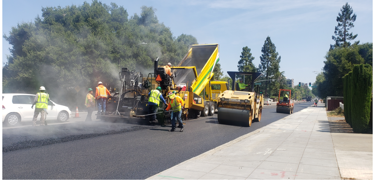
Asphalt Paving
