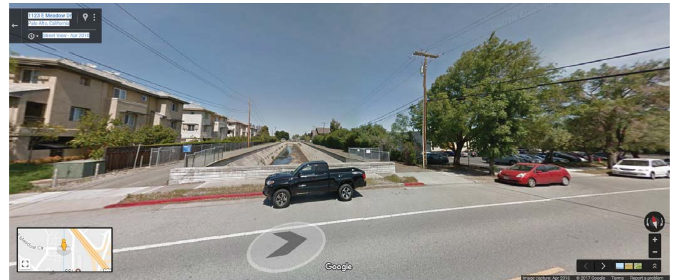
East Meadow Drive at Adobe Creek (Looking North)
