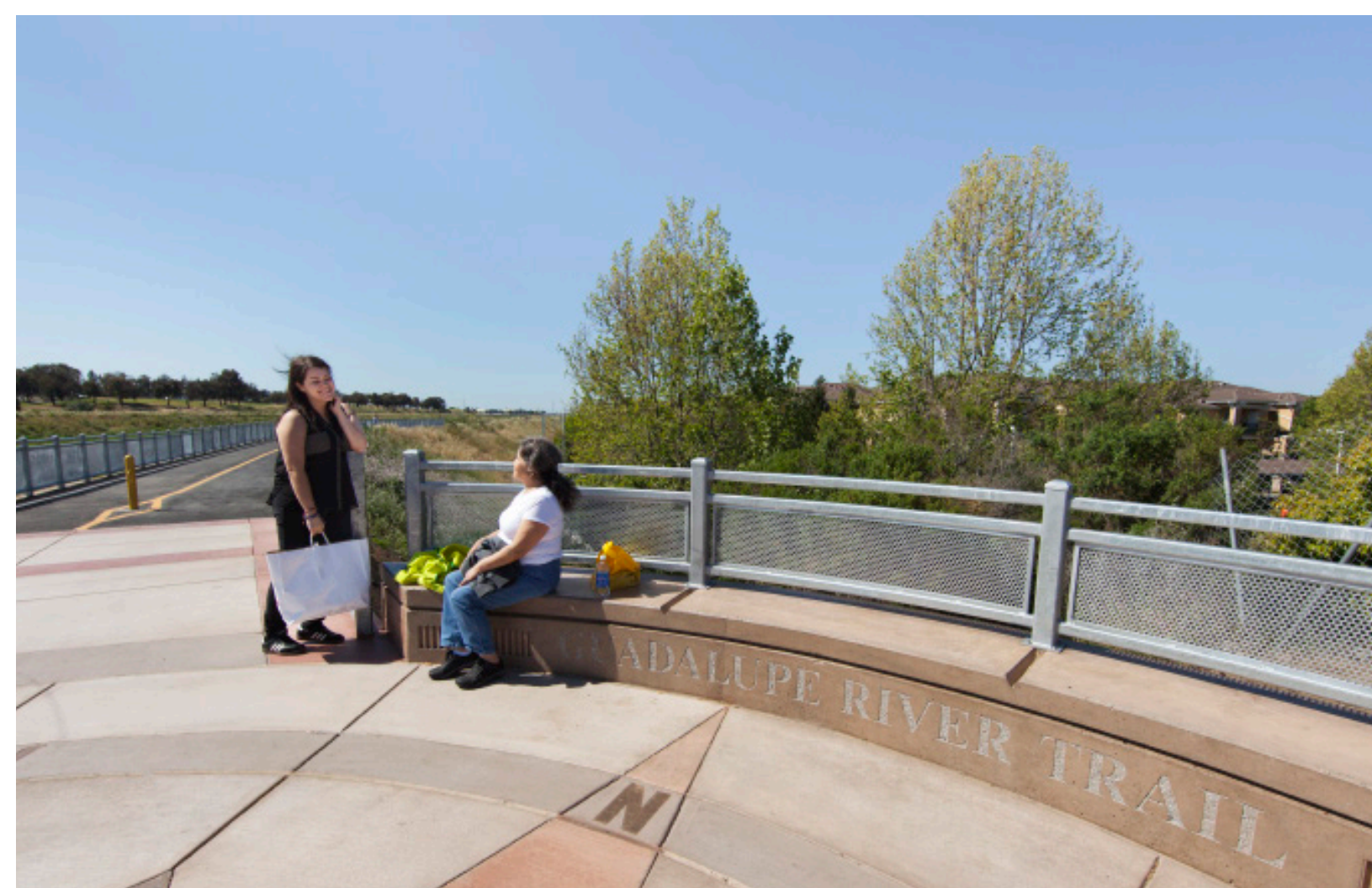
Concrete Seatwall and Railing
