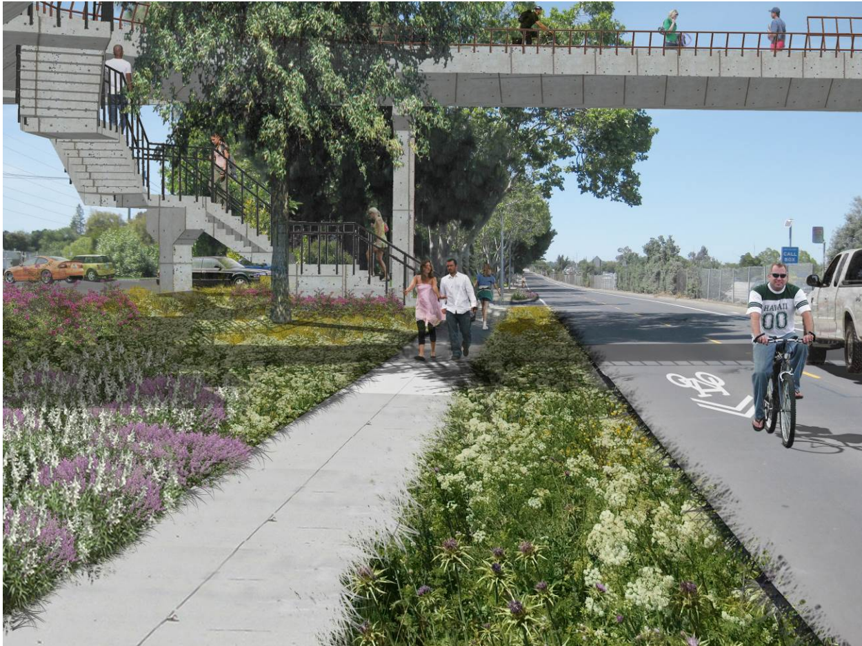
Figure 11. Photosimulation of bridge at 3600 West Bayshore Road with secondary stairway access and sidewalk improvements.
