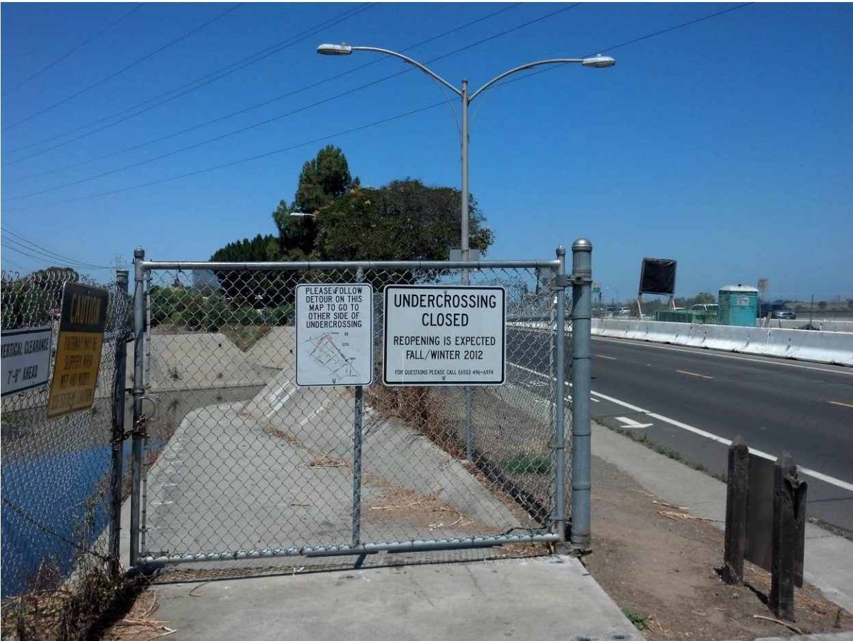
Existing Benjamin Lefkowitz Seasonal Underpass at West Bayshore Road
