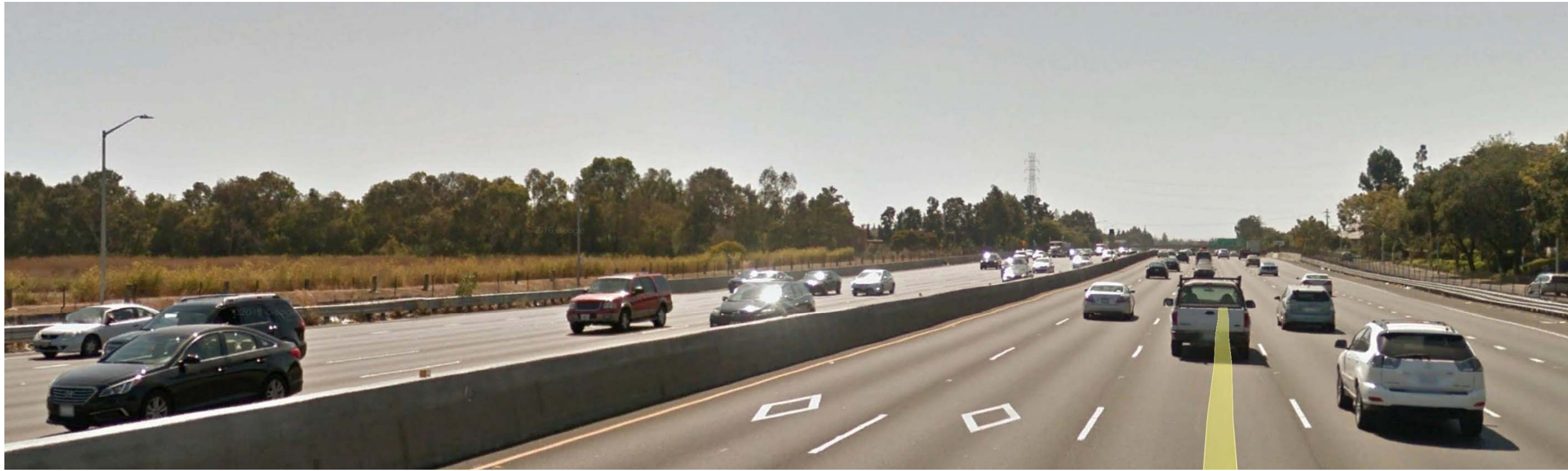
Figure 2: Existing Condition from Key View 1
