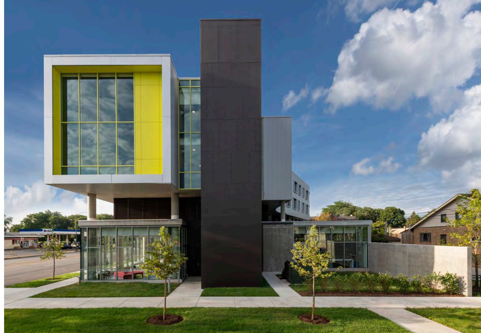
Figure 47 Urban form design standards requires setbacks and setbacks for new development that is adjacent to single family zoning.
