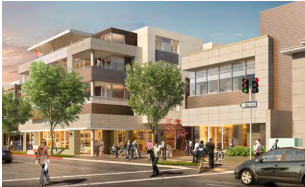
3225 El Camino Real: a mixed-use development with two distinct buildings. The first building is four stories with ground floor retail and apartments/condos on the upper floors. The second building is two stories with ground floor retail and office on the upper floor. The development includes underground and podium parking.
