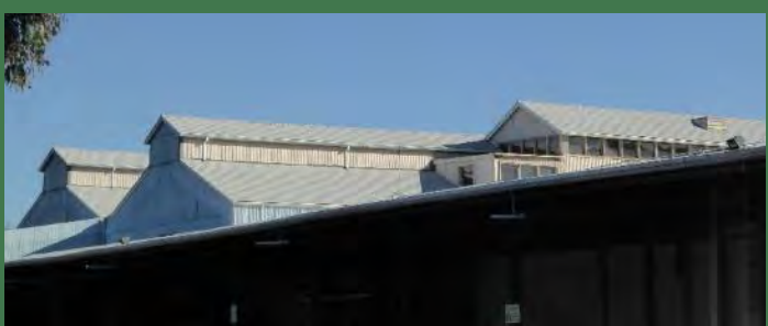
Figure 12 Gabled addition attached to the southernmost monitor roof of 340 Portage Avenue. View northeast. Source: Page & Turnbull
