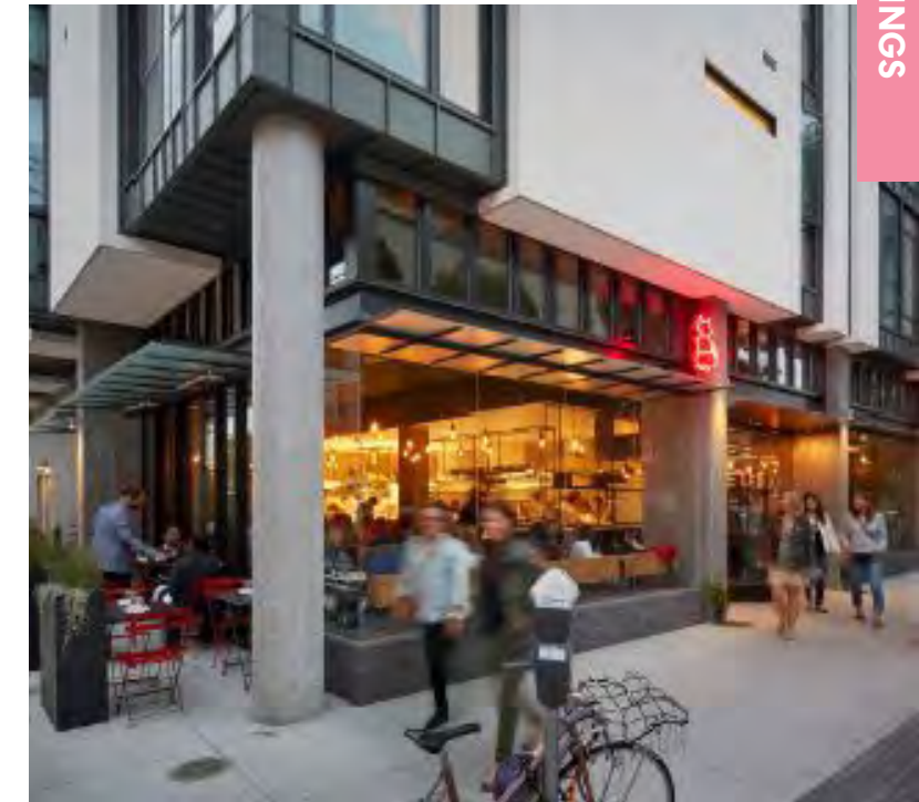
Figure 84 Ground floors can create notches of outdoor rooms to allow for lively spillover of retail.
