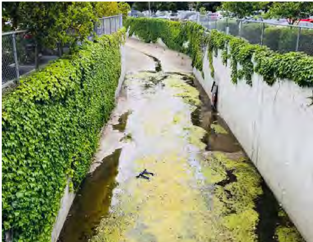
Figure 79 The Matadero Creek Channel is currently a constrained concrete trapezoidal channel.
