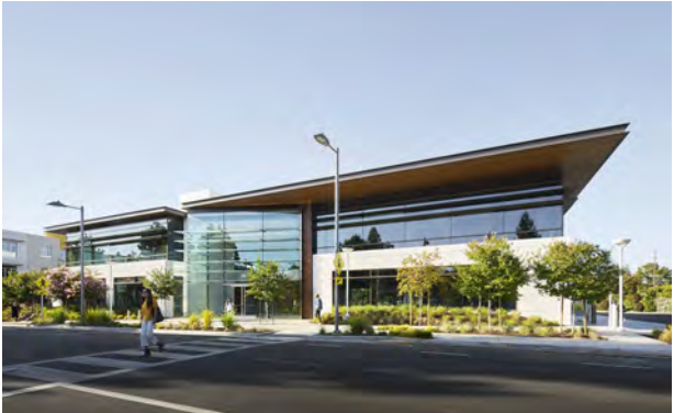
3045 Park Boulevard: a two-story shell commercial building with underground parking.
