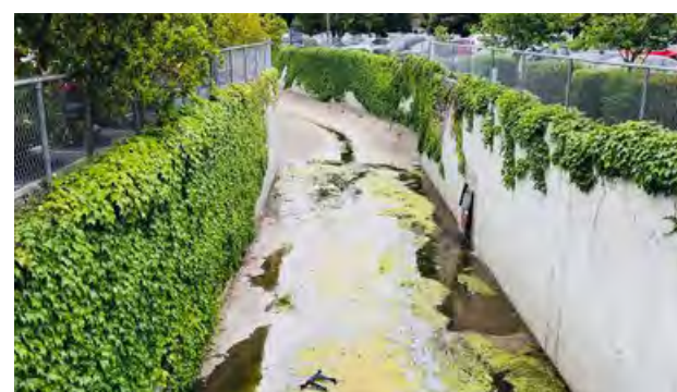
Figure 5 The Matadero Creek Channel is currently a constrained concrete trapezoidal channel.
