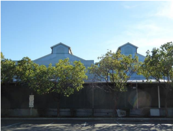
Figure 53. A planting bed with small deciduous trees along the cement loading platform at the rear façade of the building. View southeast.
