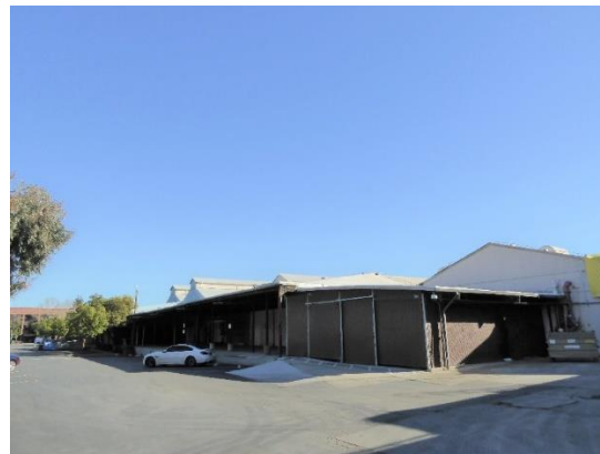
Figure 22. Middle section of the northwest façade. View northeast.
