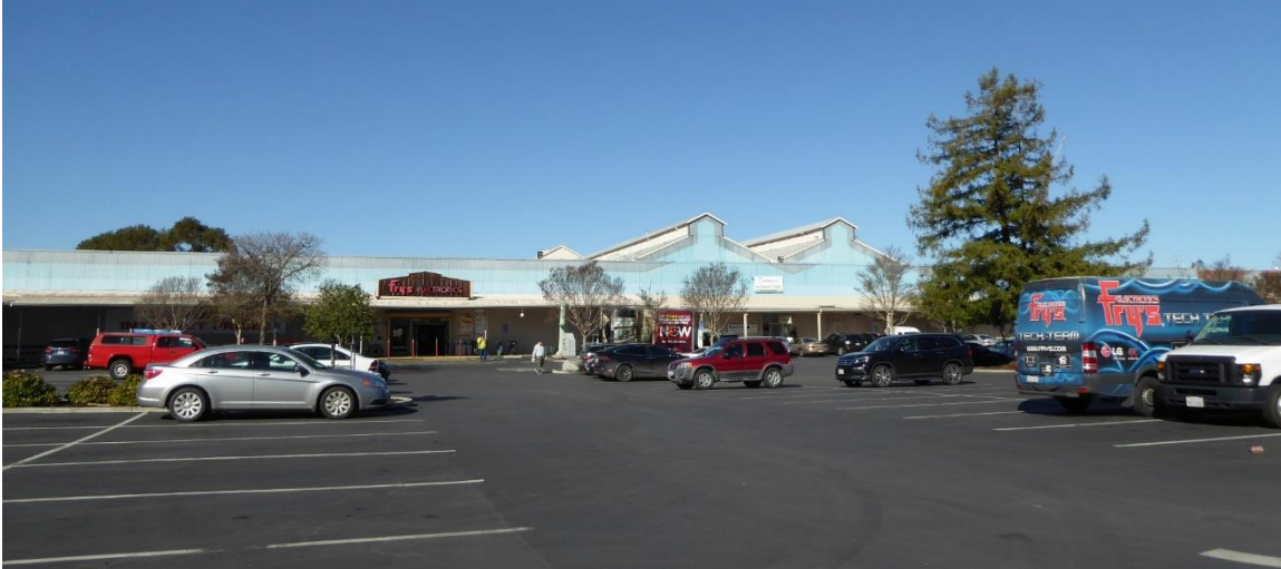
Figure 4: 340 Portage Avenue. View northwest from the parking lot located southeast of the building.
