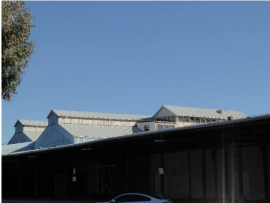
Figure 25. Gabled addition attached to the southernmost monitor roof of 340 Portage Avenue. View northeast.
