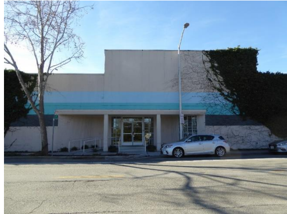
Figure 18. Recessed entry. View southwest.
