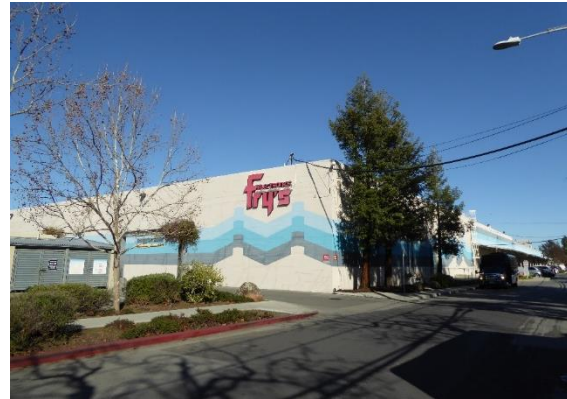
Figure 36. Southwest façade with lighted sign for Fry's Electronics. View north.
