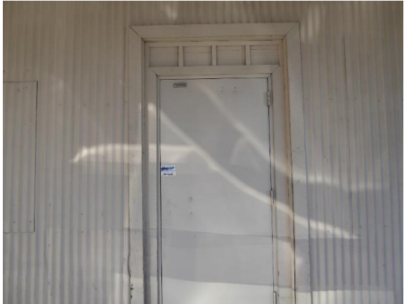
Figure 13. A metal door with blind transom and wood trim. View northwest.
