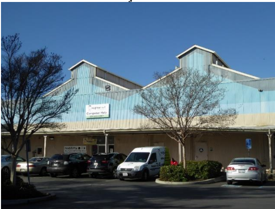
Figure 9. A pair of monitor roofs dominate the middle section of the southeast façade. View southwest.
