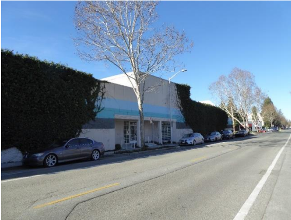
Figure 17. Northeast façade. View west.
