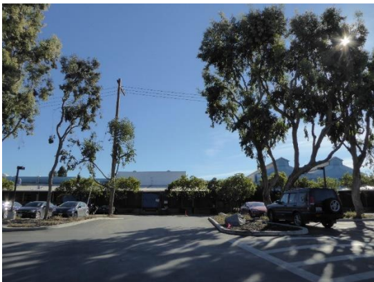
Figure 21. Middle section of the northwest façade. View southeast.
