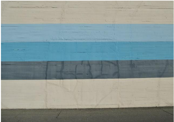
Figure 35. Repaired cracks on the southwest façade. View northeast.
