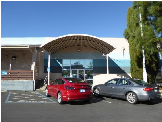
Figure 15. An arched metal awning over an altered entry at the far north end of the southeast façade. View northwest.
