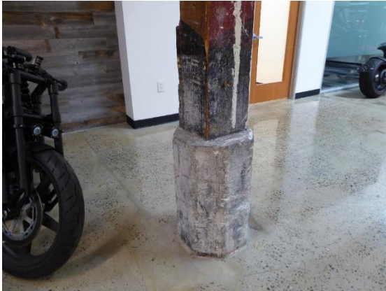
Figure 43. Original wood and concrete posts and concrete floors in 380 Portage Avenue.
