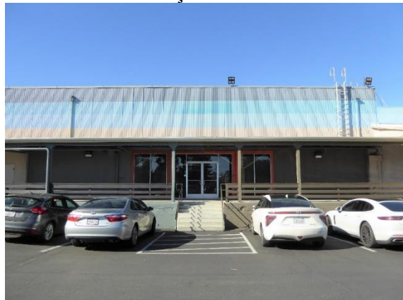
Figure 10. Concrete steps permit access to entries located on the concrete platform. View northwest.
