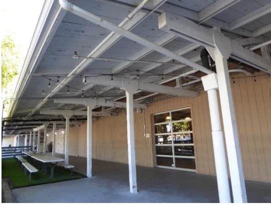
Figure 23. The loading platform or cooling porch converted into a patio with replacement aluminum frame garage door window. View northeast.
