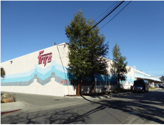
Figure 5. Southeast façade. View north.
