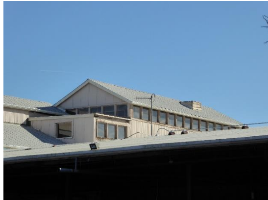
Figure 26. Close-up of the gabled and flat-roofed additions. View northeast.
