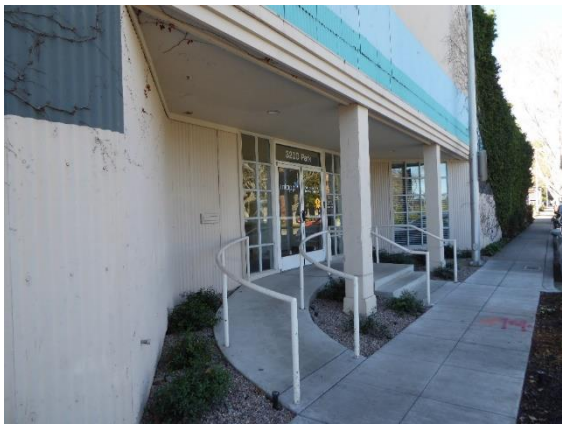
Figure 19. Curved, recessed entry with concrete ramp and steps, and aluminum frame glass doors and windows. View west.
