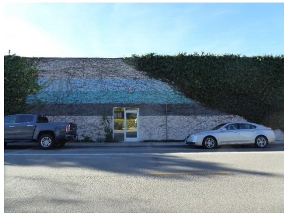
Figure 20. The second entry on the northeast façade. View southwest.
