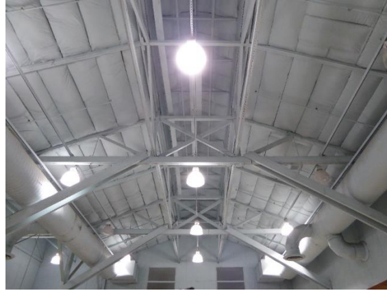
Figure 38. Exposed wood of a monitor roof, visible in 340 Portage Avenue.
