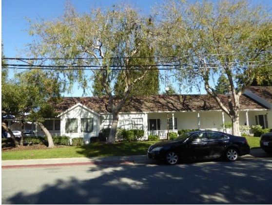
Figure 57. A portion of the southwest façade of the former office building. View northeast.
