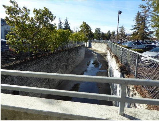
Figure 47. Matadero Creek borders the southwest parking lot. View south.
