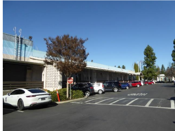
Figure 14. The north end of the southeast façade. Breezeblocks have been added beneath the awning in some locations. View north.
