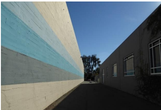
Figure 33. Southwest façade. View southeast.
