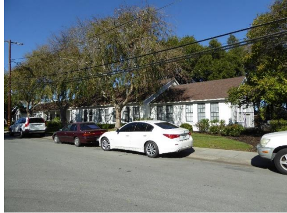
Figure 58. The rear portion of the southwest façade of the former office building. View northwest.
