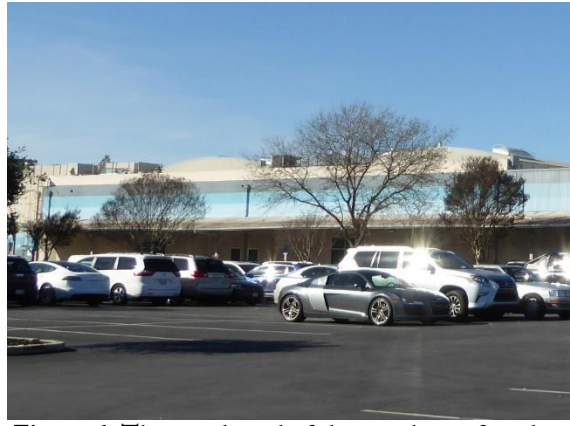
Figure 6. The south end of the southeast façade features two arched roofs. View southwest.
