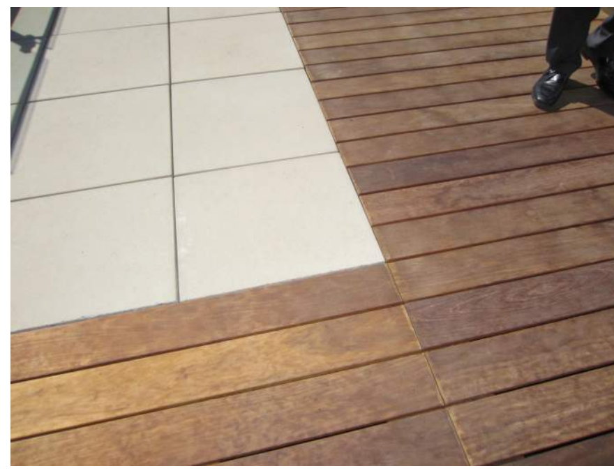
ACCENT PAVERS & WOOD DECKING ON PEDESTALS
