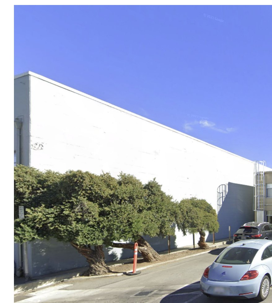
D WEST ELEVATION- VIEW FROM REAR PARKING LOT
