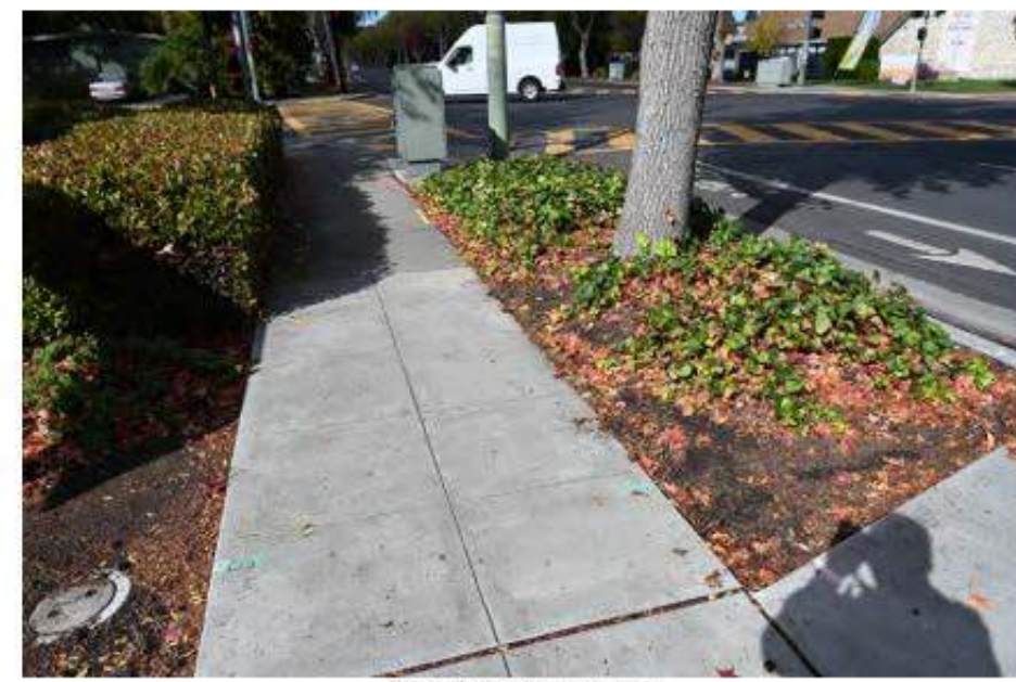
Sidewalk repair near tree #2.
