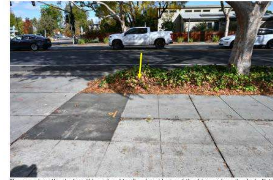
The area where the planter will be reduced to allow for widening of the driveway (see site plan). Note sidewalk repair that likely removed roots causing displacement.
