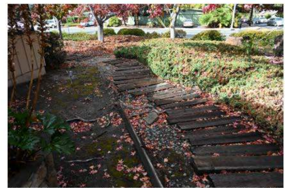
Surface roots extend 30 feet from the base of the tree. This area will be excavated for the new building foundation.
