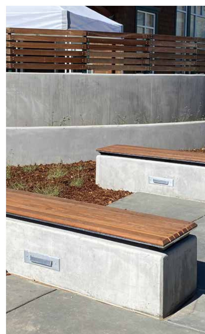
Cast in place seatwall with wood bench topper
