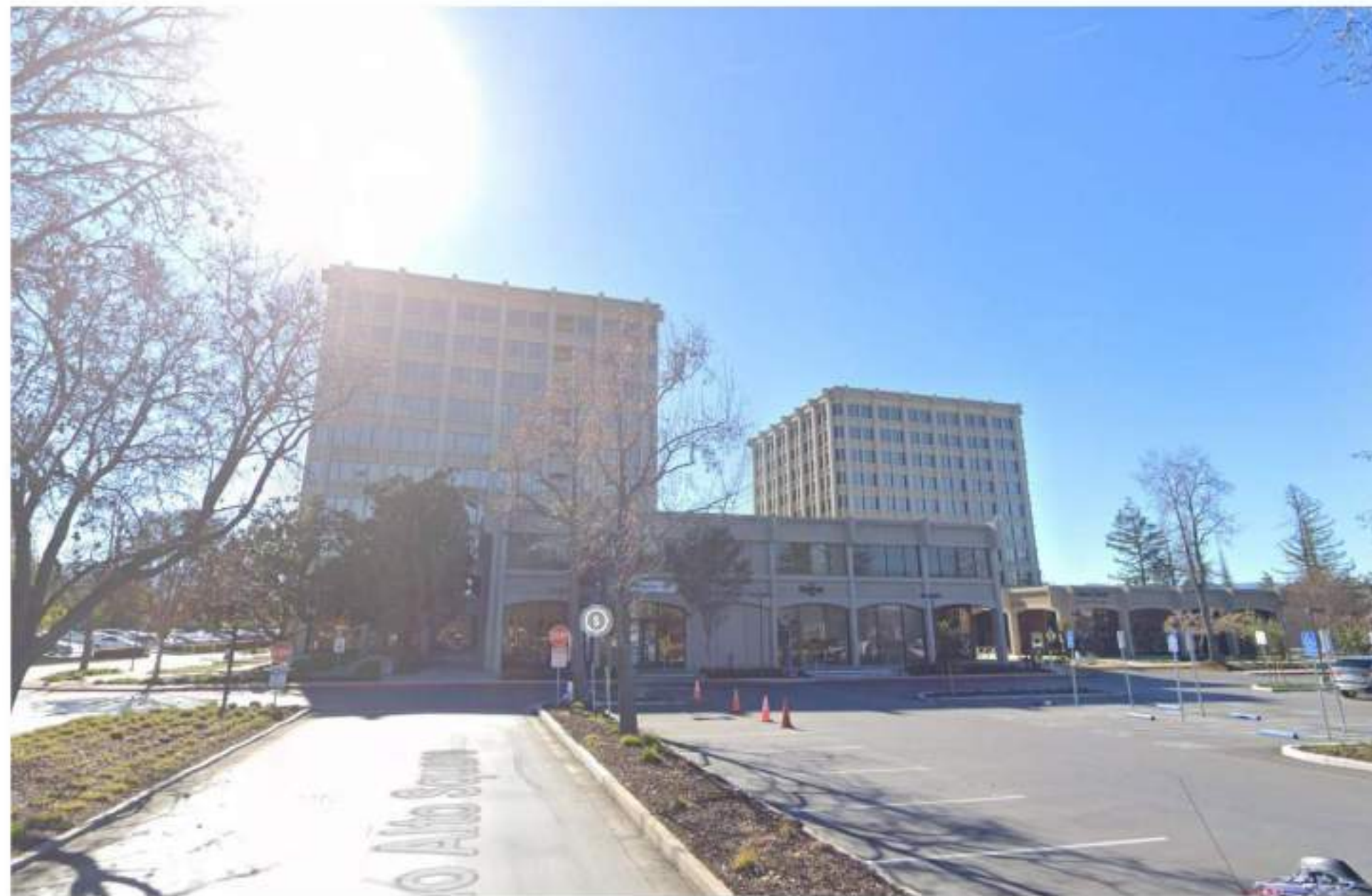
1. OFFICE BUILDING FACING ECR
