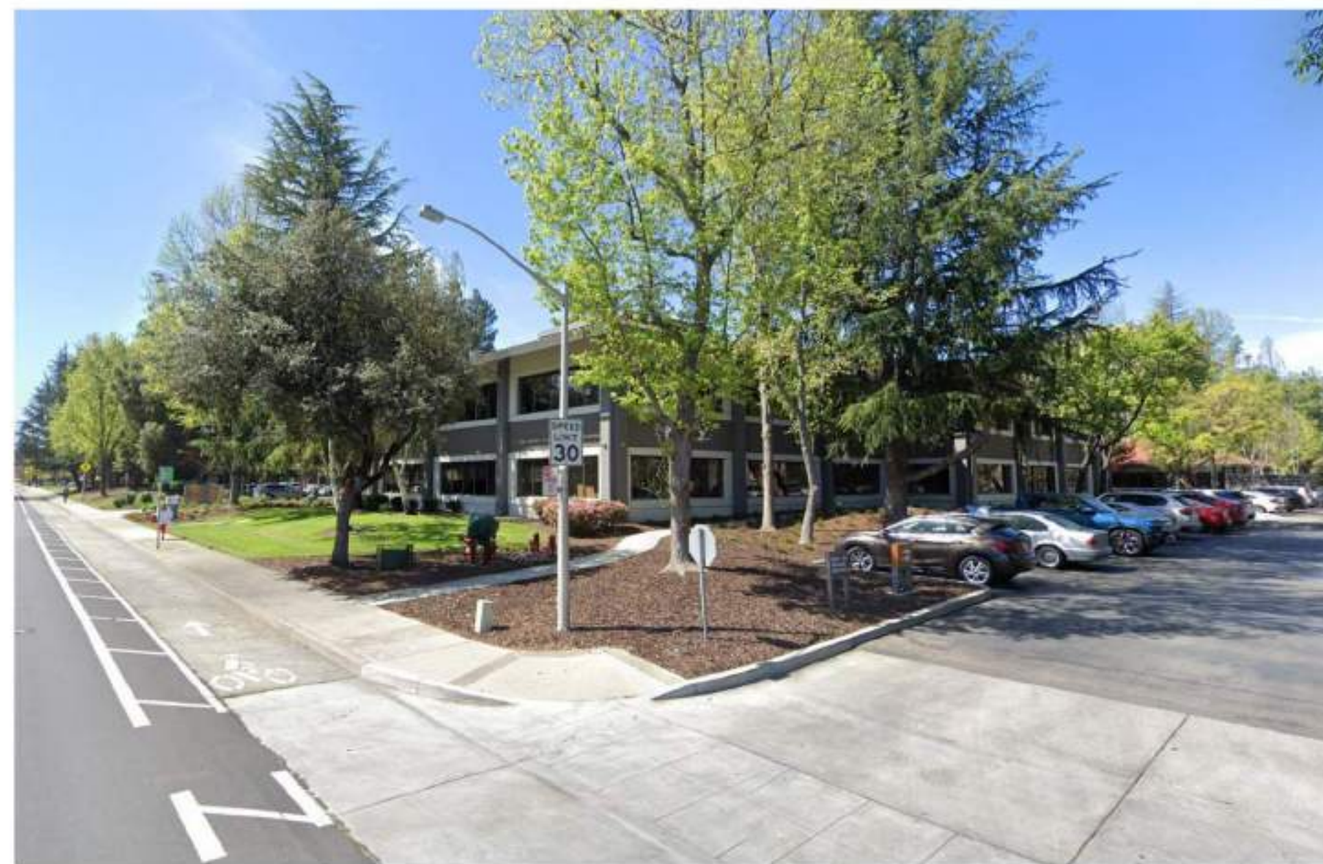
7. ADJACENT OFFICE BUILDING ON HANSEN WAY
