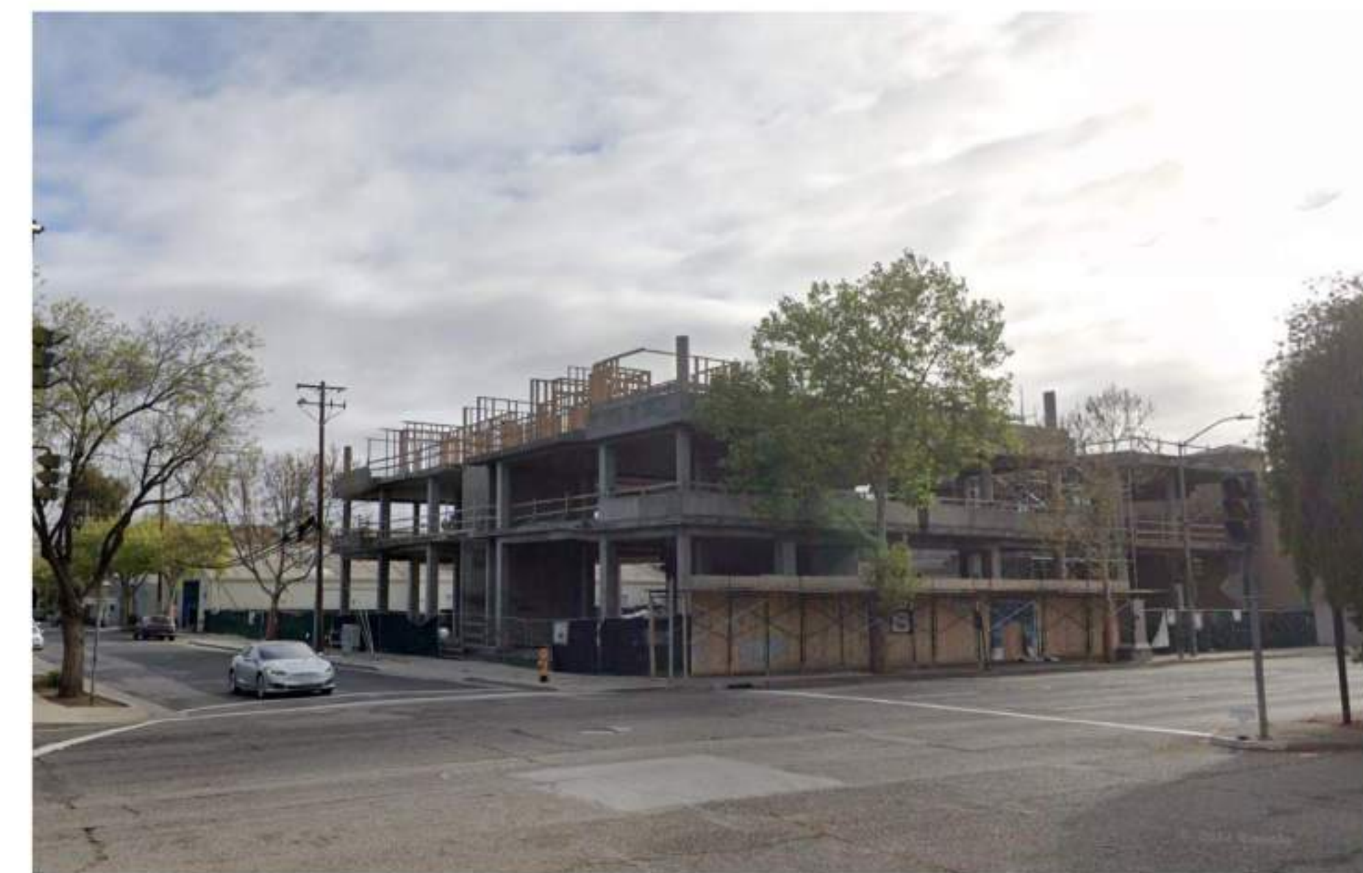
4. 5-STORY OFFICE BUILDING ACROSS ECR
