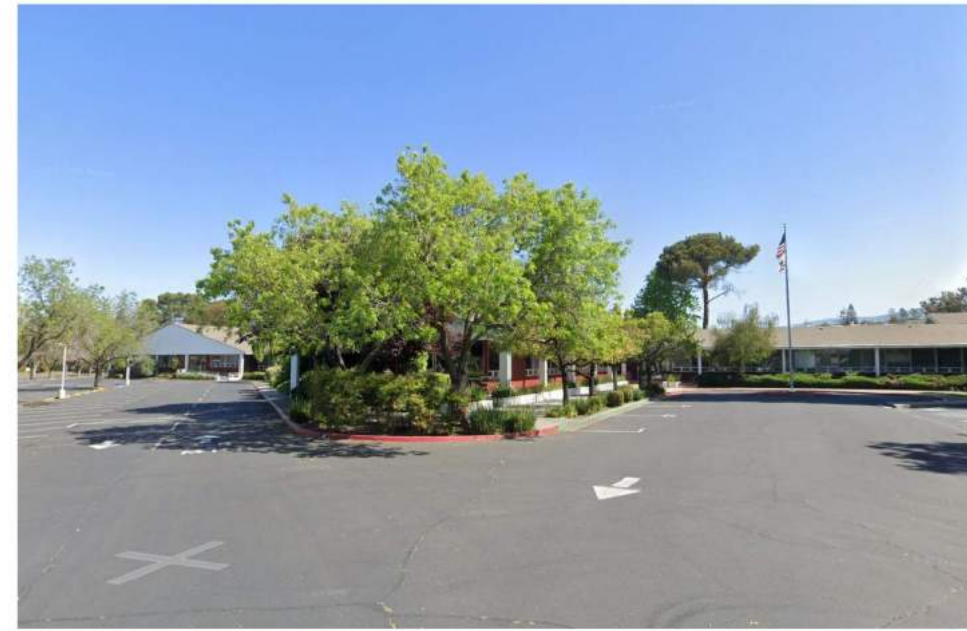
6. OFFICE BUILDING ACROSS HANSEN WAY
