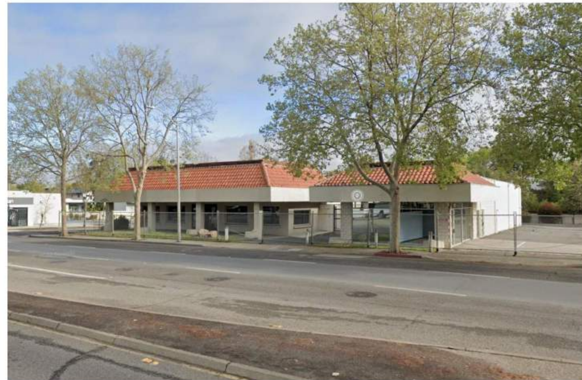
2. OFFICE BUILDING FACING ECR
