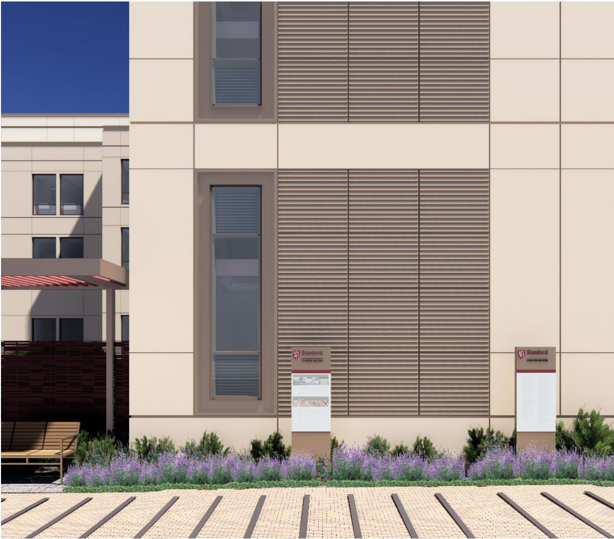
Building Close Up - Horizontal Rib Option (1" WX 3/8" D)
