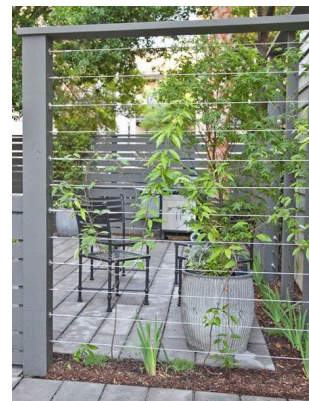
Vertical screen with tensioned ss cables
