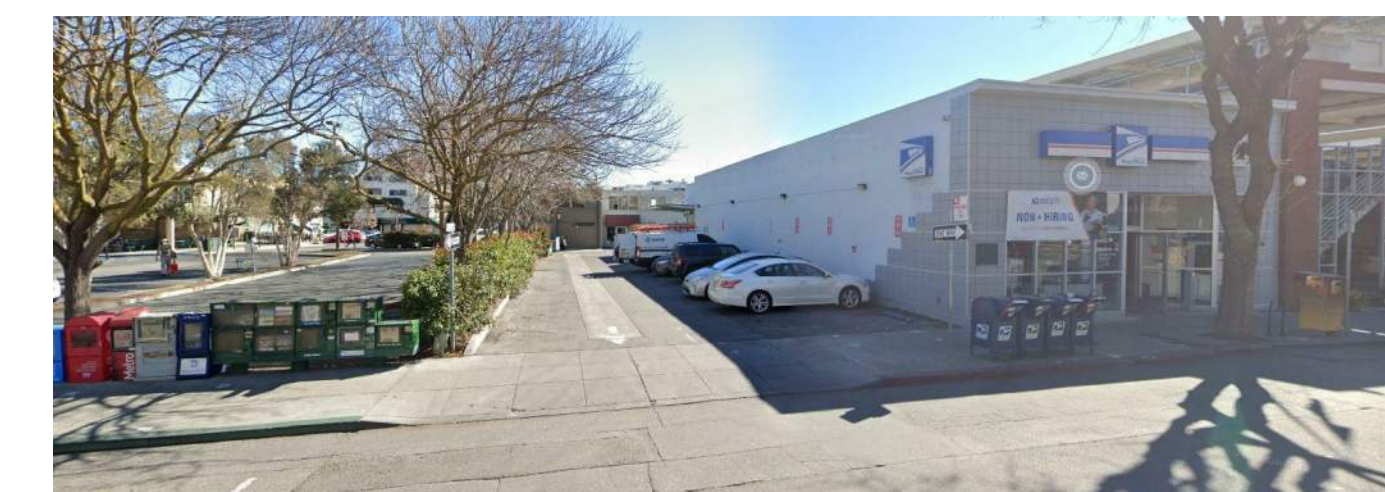
8) VIEW FROM CAMBRIDGE AVENUE LOOKING AT SERVICE ALLEY ADJACENT TO LOT "A"
