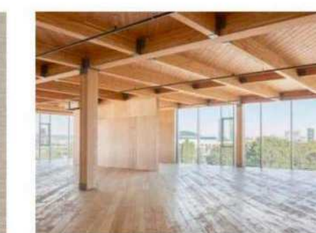
MASS TIMBER CONSTRUCTION
