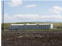
Figure 2: 2023 Reconnaissance Survey photograph.
