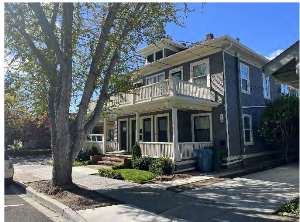
Figure 2: 2023 Reconnaissance Survey photograph.
