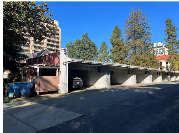
Figure 2: 2023 Reconnaissance Survey photograph.
