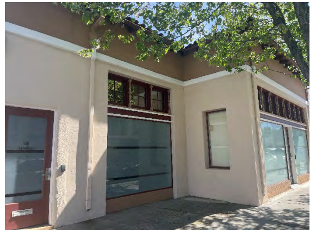
Figure 2: 2023 Reconnaissance Survey photograph.
