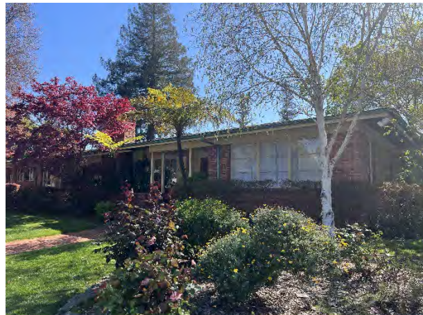
Figure 2: 2023 Reconnaissance Survey photograph.
