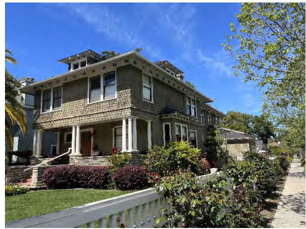
Figure 2: 2023 Reconnaissance Survey photograph.
