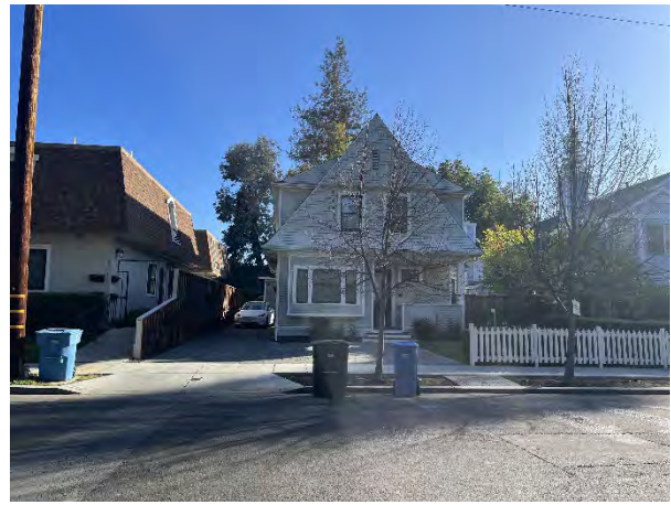
Figure 2: 2023 Reconnaissance Survey photograph.
