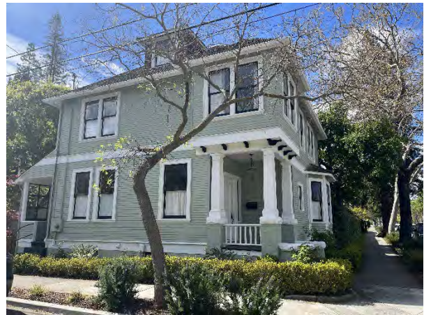
Figure 2: 2023 Reconnaissance Survey photograph.
