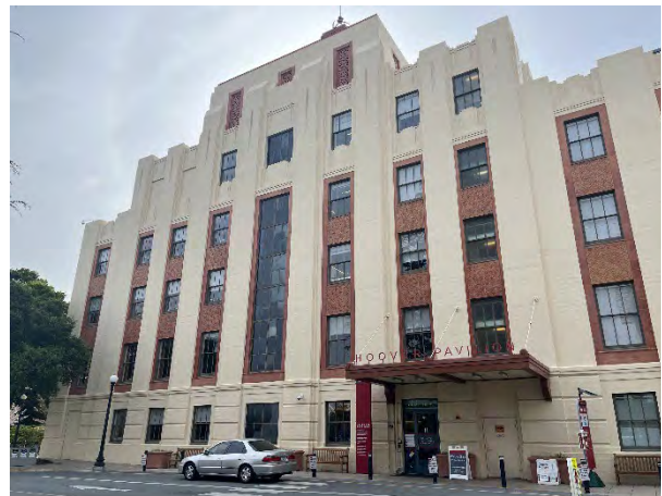
Figure 2: 2023 Reconnaissance Survey photograph.
