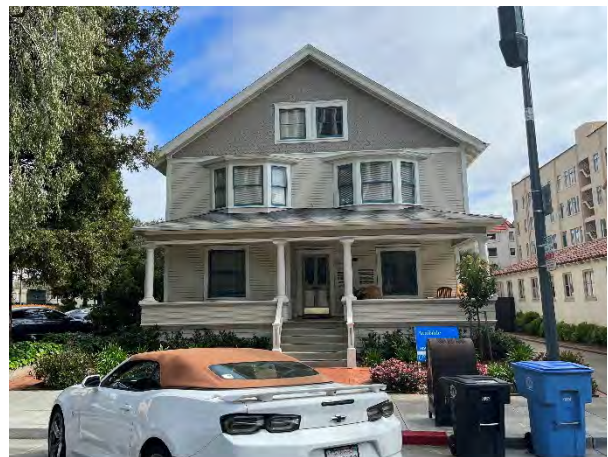
Figure 2: 2023 Reconnaissance Survey photograph.
