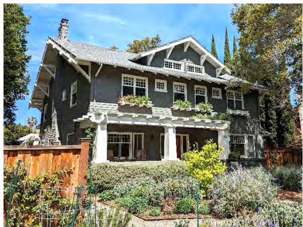
Figure 2: 2023 Reconnaissance Survey photograph.
