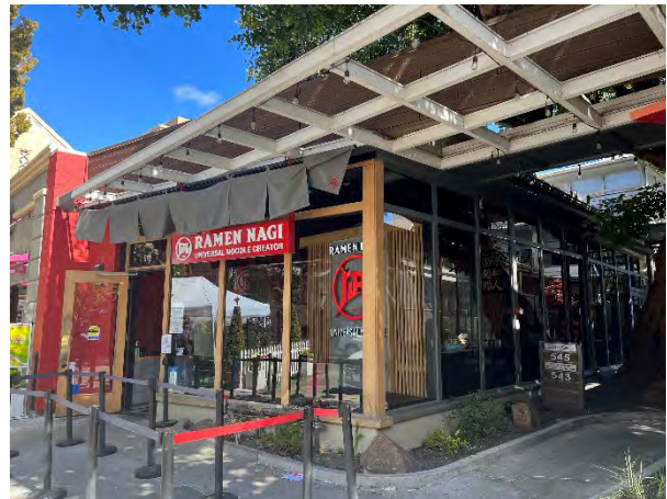
Figure 2: 2023 Reconnaissance Survey photograph.
