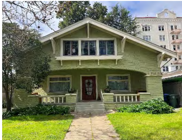
Figure 2: 2023 Reconnaissance Survey photograph.
