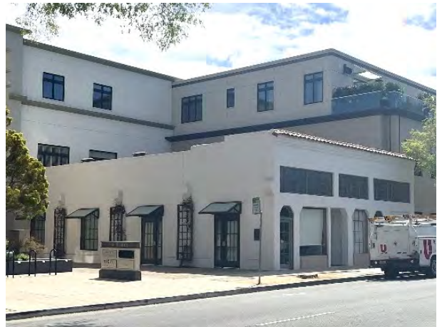
Figure 2: 2023 Reconnaissance Survey photograph.
