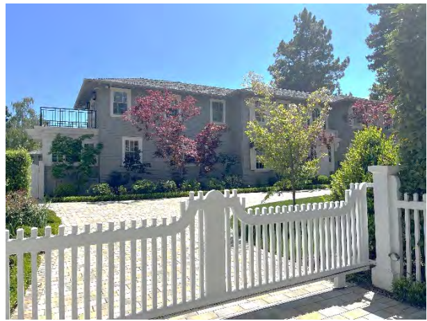
Figure 2: 2023 Reconnaissance Survey photograph.
