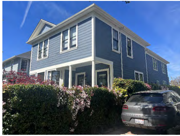
Figure 2: 2023 Reconnaissance Survey photograph.
