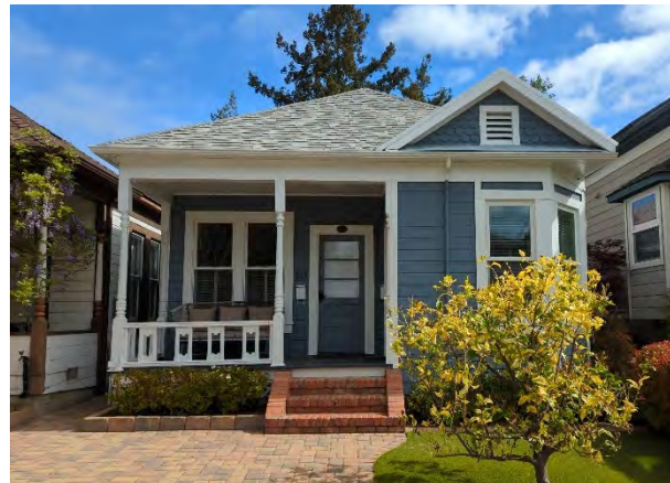
Figure 2: 2023 Reconnaissance Survey photograph.
