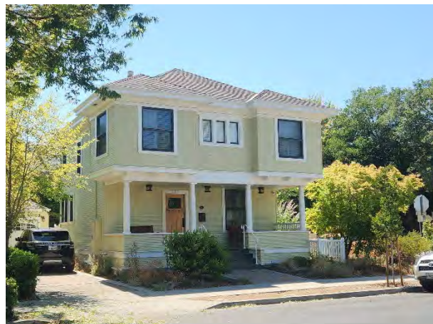
Figure 2: 2023 Reconnaissance Survey photograph.
