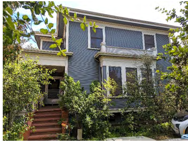
Figure 2: 2023 Reconnaissance Survey photograph.
