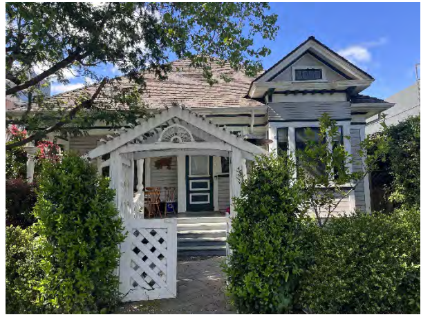
Figure 2: 2023 Reconnaissance Survey photograph.
