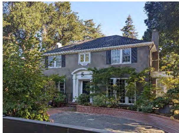
Figure 2: 2023 Reconnaissance Survey photograph.
