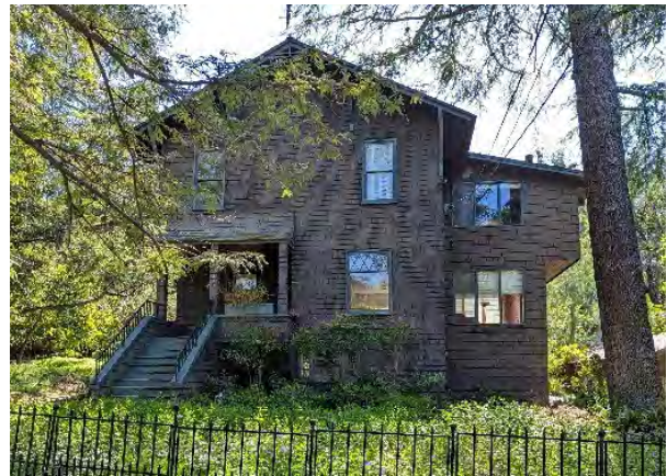
Figure 2: 2023 Reconnaissance Survey photograph.
