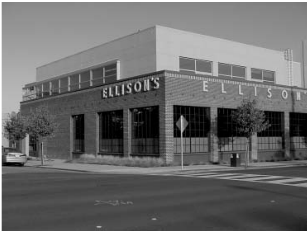
Renovated Businesses on Alma Street
