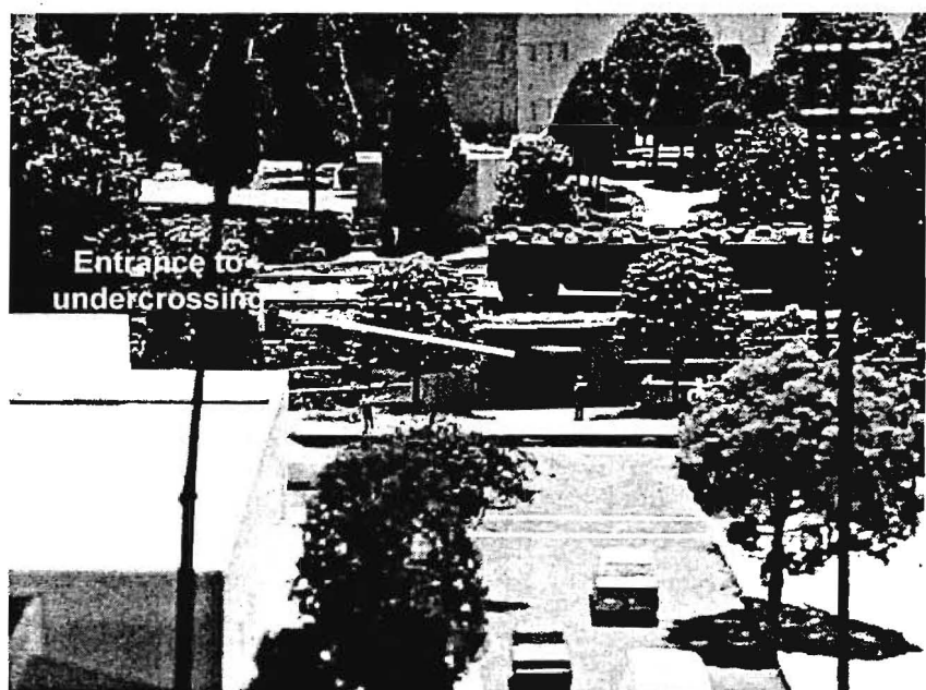
View to the west from Homer Avenue toward the new PAMF campus
