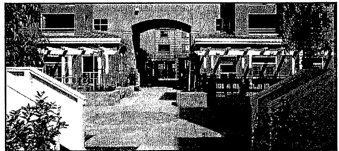
GUIDELINE 3.3.10. The top of the podium slab should be landscaped to mask the slab's artificial character. Here, the podium is designed to provide important community open space.
