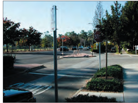
Figure 4.14: El Camino and Frontage Road at Miramonte Avenue.
