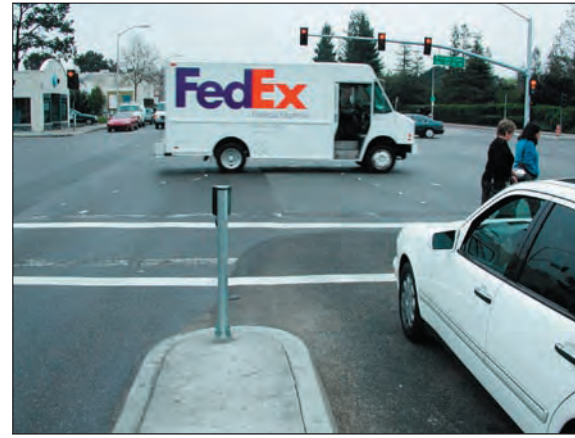
Figure 4.43: Medians like the one here at Page Mill Road do not provide a safe place for waiting pedestrians.
