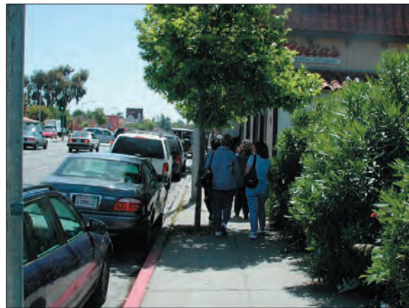
Figure 4.33: 8-foot Sidewalks constrict pedestrian circulation and access.
