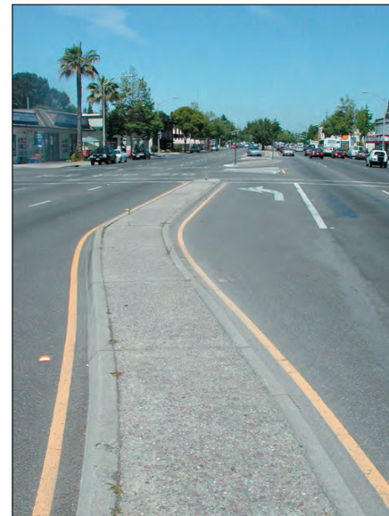
Figure 1.11: Cut-through traffic from El Camino is a concern for some neighborhoods.
