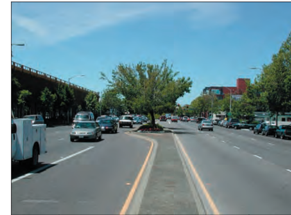
Figure 2.3: Narrow median on El Camino today.
