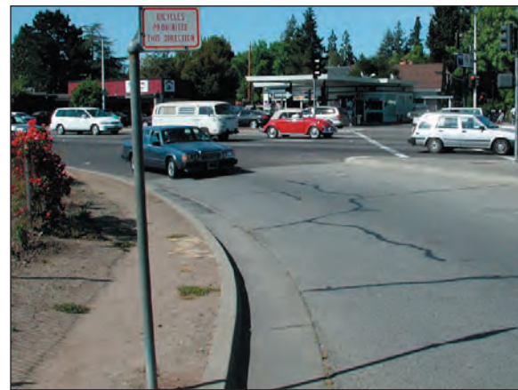
Figure 5.41: Free right turns and “pork chop” islands complicate pedestrian circulation at intersections.
