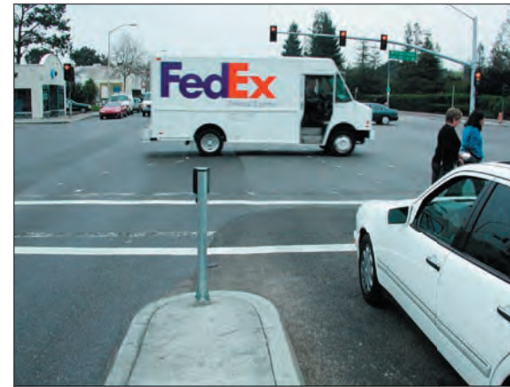
Figure 1.2: Pedestrian accommodation at medians is minimal.
