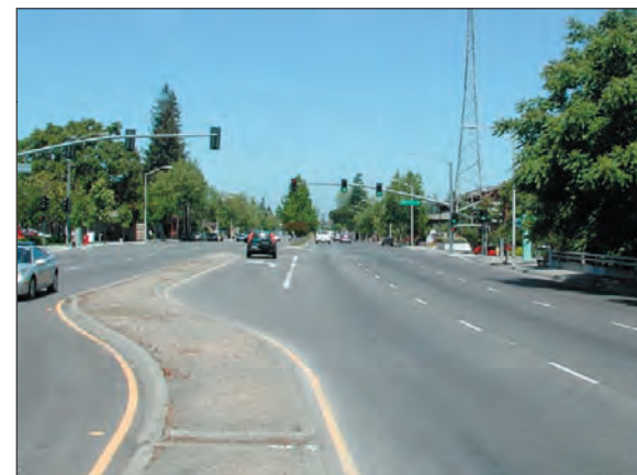
Figure 4.16: El Camino Adobe Creek (looking north).
