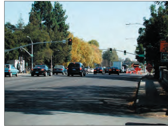
Figure 4.15: El camino at San Francisquito Creek (looking south).
