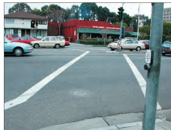
Figure 4.40: Crosswalks on El Camino have an average length of 104 feet. The distance increases where crosswalks are not perpendicular to the roadway.
