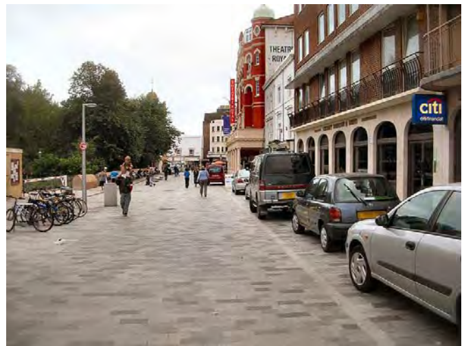
Shared streets are usually distinguished by the removal or lowering of curbs, positioning of parking stalls, street trees and other furnishing elements, lack of pavement markings, and special surface treatments.
