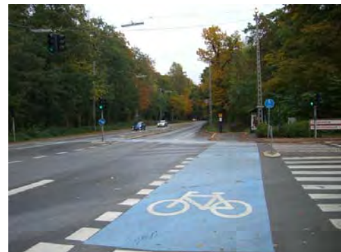
Crossbikes are commonly used in Europe to separate pedestrian and bicycle crossings of major streets.
