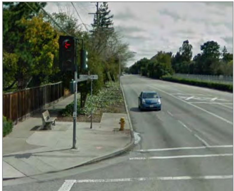
Alma Street between the Mountain View border and El Dorado Avenue is tentatively planned for repaving in 2012. Future paving and bicycle/pedestrian priorities should be coordinated as far in advance as possible to maximize design and funding opportunities for new and improved facilities. (Image from Google Streetview)
