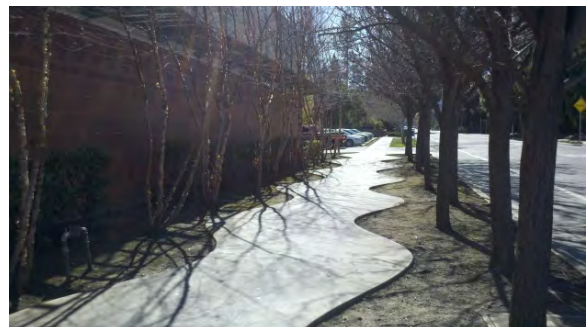
Although artistic sidewalk designs are encouraged, weaving or irregularly patterned edges should be avoided due to their difficult navigation by persons with disabilities and approved wheeled devices.
