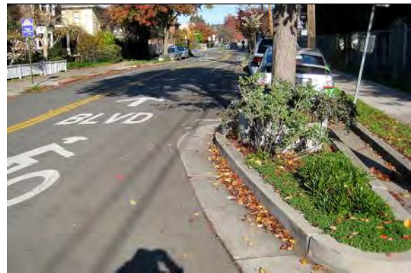
The City of Berkeley has installed a chicane along a bicycle boulevard that minimizes drainage costs by leaving a gap by the sidewalk.
