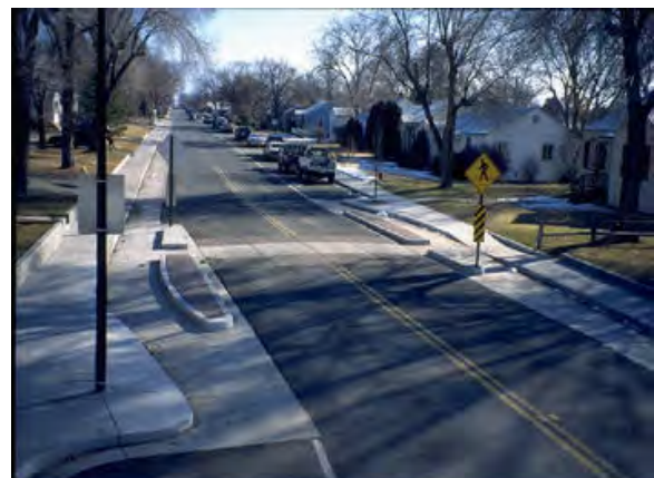
This choker shortens a mid-block crosswalk and provides a channel for bicyclists and drainage.
