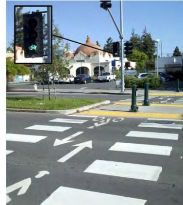
A bicycle signal is paired with a wider crosswalk to accommodate bicyclists in Berkeley, CA to assist with the Ohlone Greenway crossing of University Avenue.
