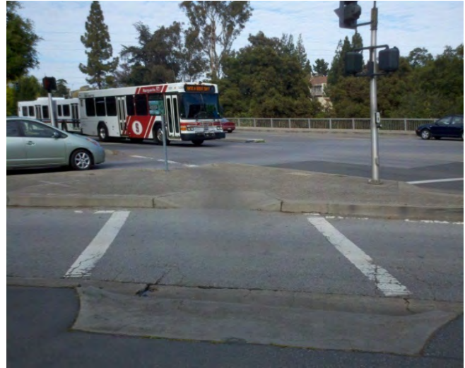
The series of non-conforming curb ramps and isolated islands across Palm Drive and the El Camino Real off ramps makes walking or biking to downtown or the transit center much less inviting.
