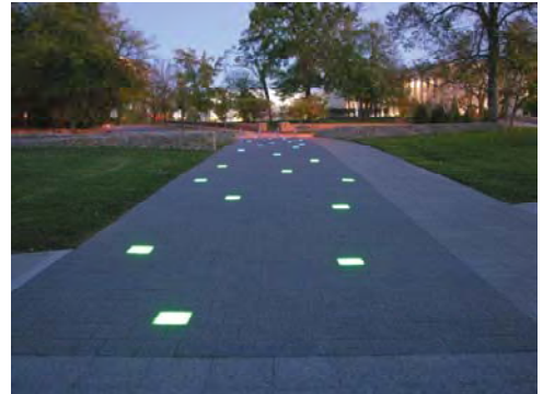
Inlaid lighting at the Kansas City Art Institute (source: Bowman Bowman Novic, Inc.)
