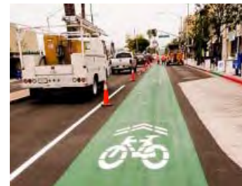
This sharrow in Long Beach, CA uses an underlying green color treatment to help improve visibility and alert motorists
