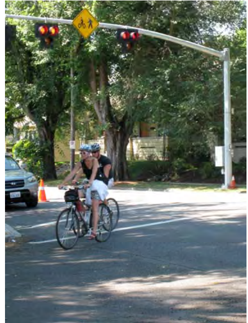
HAWK signal in Portland, OR assists with an arterial crossing on a bicycle boulevard. Note the use of the combined pedestrian/bicycle warning sign (W11-15).
