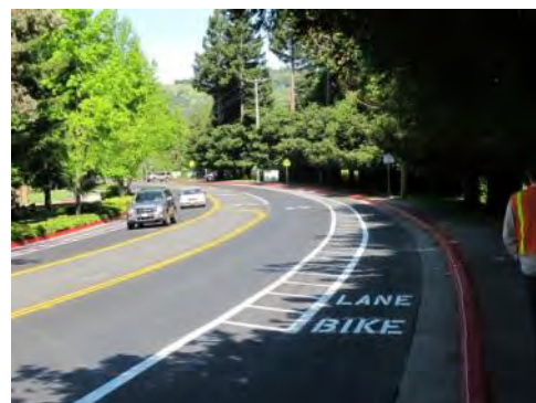
Fairfax, CA: Buffered bike lanes installed as part of a Safe Routes to School project on Sir Francis Drake Blvd (arterial).
