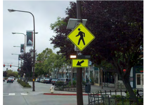
RRFBs can be solar powered and are an inexpensive alternative to full signalization. Note: City of Palo Alto standards call for a circular, as opposed to a rectangular, beacon signal head.
