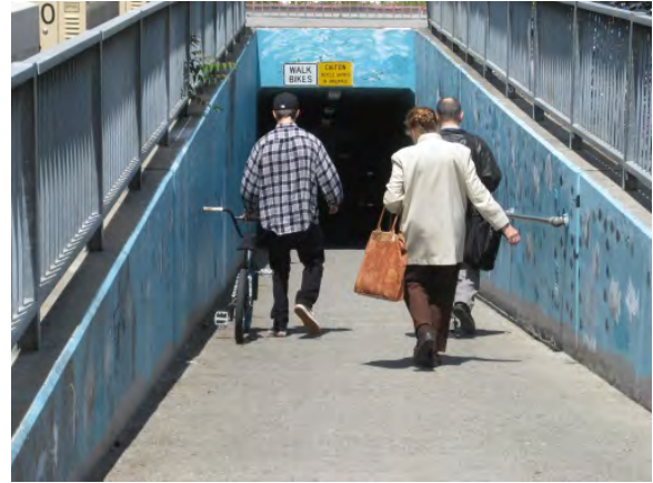
The California Avenue undercrossing is frequently used, but it is narrow and challenging for pedestrians with disabilities.
