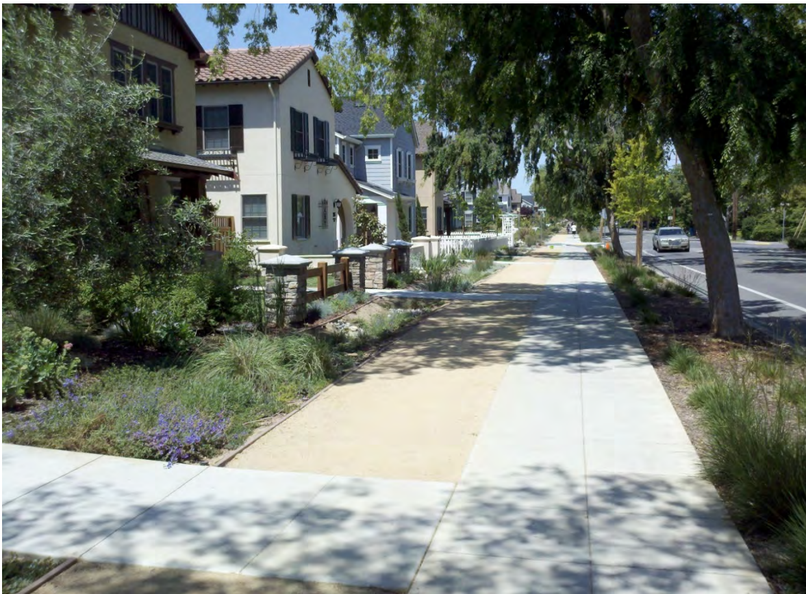
The new sidewalk constructed along Stanford Avenue adjacent to a faculty housing development includes both a paved and unpaved surface to support utilitarian and recreational (jogging) pedestrian activity. This hybrid walkway extends from Hanover Street to El Camino Real along the Bay to Ridge Trail.
