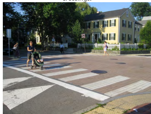
Raised intersections also calm traffic, but can be expensive due to drainage issues.
