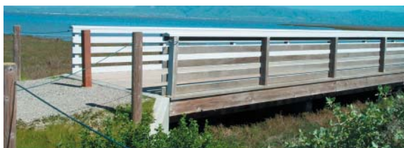
Sailing Station Pier: interior of fence is painted white, exterior is unpainted. Note how the unpainted side blends with the natural environment while the white painted side stands out.
