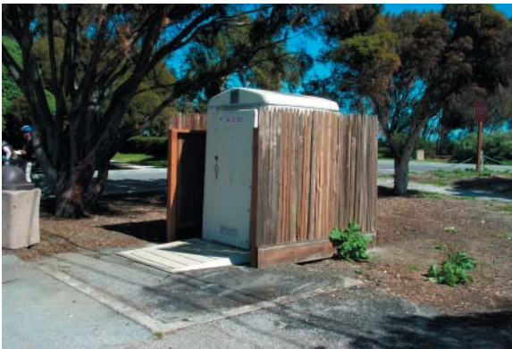
Insufficient enclosure at Duck Pond parking lot. Wood stakes are not tall enough to fully screen portable rest room. The design, material selection and construction detailing appear improvisational and of marginal quality.
