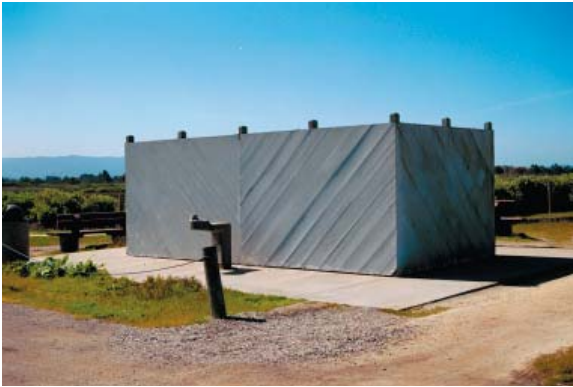
Acceptable bathroom enclosure at Sailing Station parking lot. Wood has been stained or painted gray to fit in with landscape.
