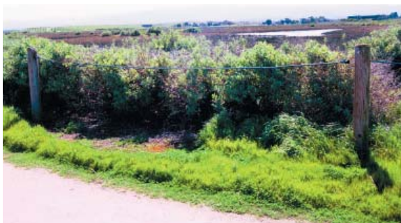
Bollard from 8" peeler core and plastic-coated cable
