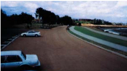
NaturalPave, an alternative resin pavement installed at the Harbor Point Parking Lot is being evaluated.
