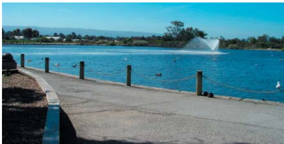
Bollards from re-used utility poles and galvanized chain
