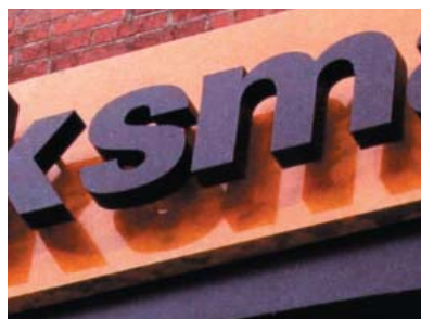
Individually formed letters, raised attachment
