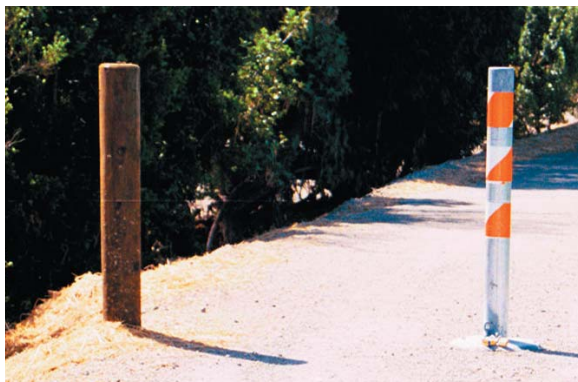
Here two kinds of bollards are used– the removable bollard has orange and white reflective tape. White tape alone would probably be sufficient for safety and less visually jarring.
