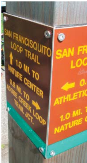
Haphazard installation of Directional Sign adds to visual clutter.
