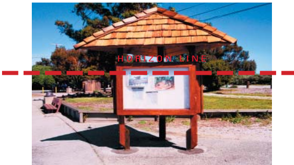
Duck Pond Kiosk, with its bright colors and isolated placement, appears awkward. Its roof punctures the horizon line.
