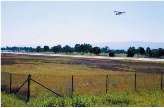
Airport: black vinyl-coated chain link fence— no top rail.
