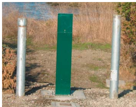
Here metal bollards and a steel enclosure are of different colors. One muted color for all the elements would be better.
