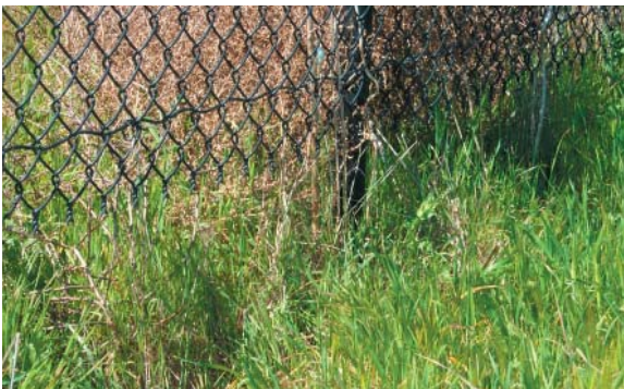
Airport: 4" gap allows wildlife to slip under the fence
