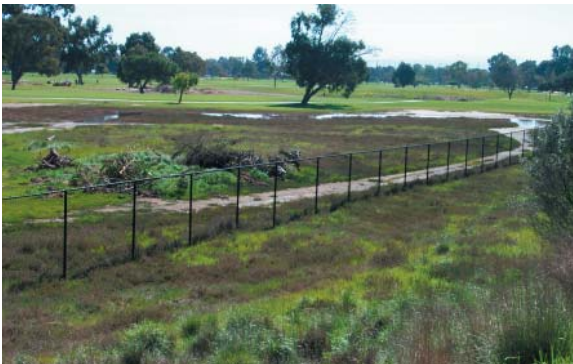
Golf Course: black vinyl-coated chain link fence— with top rail.
