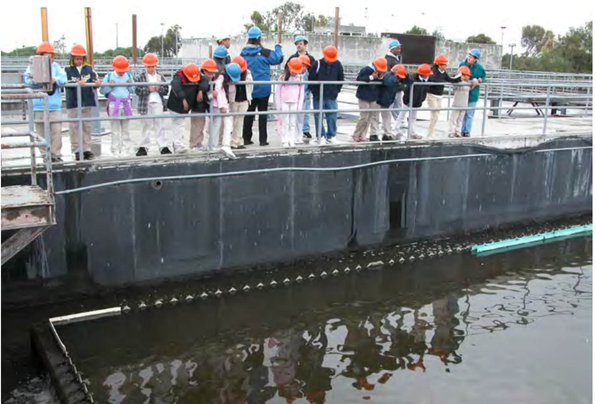
The Regional Water Quality Control Plant has been designed to remove most of the organic pollutants found in wastewater. The plant consistently removes 99 percent of these organic and solid pollutants which has gone a long way to restoring the health of the South Bay. Shown above is a school tour of the waste-water clarifiers. Also see "Thank you" letter from one of the tour participants in this chapter.
