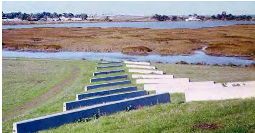
The Chevrons, made from highway barriers, reference the nearby Bayshore Freeway. They also align with the airport runway and from the air, create an aeronautical symbol meaning "don't land here."
