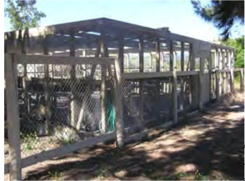
Native plant nursery—built with Save The Bay volunteers in 2004 to propagate plants for marsh and riparian habitat restoration.
