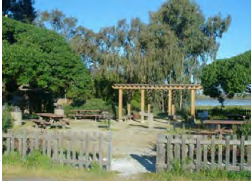
New picnic area—built in 1991—near the Harbor Master’s Cottage in the Palo Alto Baylands
