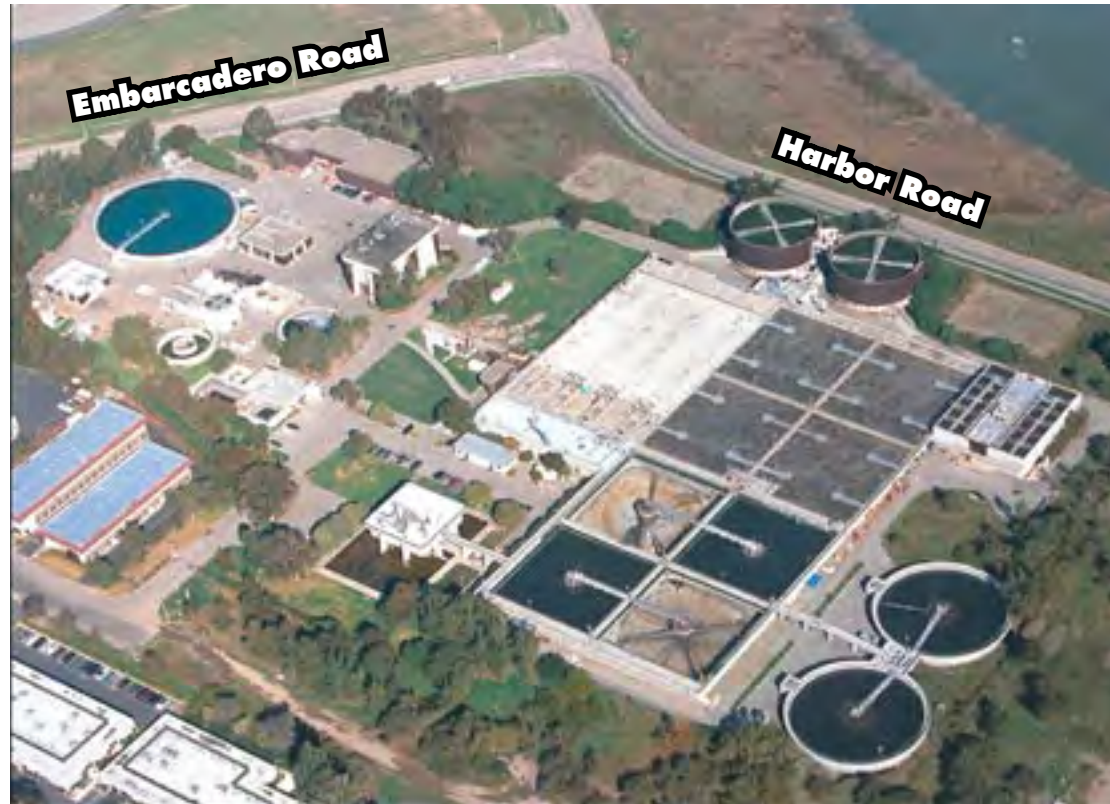
1999 aerial photo of the Palo Alto Regional Water Quality Control Plan (Also see photo of Palo Alto Sewage Treatment Plant taken around 1948 in the “Overall Environmental Quality” chapter.)
