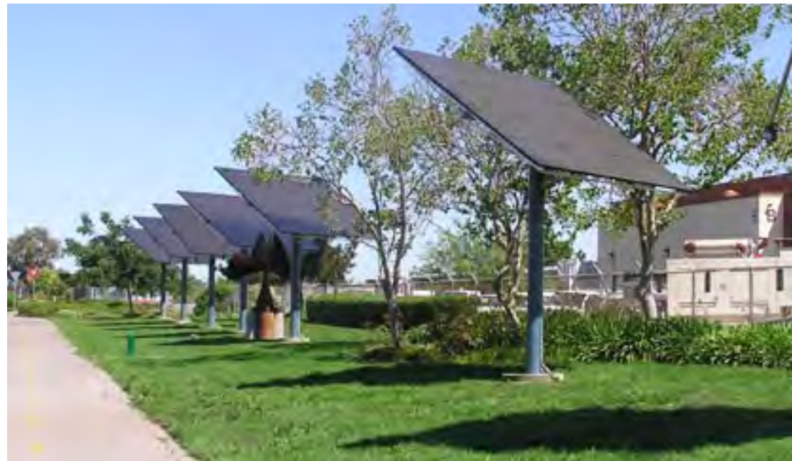
The photovoltaic panels installed at along the frontage road at the MSC are “trackers”. They pivot to follow the sun—maximizing the amount of electricity they can produce each day.
