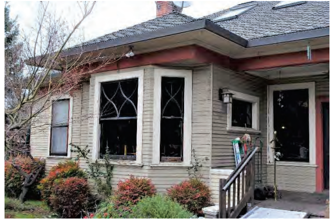
Figure 2: Primary (southwest) façade entrance, looking north.
