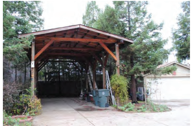
Figure 10: Detached, double-height carport, looking northwest.
