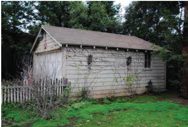
Figure 9: Detached garage, looking west.
