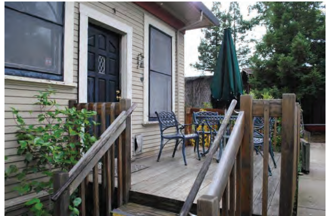
Figure 8: Wood deck on northwest façade, looking south.
