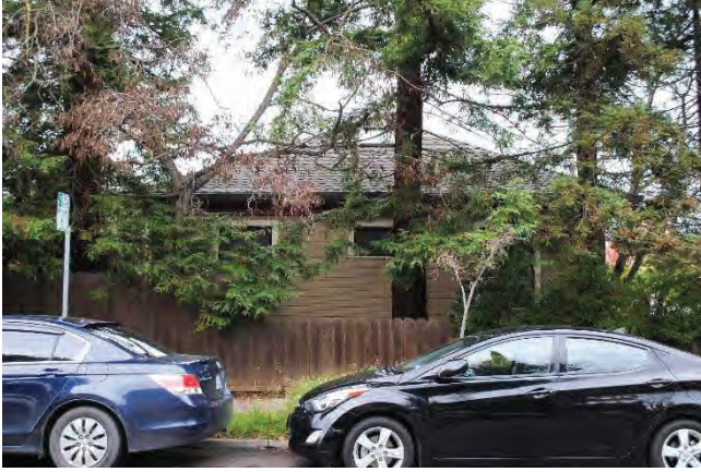
Figure 5: Southeast façade, looking northwest.
