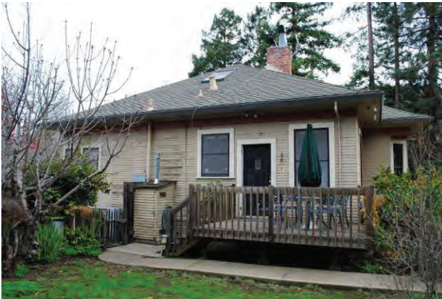
Figure 7: Northwest façade, looking southeast.
