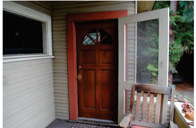
Figure 4: Secondary, replacement entry door, looking east.
