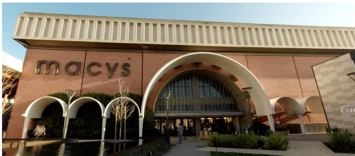
Existing Exterior Facing Façade (South West)
