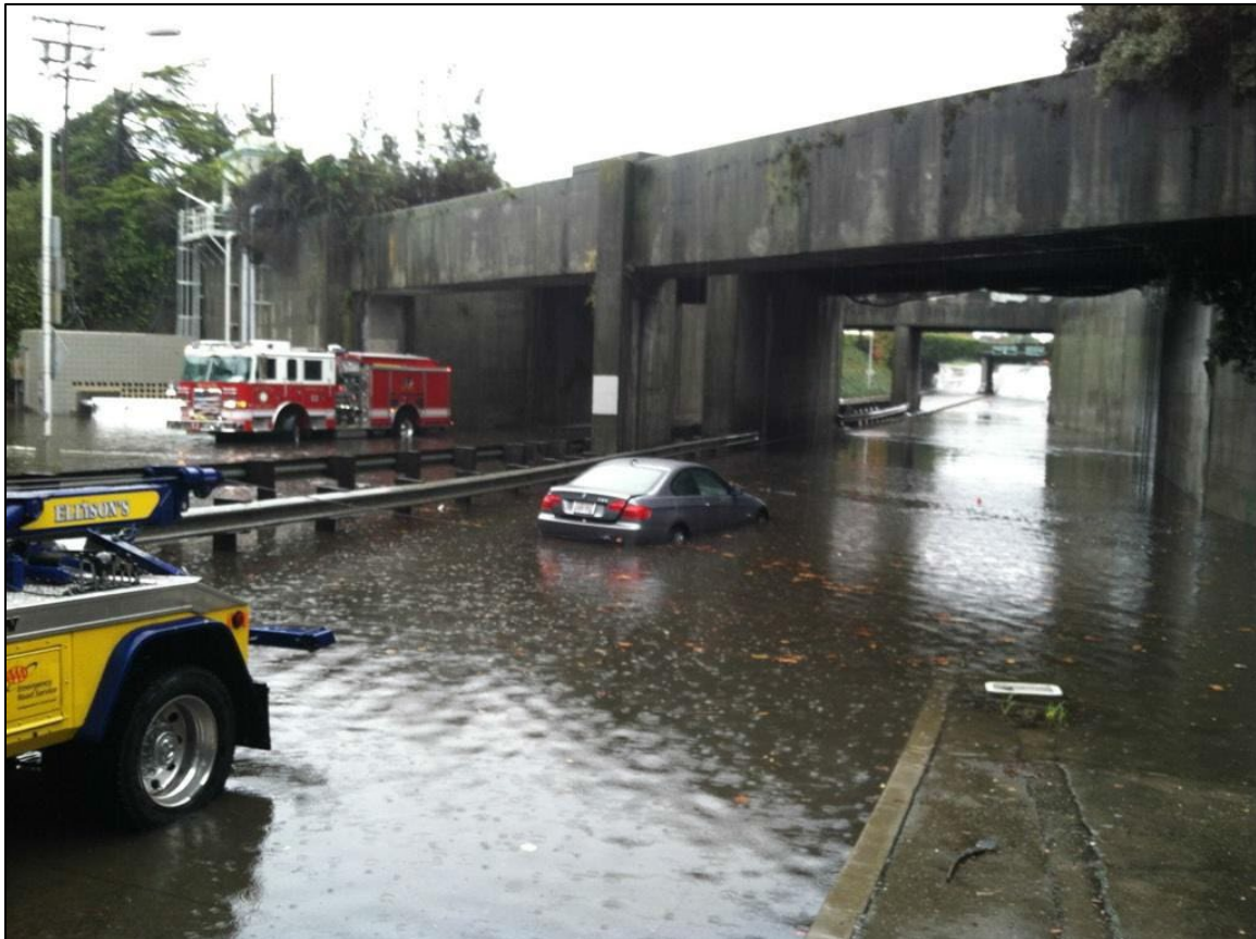
Figure 1: Photo: Dec. 2, 2012: Car Stuck in Flood under Oregon/Alma Underpass
