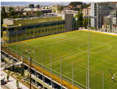
Underhill Parking Garage at UC Berkeley includes a full size soccer field built over a 1,000 space, four-level parking facility
