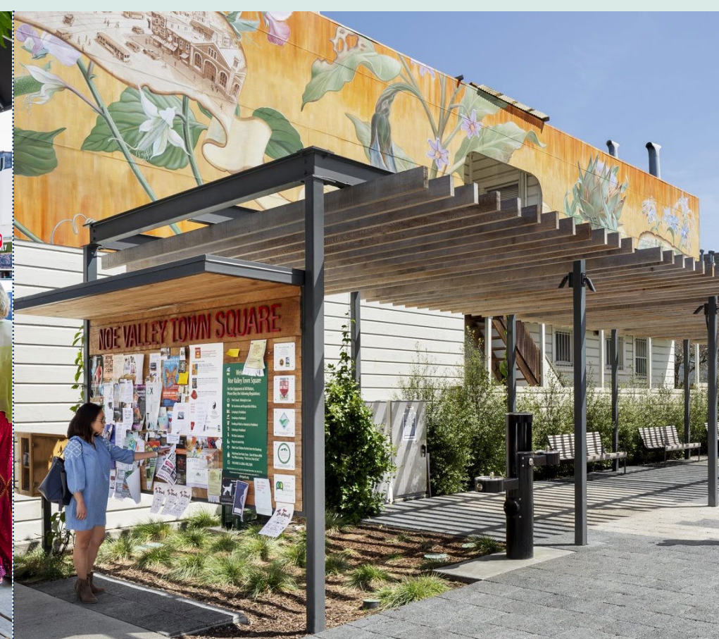
Custom fixed overhang with built-in community board
