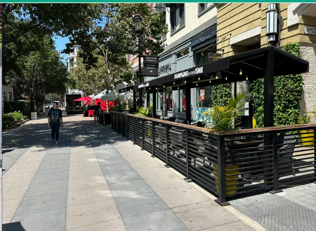
Bolted metal railings with overhang
