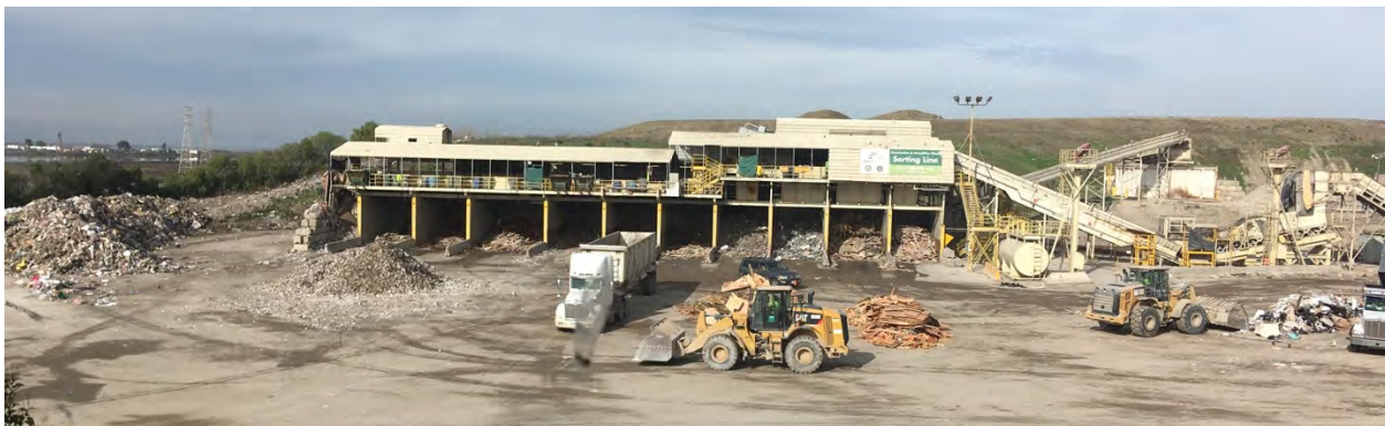
Zanker Materials Processing Facility
