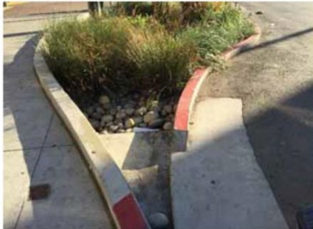
Figure 2-26. Effective curb radius for a street sweeper in SF. (Credit: EOA)
