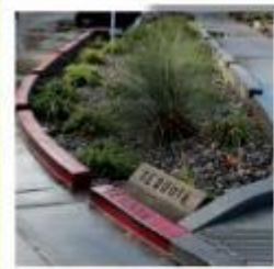
Engineered bioretention beds mimic nature by slowing, spreading, sinking and filtering storm water.
