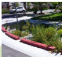
Bioretention area in a curb cut-out in the Southgate Neighborhood, Palo Alto
