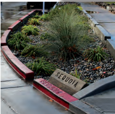
Engineered bioretention beds mimic nature by slowing, spreading, sinking and filtering storm water.
