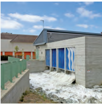
The San Francisquito Creek Storm Water Pump Station installed in 2009 clears storm water from streets in a 1,250 acre neighborhood in northeastern Palo Alto.
