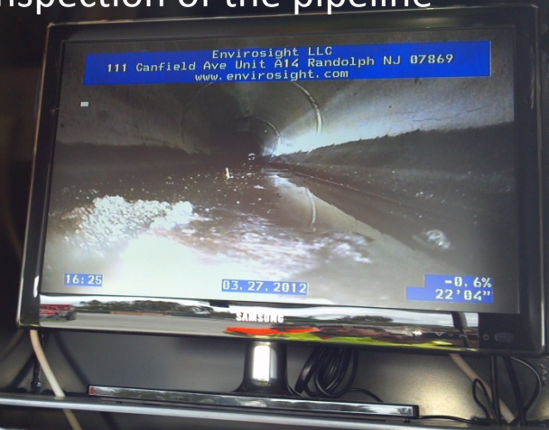
Camera inspection of the pipeline
