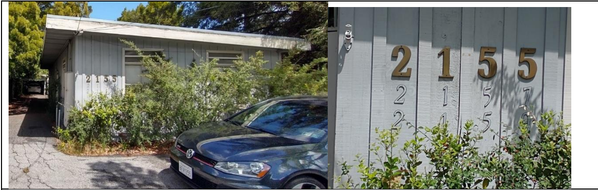
There are three existing units, not two.
