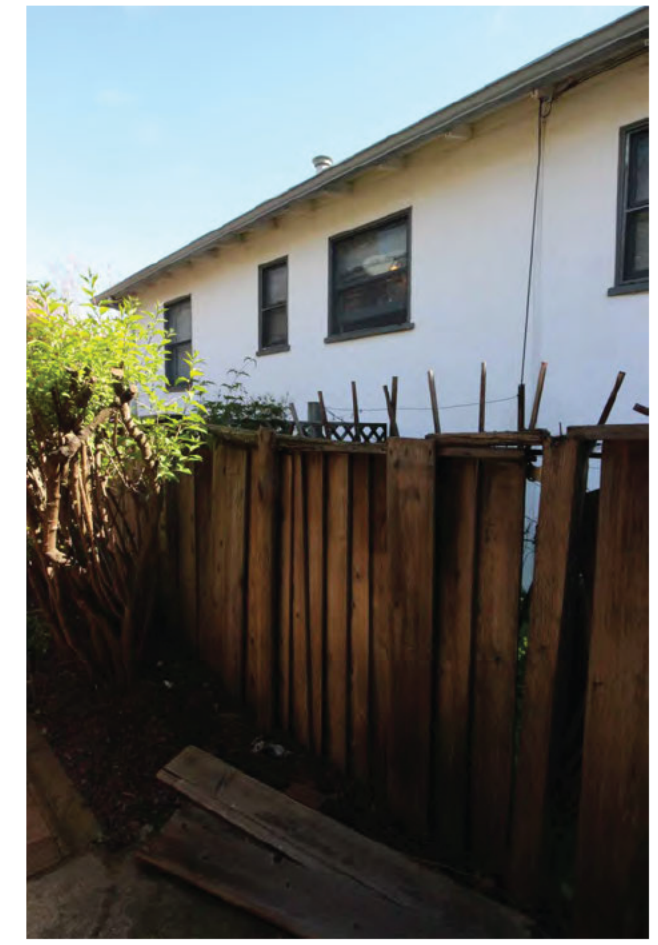
4 VIEW OF 991 CHANNING FROM EAST SIDE YARD
