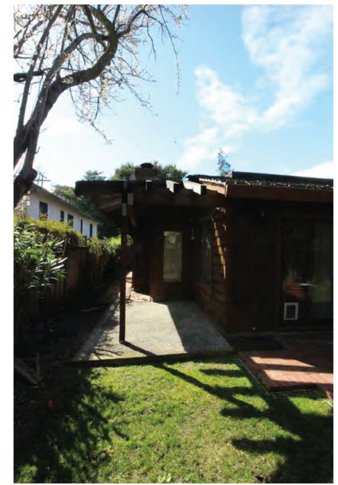
7 (E) PATIO AT AT NORTHEAST CORNER OF BUILDING
