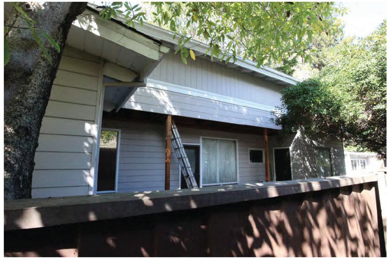
2 VIEW OF 975 CHANNING FROM WEST SIDE YARD
